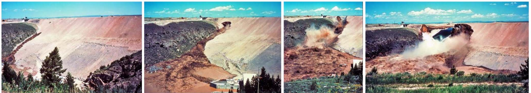
Breach of Teton Dam, June 5, 1976
