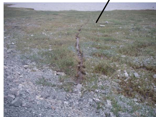
Example of unimpeded flow through pad.
