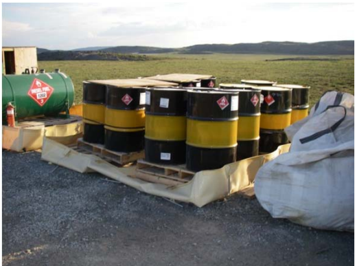
Secondary containment for jet fuel. Note compromised berm.
