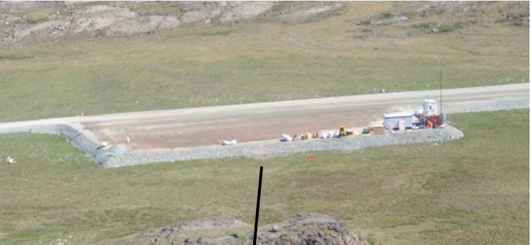
Oblique aerial of the north airstrip apron. Note air traffic control tower, emergency shelter and genset on right.
