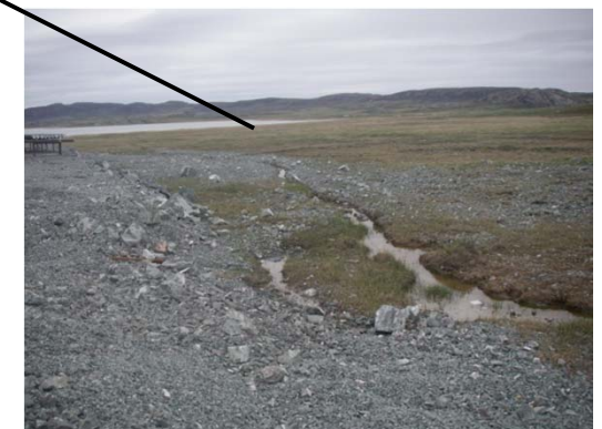
Example of unimpeded flow through pad.
