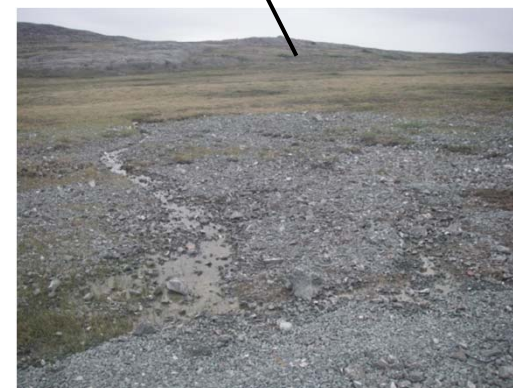
Example of unimpeded flow through pad.
