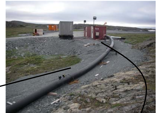
Doris Lake water intake pipeline and pump station.
