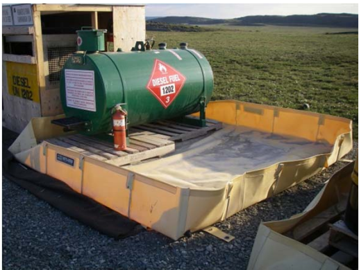
Secondary containment for fuel tank supplying the airstrip control tower generator. Note compromised berm.
