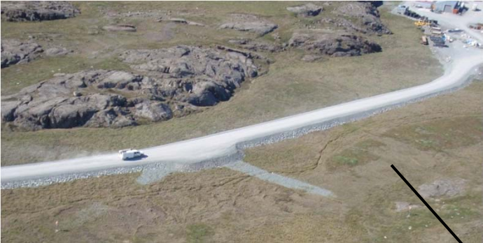
Typical example of all weather road turnout. The spurs leading from this turnout are to service runway lights.
