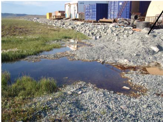
Ponded water at the toe of the pad.
