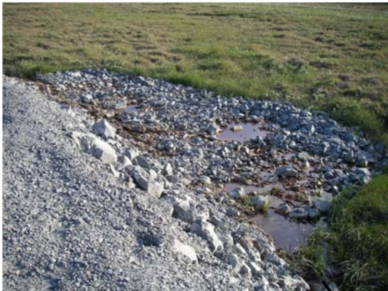
Ponding on west side of road north of road laydown area. Site of a road turnout that was removed.
