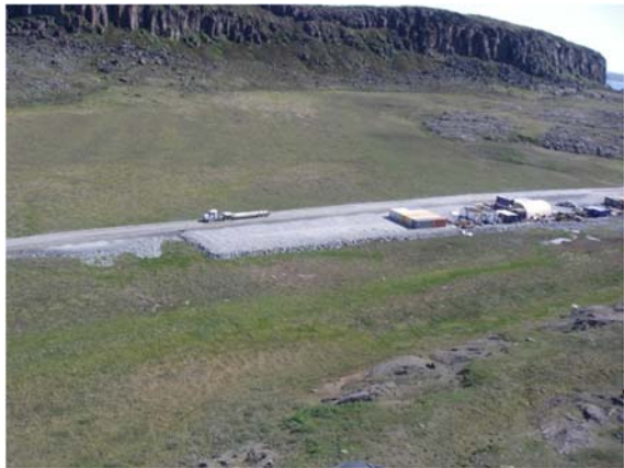
Oblique view looking south across road laydown area. Note rock pulled back of tundra adjacent to turnout.
