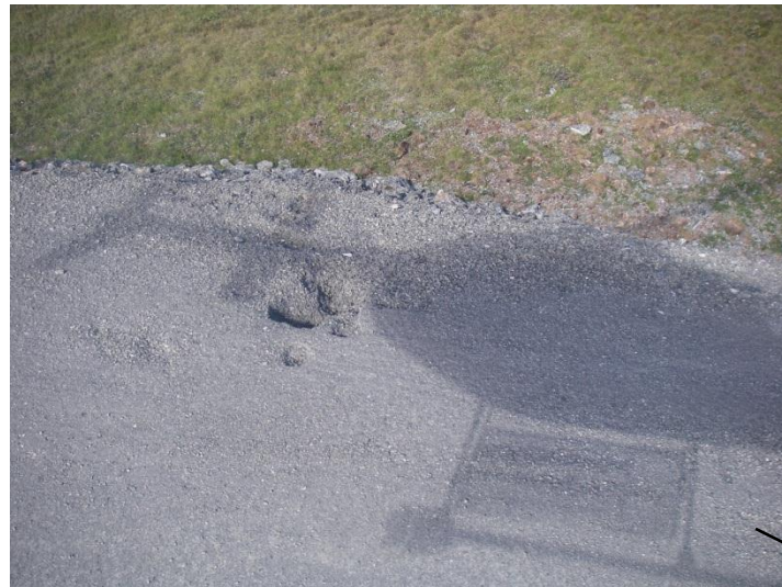
Settlement/ Pothole along the edge of the road
