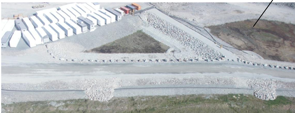
Rip rap aprons constructed for water dissipation, at pond culvert outlets
