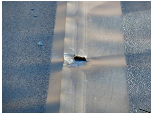
A puncture in the liner at the top northeast corner of the Sedimentation Pond
