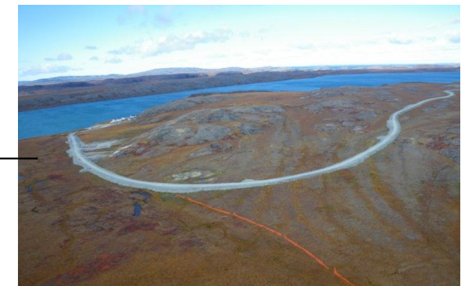
Doris-Windy Road leading to Windy Camp where no surfacing material has been placed
