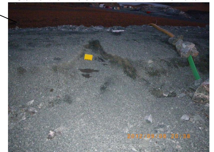
Exposed liner along the crest of the Berm
