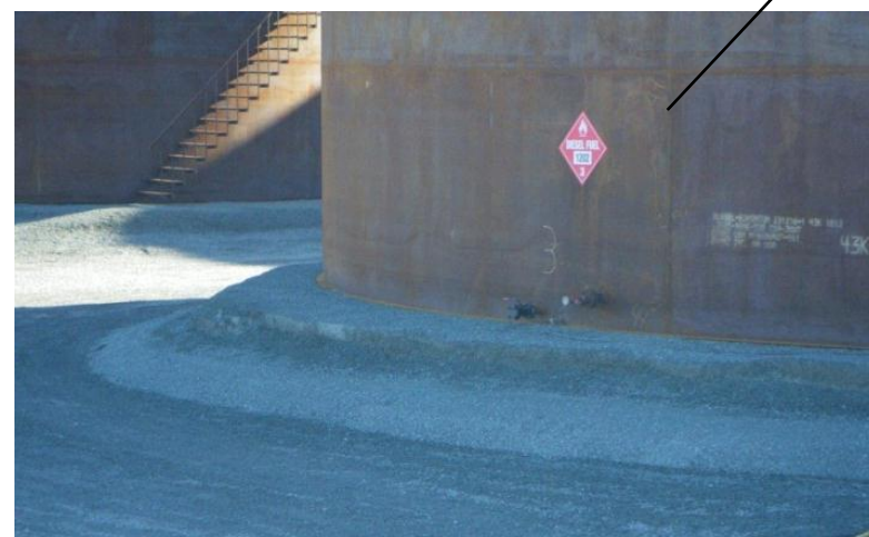
Pedestal of Tank #3 that has been undercut
