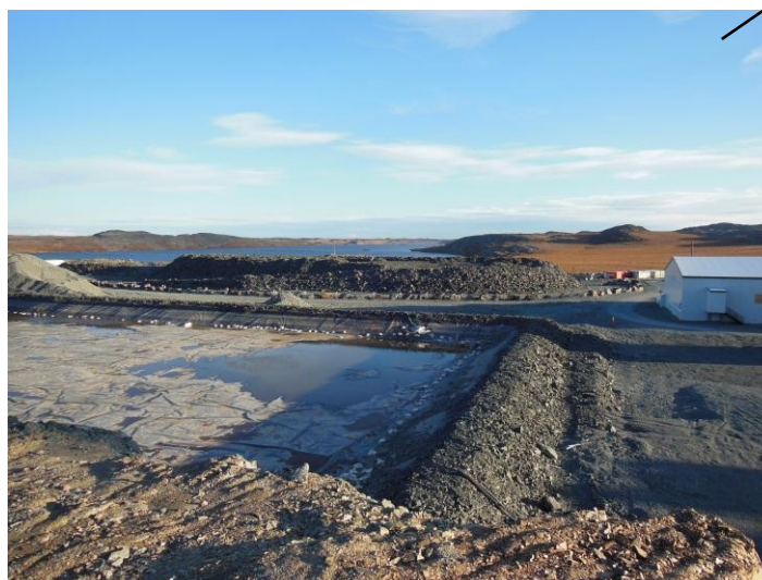
The exposed liner in the Temporary Pond on Pad D. Looking south from the Doris North Access Road
