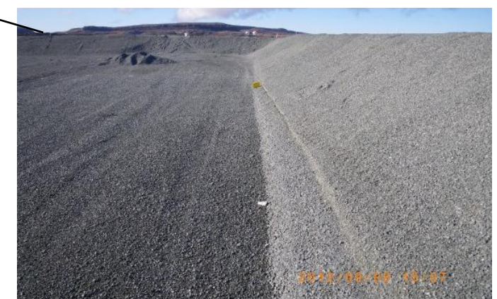
Interior Berm that shows evidence of wheeled traffic. Looking north from Tank #3
