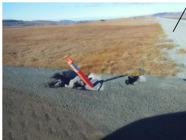
Sinkholes and erosion gully on the south edge of the South Apron
