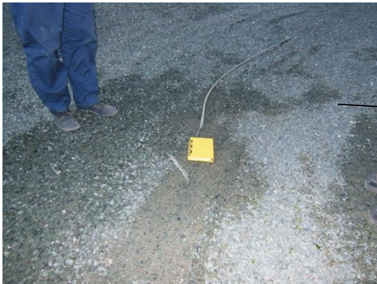
Exposed Grounding Cable in the 5ML Fuel Tank Farm in Pad R
