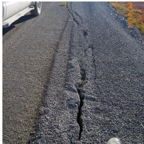
Tension cracks along west side of run-way
