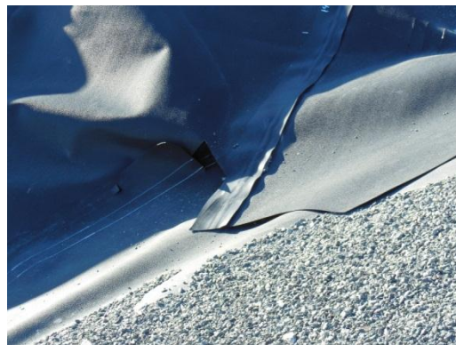
A gap in the overlap of two liner panels that has not been welded
