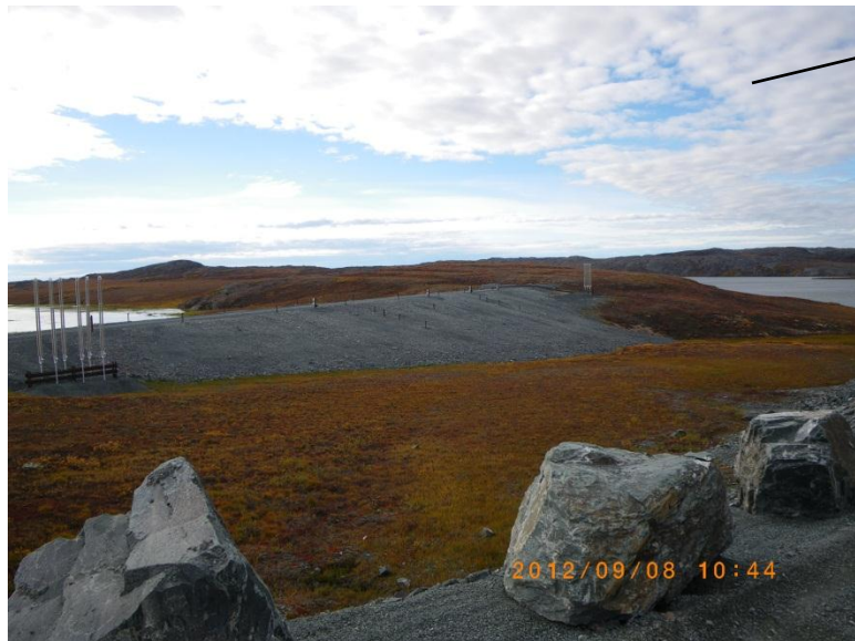
Instrumentation installed in the downstream face of the North Dam
