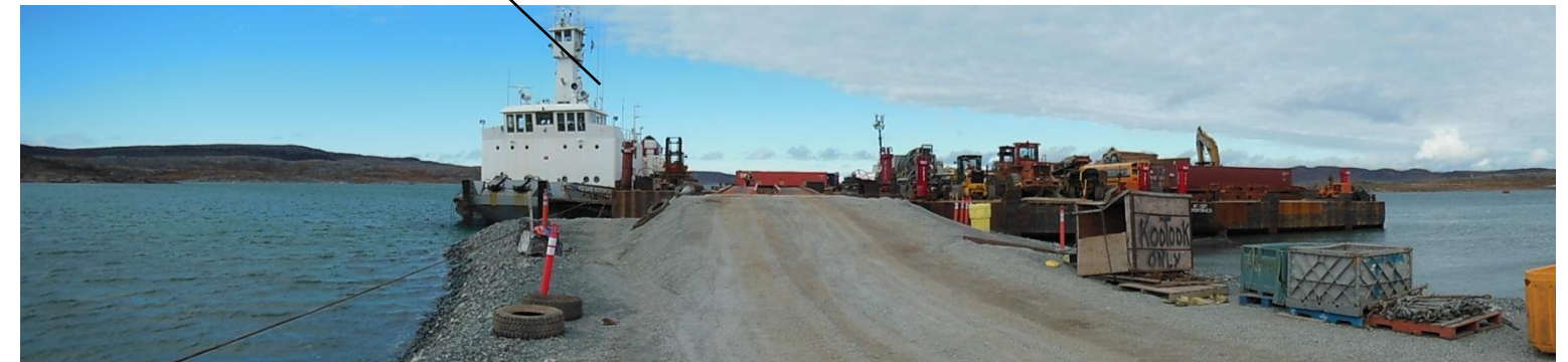
North end of Jetty showing earth fill ramp to resist loading barges – looking north
