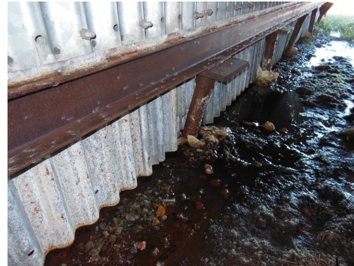
Condition of the battered and straight piles along the north side of Arched Culvert #1
