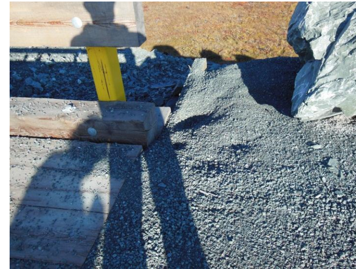
Small sinkholes were observed where the abutment joined the bridges for Stream Crossings #2 and #3
