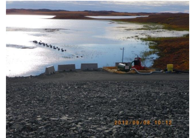
Pump station and water intake line located at the west upstream toe of the dam. The inundated Tail Lake shoreline in the background
