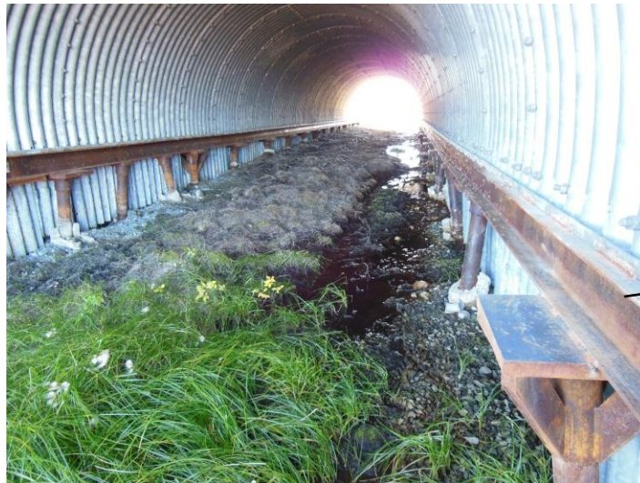
Water running against the north piles around Culvert #1
