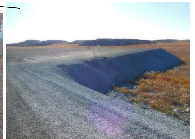
Sinkholes and erosion gully on South Apron
