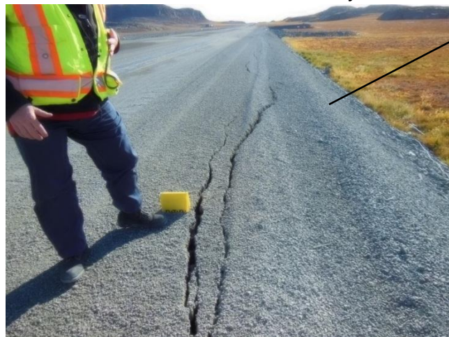
Tension cracks along west side of run-way
