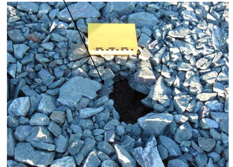
A sinkhole in the upstream face of the North Dam
