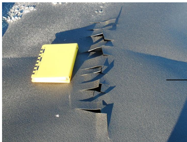
Cuts in the liner at the top northeast corner of the Sedimentation Pond
