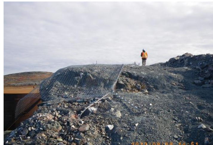
High wall reinforcement along the top of the west high wall
