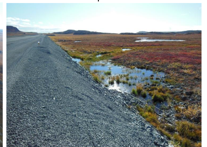
Ponding of surface water along the west side of the airstrip
