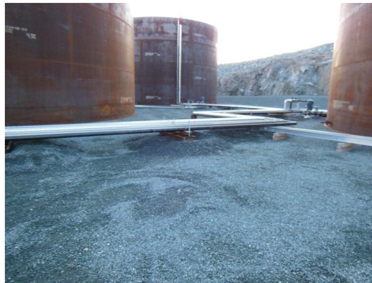
Internal Pipe Supports in the Pad R 5ML Fuel Tank Farm
