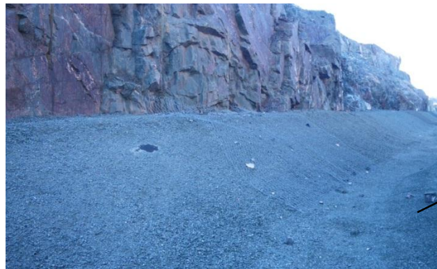
Interior Berm along western high wall showing the liner has been exposed
