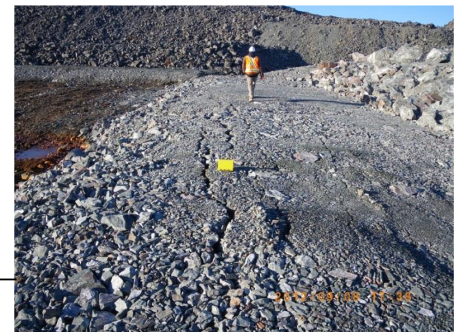
Tension cracks on the interior bench of the Pollution Control Pond
