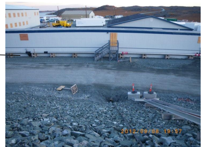
Conduit from the toe of Pad B under the access road coming out by the arctic corridor loading towards the admin and mine day buildings
