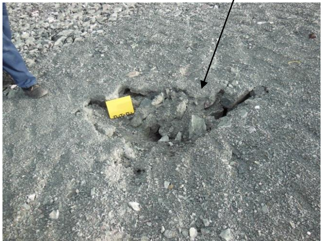
Sink Hole in the downstream face of the North Dam
