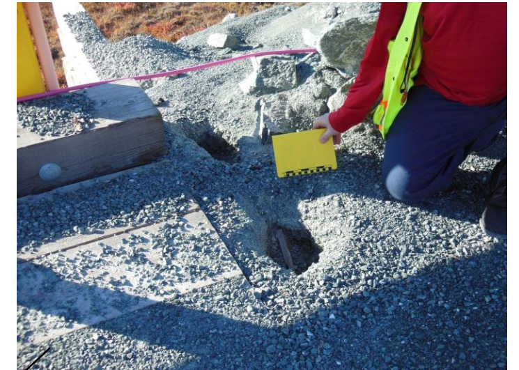
Sink holes were observed where the abutment joins the bridges for Stream Crossing #4
