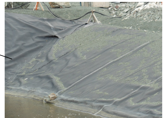
A large rock on the exposed liner at the north corner of the Sediment Control Pond
