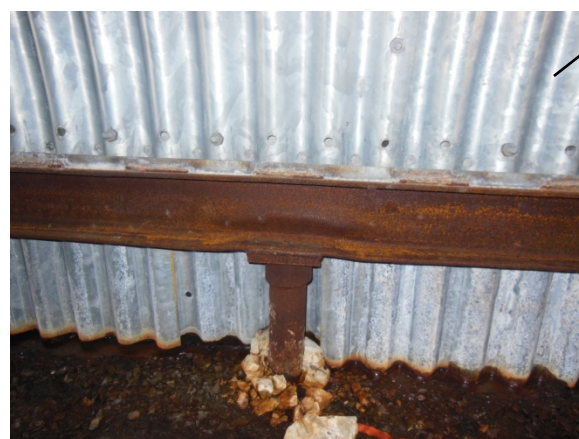
Water running against the north side of Arched Culvert #1
