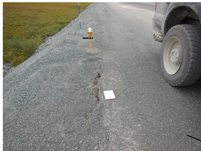
Tension cracks along west side of run-way
