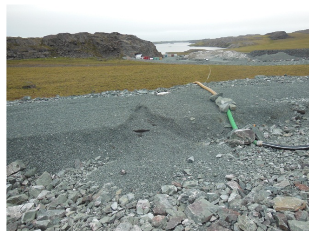
Exposed liner along the crest of the Doris North Diversion Berm
