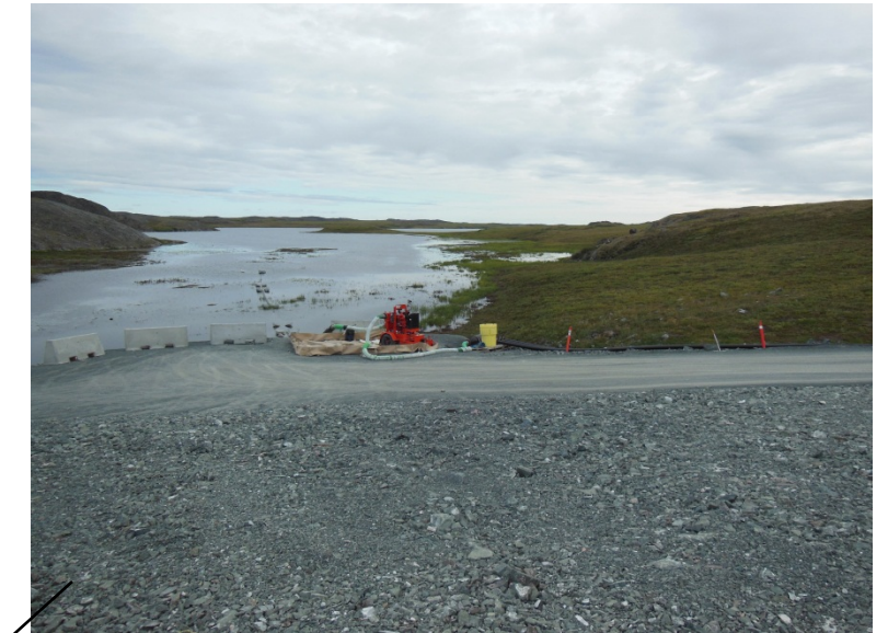
Pump station and water intake line located along the upstream toe at the west side of the North Dam. The condition of the Tail Lake Shoreline is in the background
