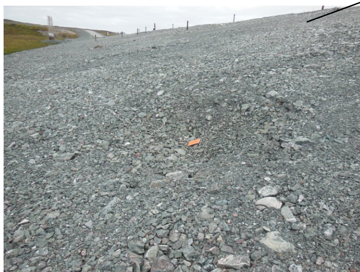
Sink holes in the downstream face of the North Dam
