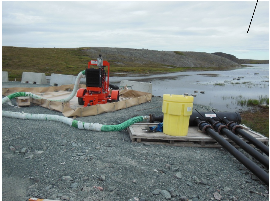
Pump station and water intake line located along the upstream toe at the west side of the North Dam
