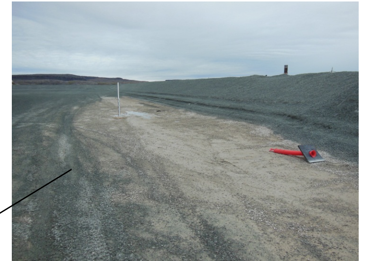
Interior berm along the east side of the 20 ML Tank Farm. Evidence of wheeled traffic along the toe of the berm and high water levels – looking north from Tank #2
