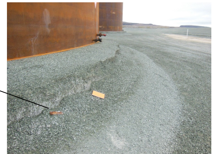
Condition of the Tank #2 pedestal
