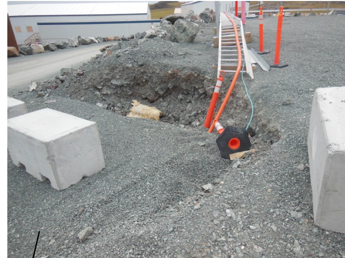
A large erosion gully on the crest of Pad B which can lead to erosion issues
