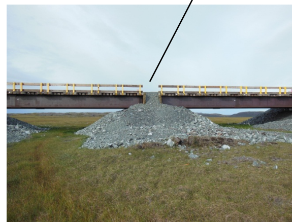
The abutments between the two bridges over Stream Crossings #2 and #3. Water is ponded against the abutment at the toe.
