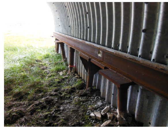
Condition of the battered and straight piles along the north and south sides of Arched Culvert #1
