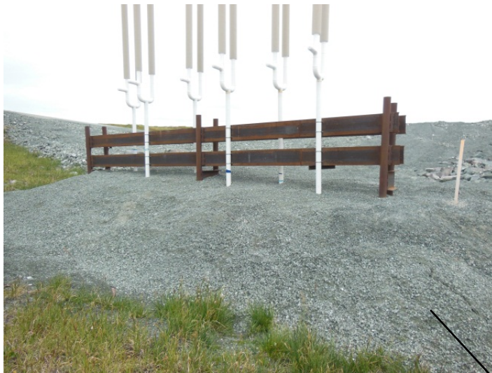
Condition of north radiator foundation. The surface contact thermistor bead appears to be exposed.
