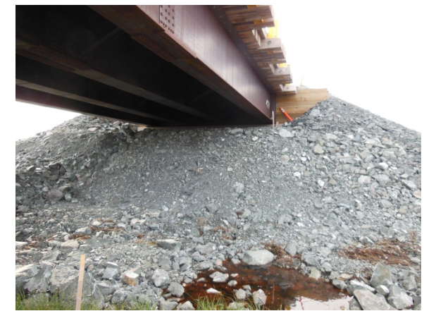
Ponded water against the south abutment of the bridge over Stream Crossing #3
