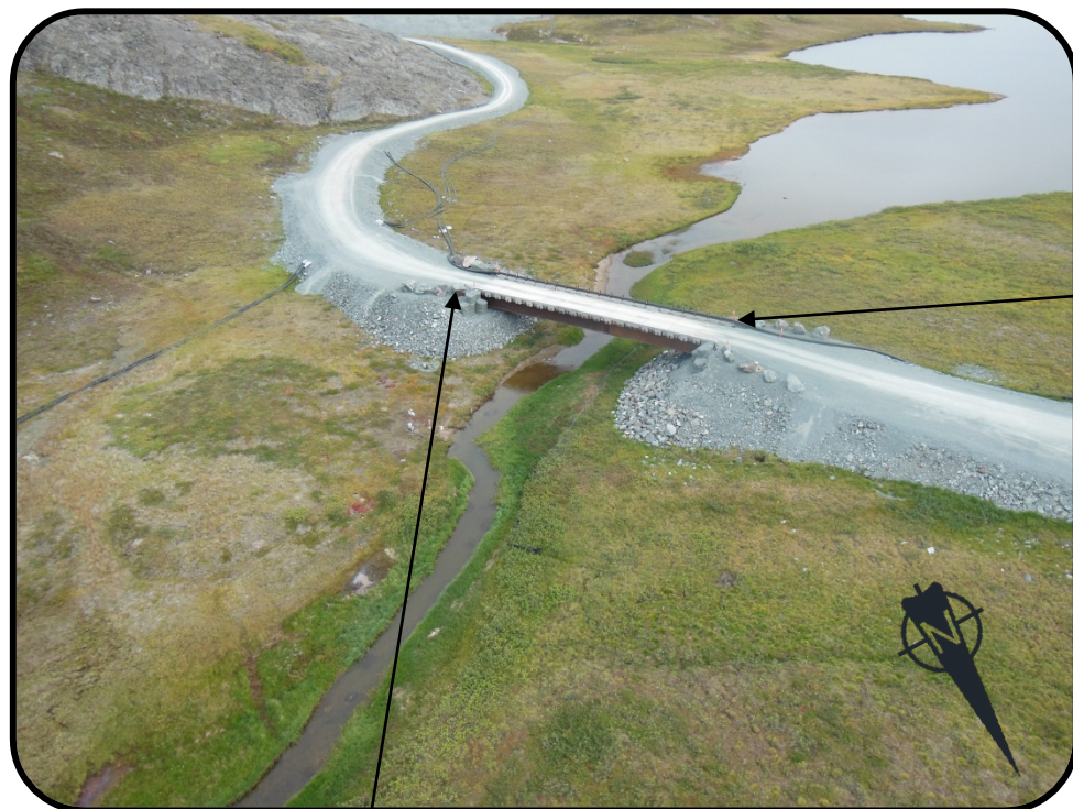
The condition of the rock gabions on the southwest side of the Doris Creek Bridge west abutment
