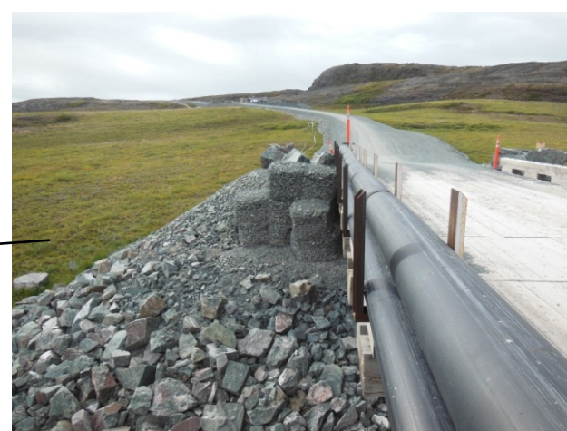
The condition of the rock gabions on the southwest side of the Doris Creek Bridge west abutment
