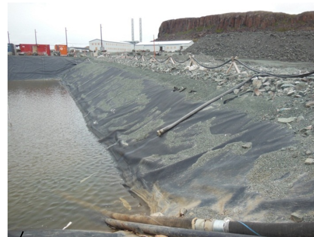
The east side of the Sediment Control Pond. Overliner material from the Divider Berm has washed down on to the exposed liner
