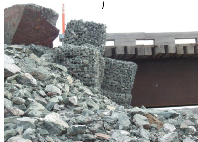
The condition of the rock gabions on the northeast side of the Doris Creek Bridge east abutment
