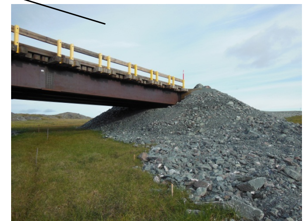
The south abutment of the bridge over Stream Crossing #4
