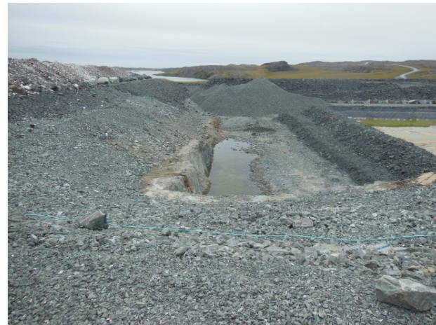
The condition of the east high wall of Pad D. There is water ponding against the high wall.
