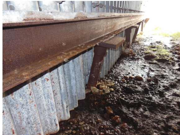
Condition of the battered and straight piles along the north and south sides of Arched Culvert #1
