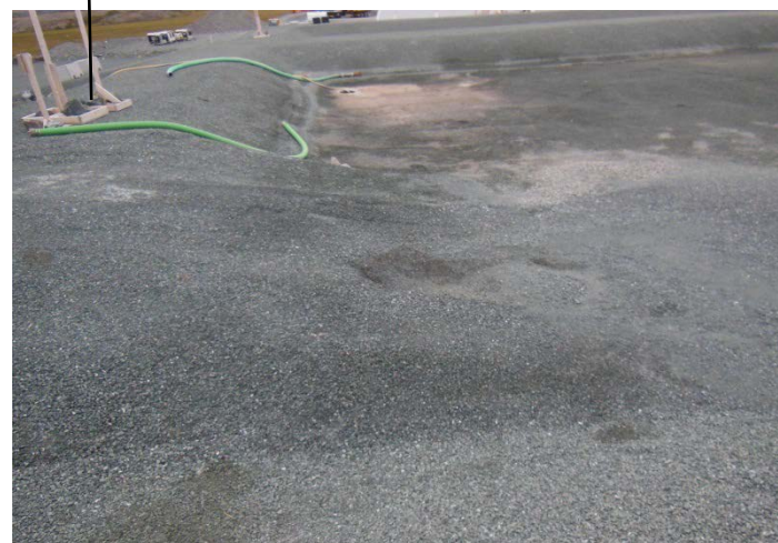
Large depression in the access ramp and condition of the sump in the Snow Pond – looking north
