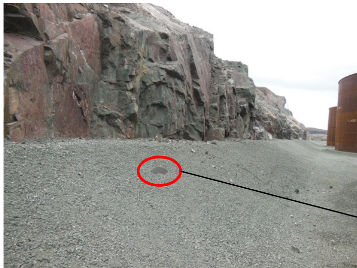
Interior berm along the western high wall showing where the liner has been exposed.
