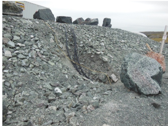
Conduit running down from Pad L and under the access ramps
