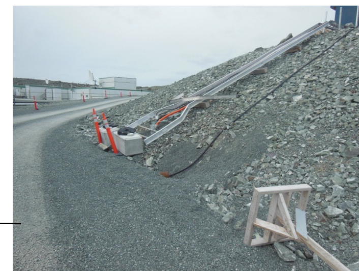
Conduit from the power plant running down to the toe of Pad B and under the Access Road to Doris North Camp
