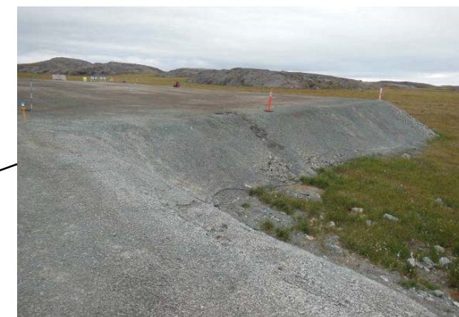
Sink holes and an erosion gully on the north edge of the south apron
