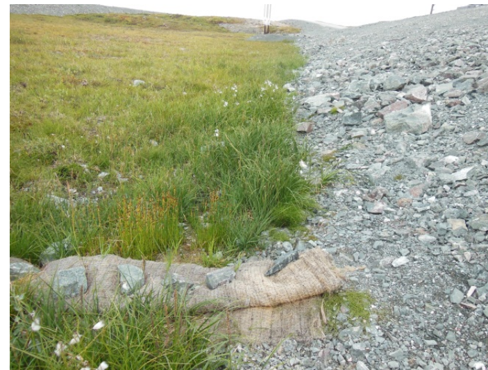
A roll of coconut matting along the down stream toe of the North Dam
