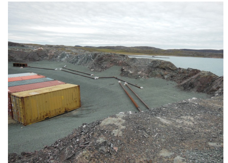
West high wall of the Quarry #1 Tank Farm with the fuel transfer pipes disconnected – looking southwest
