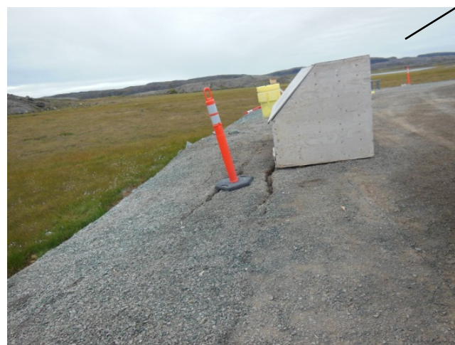
Tension cracks along the south end of the south apron
