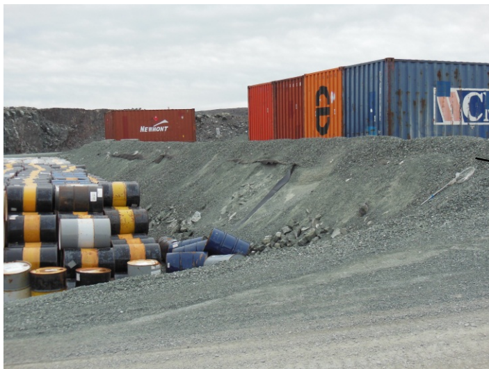
Fuel drum storage and the exposed liner along the back of the fuel transfer station
