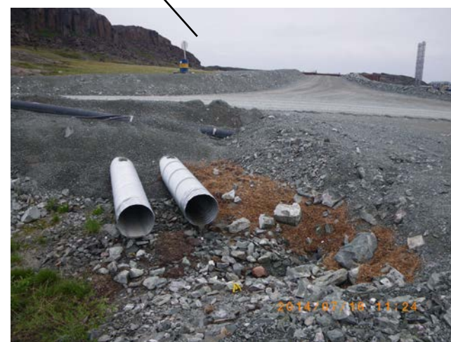
The culverts going under the Primary Road at the junction of the Primary Road and the North Access Road and Doris North Diversion Berm
