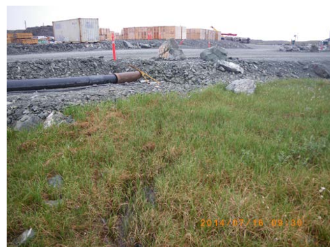
The junction of the Primary, Doris-Windy, and Float Plane Dock Access Roads – the rock fill is 0.5 m thick with surface water into the junction of the roads
