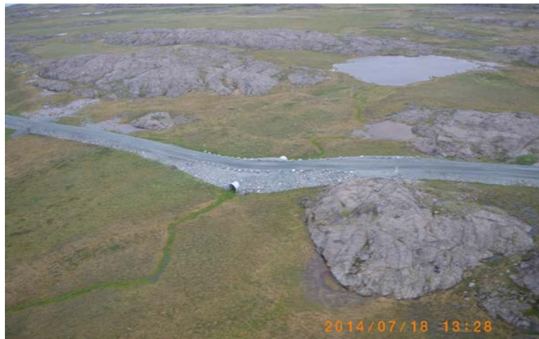
Aerial view of the arched culvert at Stream Crossing #1
