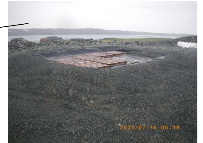
A lined containment area has been constructed at the western edge of Quarry D next to the tote bags of drill cuttings – looking west
