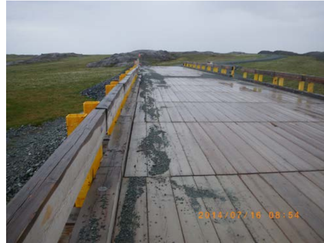
The bridge over Stream Crossing #3 appears to have been shifted as indicated by the decking – looking north from the south end of the bridge
