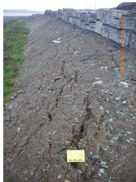
Tension cracks on west side of the Quarry D Overburden Stockpile
