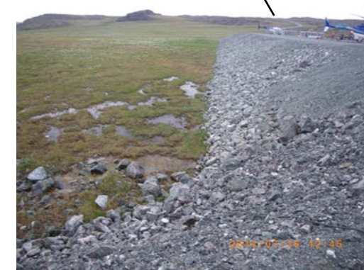
Seepage coming from along the eastern edge of the Helipad – looking south
