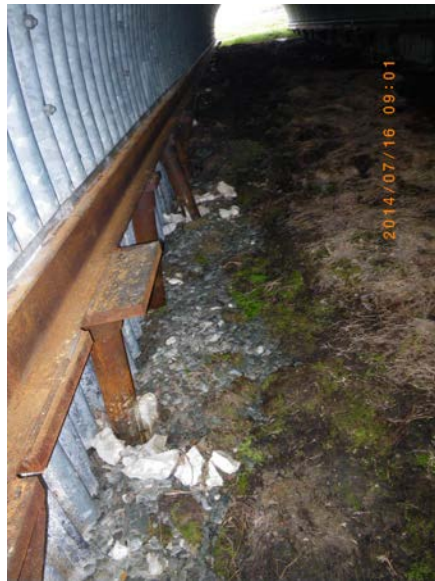
Condition of the battered and straight piles along the north and south sides of Arched Culvert #1
