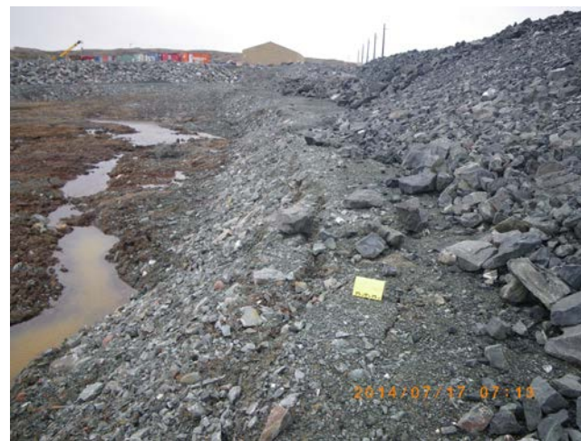
Seepage from the toe of the Waste Rock Pile and from the toe of Pad I. Tension cracks have developed along the crest of Pad I Pad I– looking west
