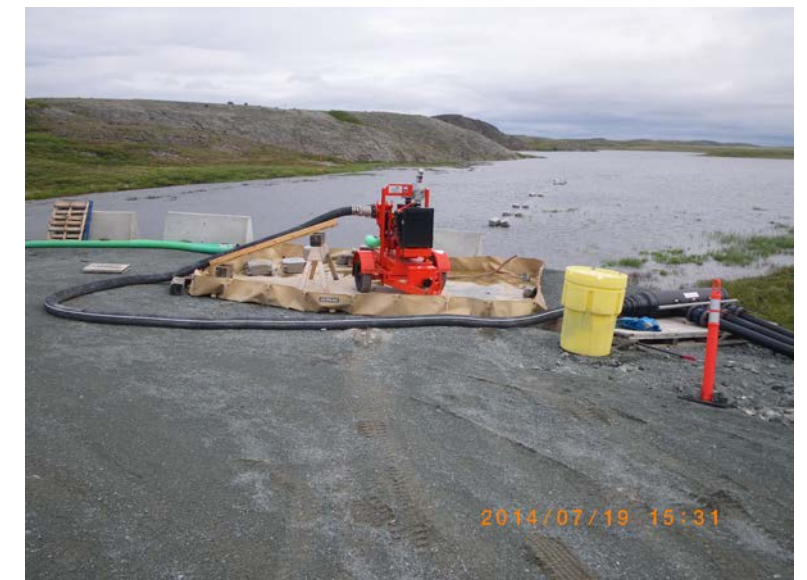
Pump station and water intake line located along the upstream toe at the west side of the North Dam
