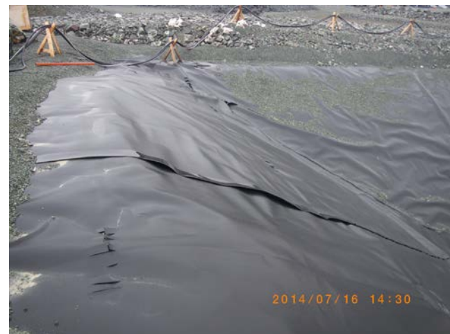
Cuts in HDPE liner along the crest of the Sediment Control Pond at Pad E/P
