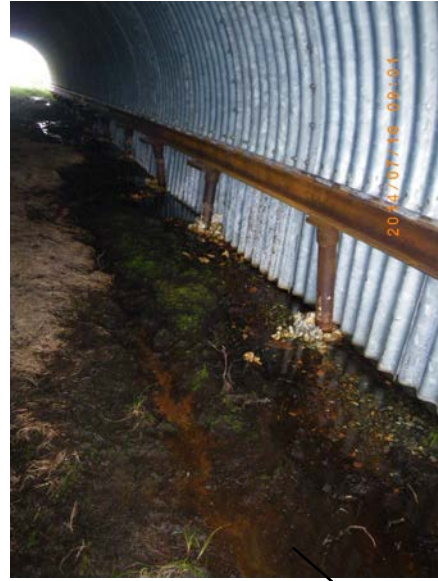
Condition of the battered and straight piles along the north and south sides of Arched Culvert #1
