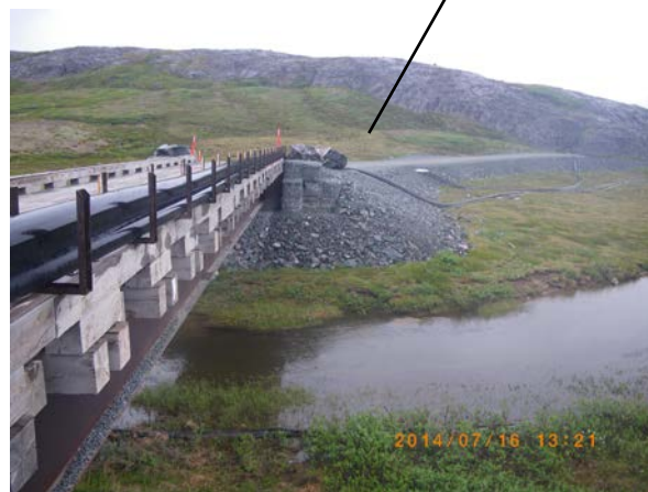
Southeast abutment and rock gabions at the Doris Creek Bridge
