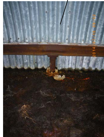
The condition of the I-beam along the south side remains unchanged
