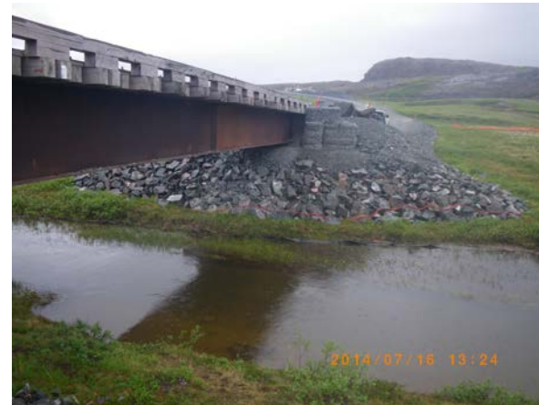
Northwest abutment and rock gabions at the Doris Creek Bridge
