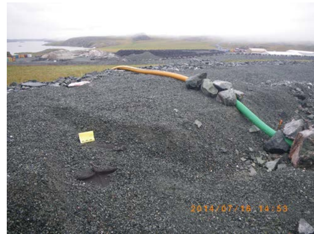
Exposed geotextile along the North Diversion Berm
