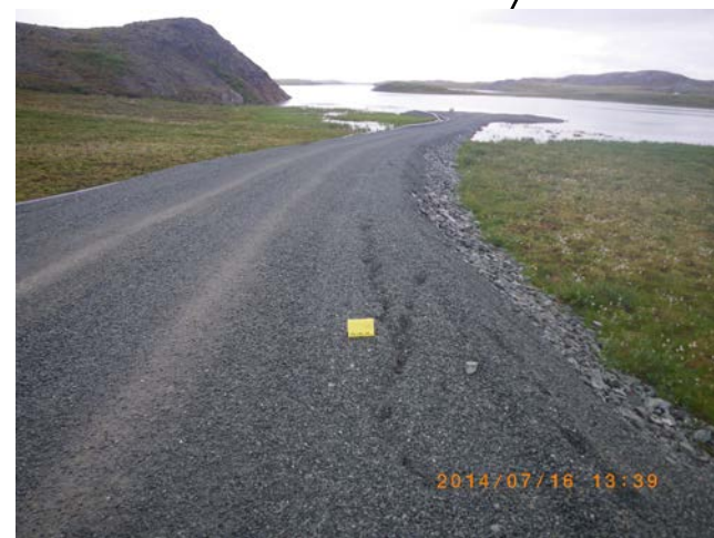
Tension cracks on the south side of the Tail Lake Access Road near the Frozen Core Plant Pad
