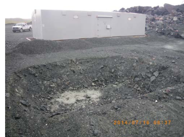
A sump has been excavated in the middle of Quarry B
