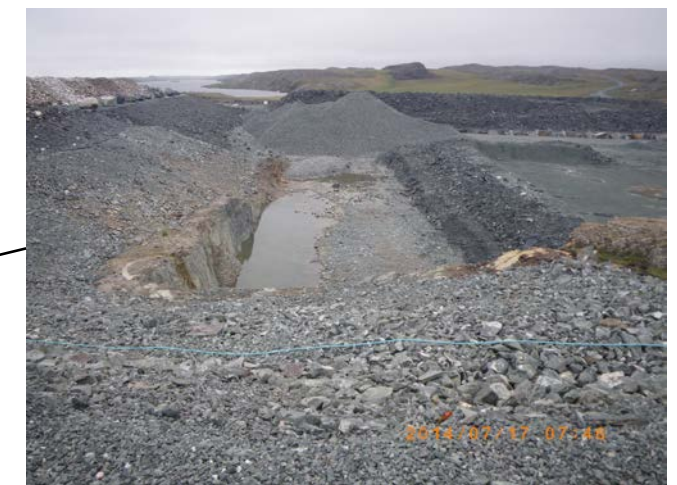
Water ponding by the highwall near northeast corner of Pad D
