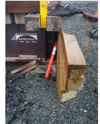
The timber retaining wall at the south abutment of the Bridge over Stream Crossing #3 has also been shifted
