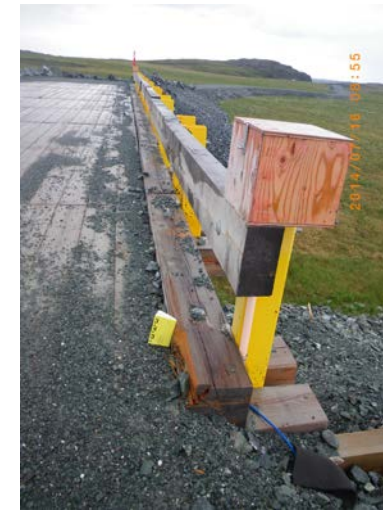
The wooden timber, along the west side, at the north end of the bridge over Stream Crossing #3 has been damaged
