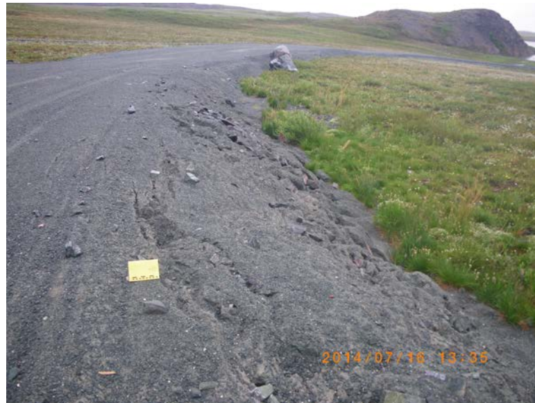
Tension cracks on the south side of the Tail Lake Access Road near the Frozen Core Plant Pad - looking east
