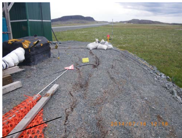
Tension cracks near south corner of the north apron behind the flight tower – looking north
