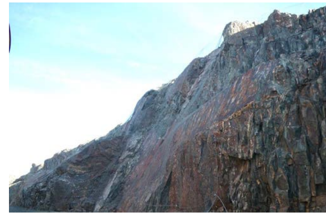
Mesh on high wall protecting the fuel tanks from falling rock – looking up from Tank #2
