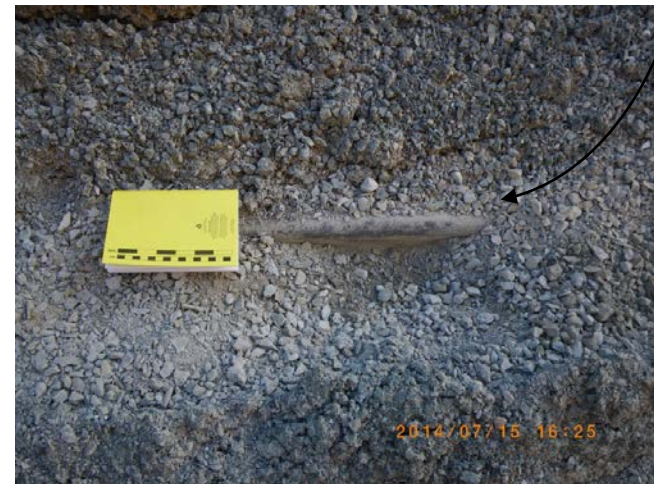
Exposed liner along the containment berm behind Tank #1
