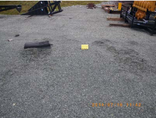
Exposed geotextile along the perimeter of the AN Storage area in the southwest corner of the Upper Reagent Pad
