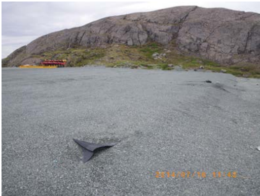
Exposed geotextile along the perimeter of the AN Storage area in the southwest corner of the Upper Reagent Pad
