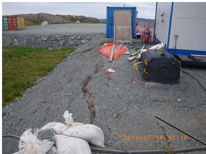
Tension cracks near south corner of the north apron behind the flight tower – looking north
