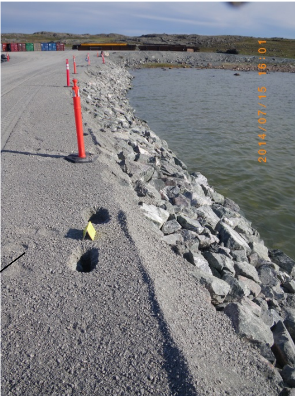
Settlement/Pothole along west edge of Jetty – looking south
