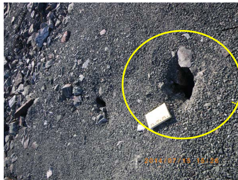
Sink holes at the entrance of the Overburden Dump
