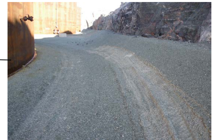
There has been vehicle traffic behind Tank #3. The condition of the liner is unknown – looking southeast
