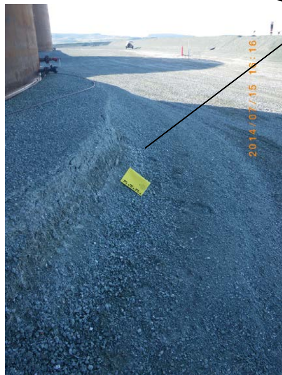
Exposed liner along the containment berm behind Tank #1
