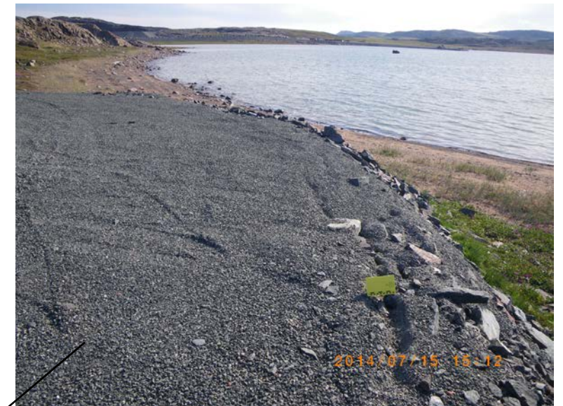
Tension cracks along the crest of the turn-a-round
