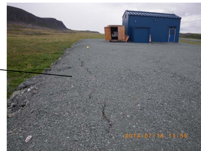
Tension cracks along the crest of the east side of the Wash Bay / Explosives Mixing Plant Pad
