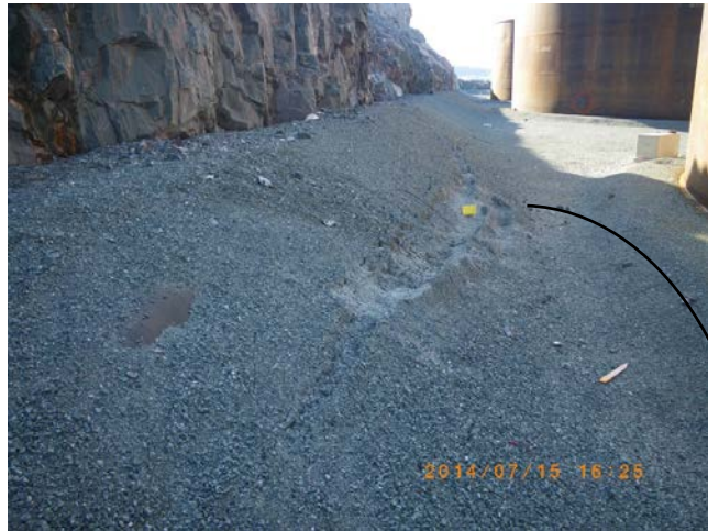
Exposed liner and grounding cable along the containment berm behind Tank #1 – looking northwest
