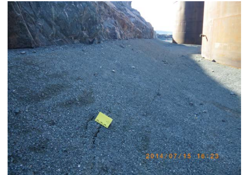
Tension cracks along the berm below the highwall – looking north from Tank #2
