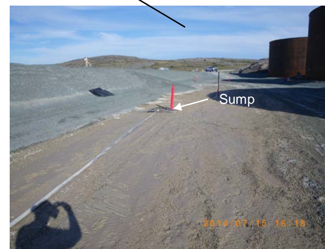
The sump east of the fuel tanks. The area surrounding the sump is covered with fine sediments – looking south towards the access ramp
