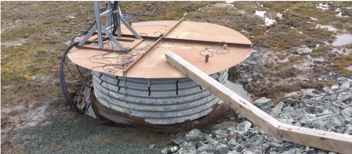
Photo 3. View of Sump #1 showing standing water around the perimeter of the sump which cannot drain due to the lack of drainage holes sufficiently low.
