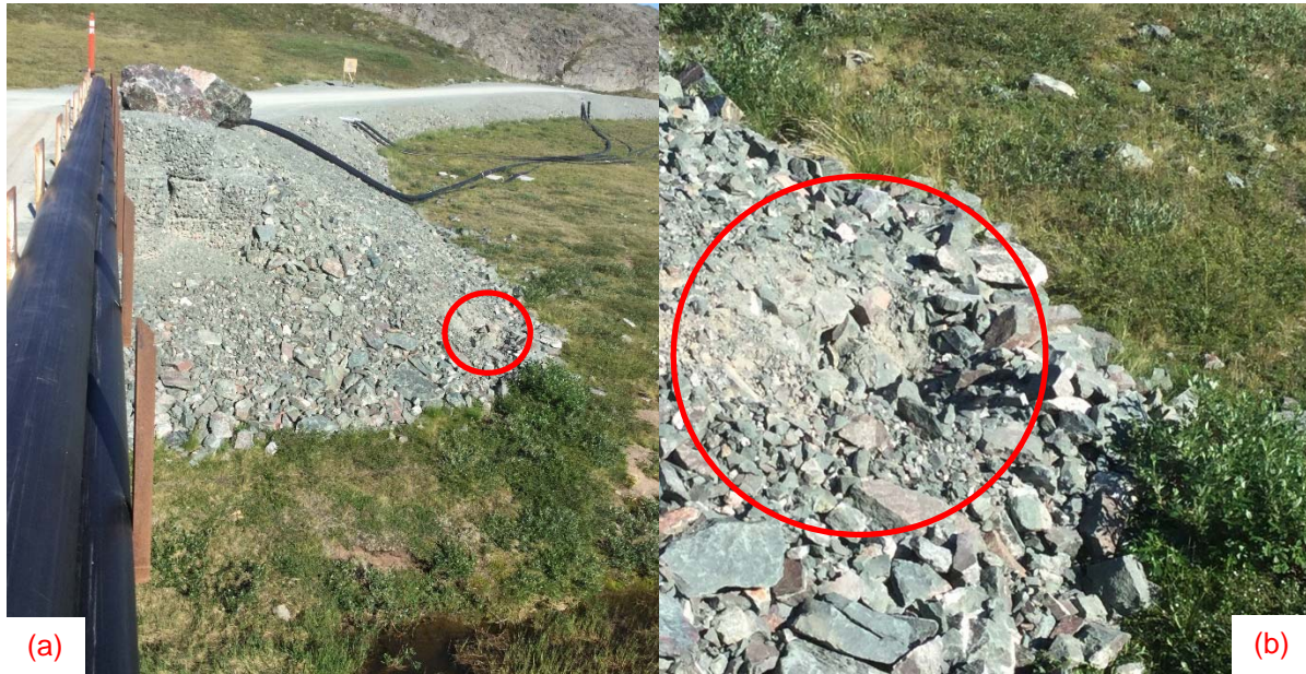
Photo 1. (a) View of south-east abutment of Doris bridge showing location of depression (red circle). (b) Close-up of depression measuring approximately 0.5 m in diameter with subsidence of about 0.3 m
