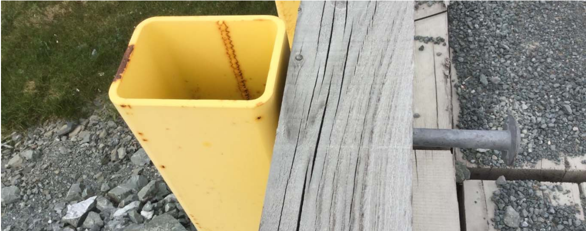
Photo 2. Example of one of the through bolts securing the timber guard rails to the steel bridge posts which loosened itself along the Doris Windy all-weather road
