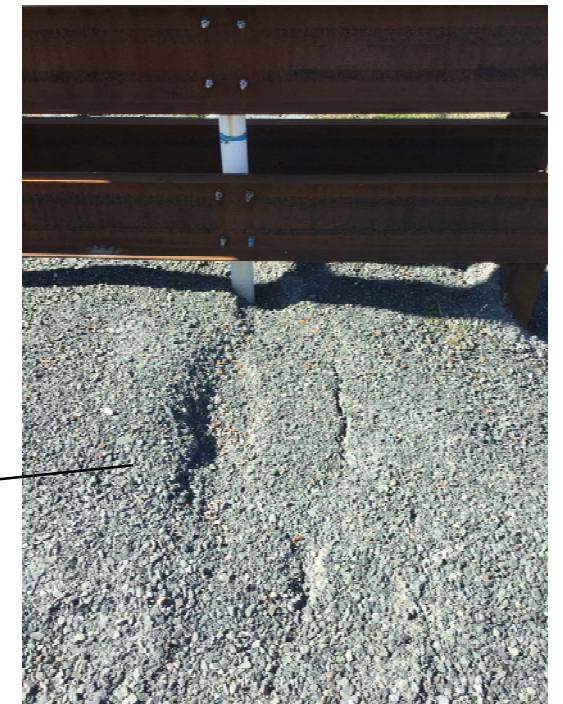
Erosion on the foundation of the North Thermosyphons.
