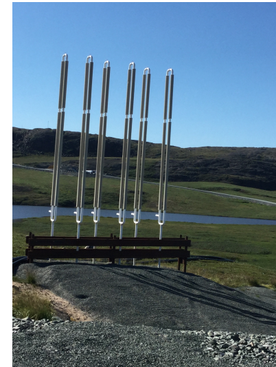
The foundation for the South Thermosyphons.
