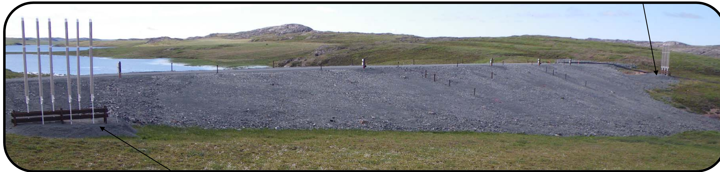
The foundation for the South Thermosyphons.
