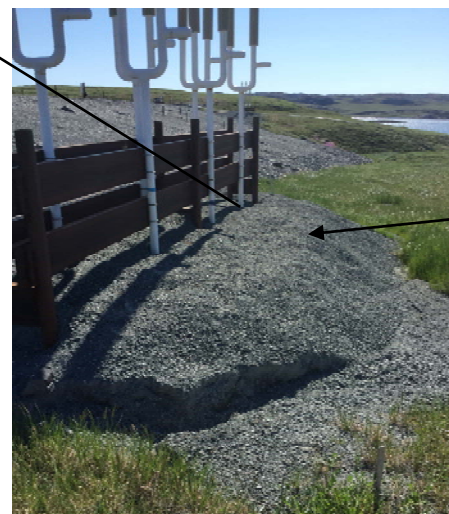
The foundation for the North Thermosyphons, looking west.
