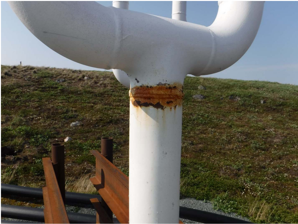
Figure 1- Rust on South Thermosyphon
