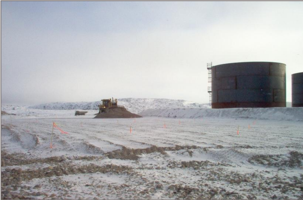
Photo 1: Completed lift of 50 mm fill during construction of the Set 3 Tank Farm in late 2005
