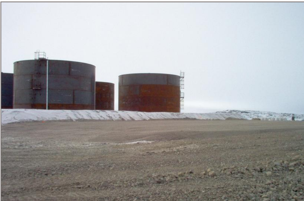
Photo 4: Final grade of 20 mm minus rockfill
