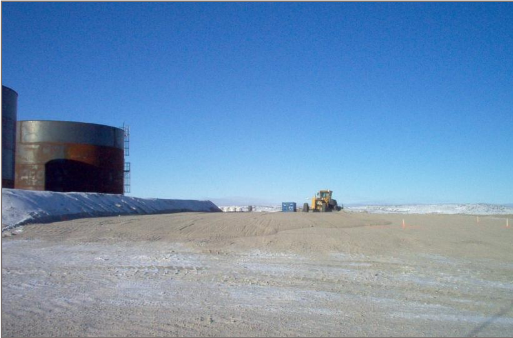
Photo 3: Grader placing single lift of 20 mm minus rockfill
