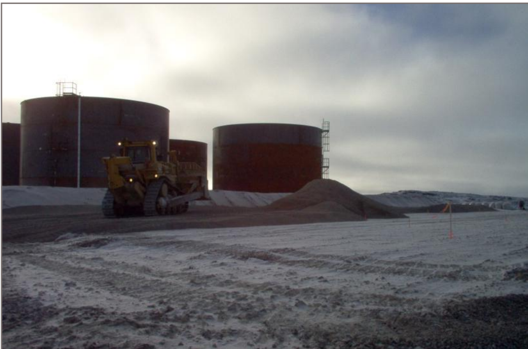
Photo 2: Dozer spreading 20 mm minus rockfill
