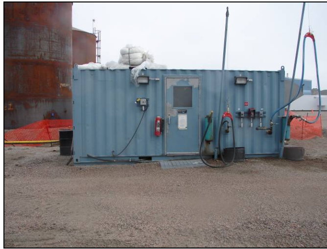
Photo # 10: Fuelling station at the camp's fuel tank farm
