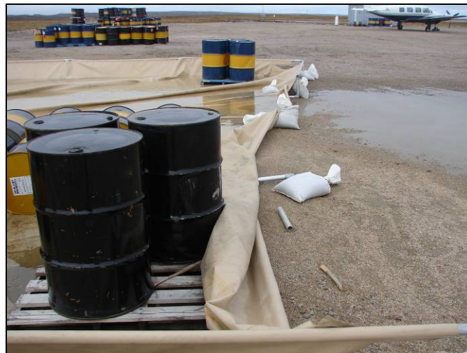
Photo # 6: Close-up of fuel storage containment unit at airport
