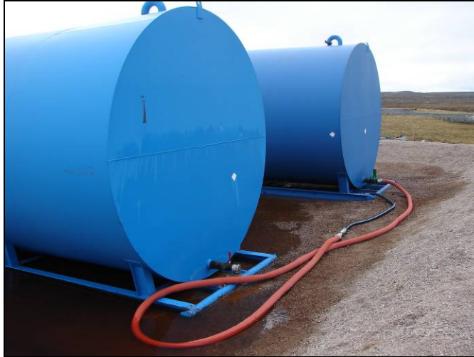
Photo # 23: Two fuel tanks within a fuel berm at the airstrip
