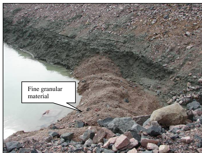
Photo # 16: Reinforcement of permeable barrier – addition of fine granular material to prevent seepage in the structure's corner
