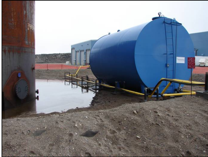
Photo # 21: Small amount of sheen visible on water pooled within the bermed area at main fuel containment area
