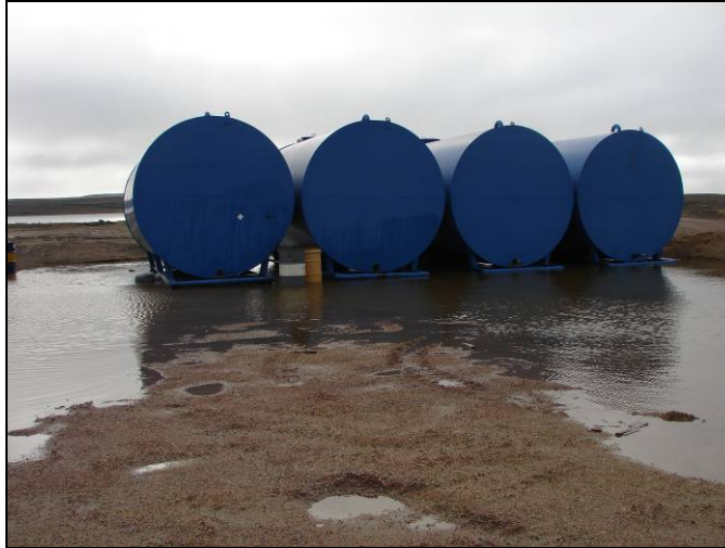
Photo # 25: Fuel tanks holding contaminated fuels within another bermed area (no visible contamination)
