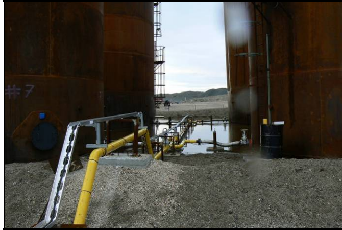
Photo # 16: Standing water within bermed area at Main Fuel Tank Farm
