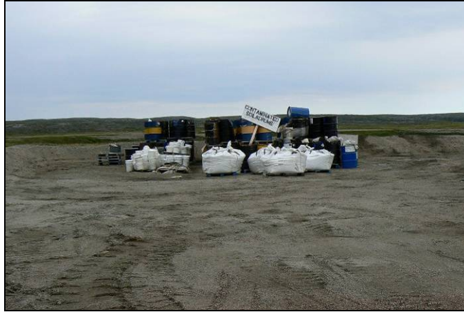
Photo # 25: Waste Transfer Containment Area – West Cell – Drummed and bagged hydrocarbon contaminated soil
