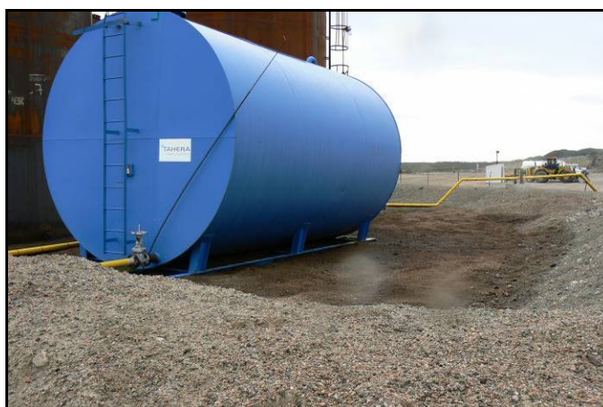
Photo # 15: Contaminated soil within bermed area at Main Fuel Tank
