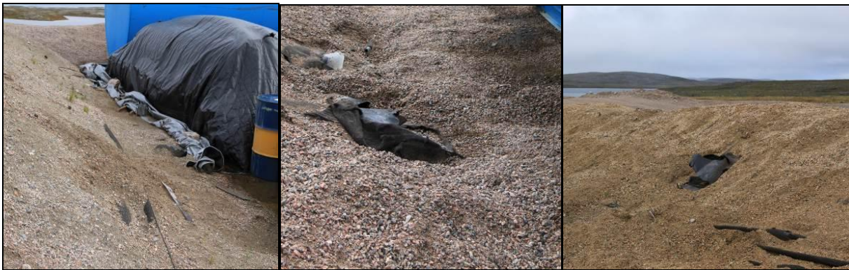
Photo 30: Exposed liner at the Hazardous Waste Transfer Area
