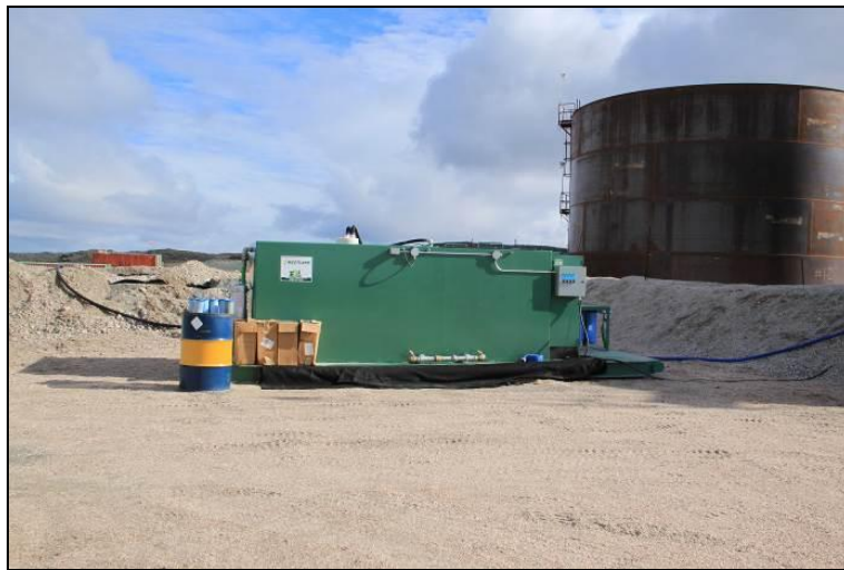
Photo 22: Water reclamation unit (ozonator)
