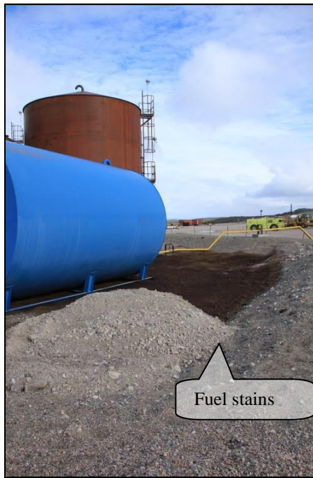
Photo 27: Contaminated soil within bermed area at main fuel tank
