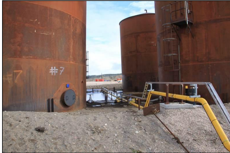
Photo 25: Standing water within bermed area at main fuel tank
