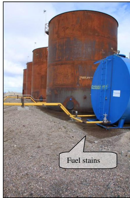
Photo 27: Contaminated soil within bermed area at main fuel tank
