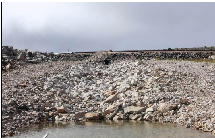
Photo 20: Culvert at C1 Diversion – facing upstream
