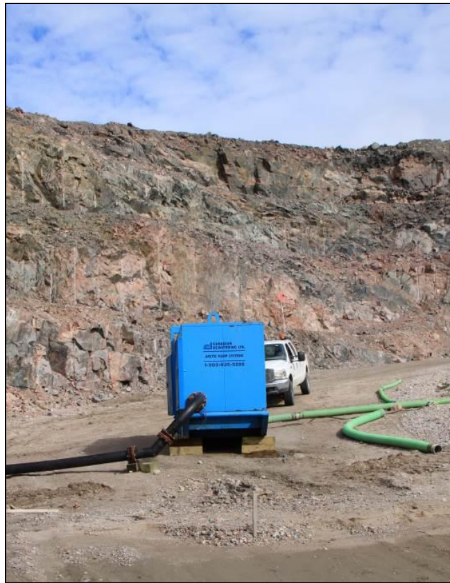
Photo 17: Pump used to dewater pit
