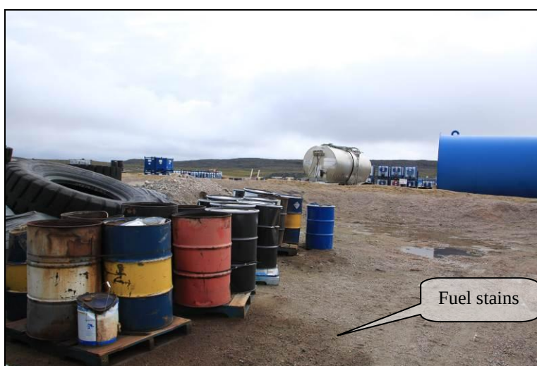
Photo 34: Waste Transfer Containment Area (westerly direction) – bulked and drummed hydrocarbon contaminated soil
