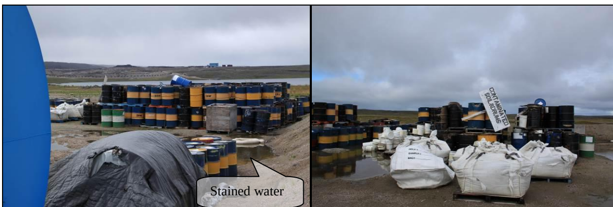
Photo 33: Waste Transfer Containment Area (westerly direction) – drummed and bagged hydrocarbon contaminated soil
