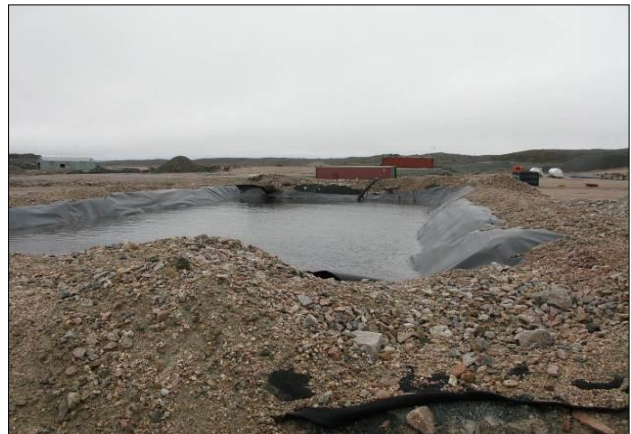
Photo 26: Holding pond for materials being filtered and tested before release
