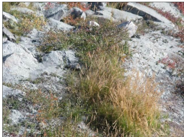
Photo 40: Vegetation growing on slope of East Dam
