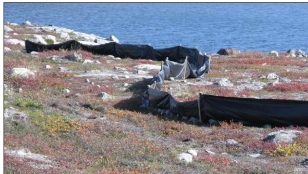
Photo 37: Silt curtain close-up
