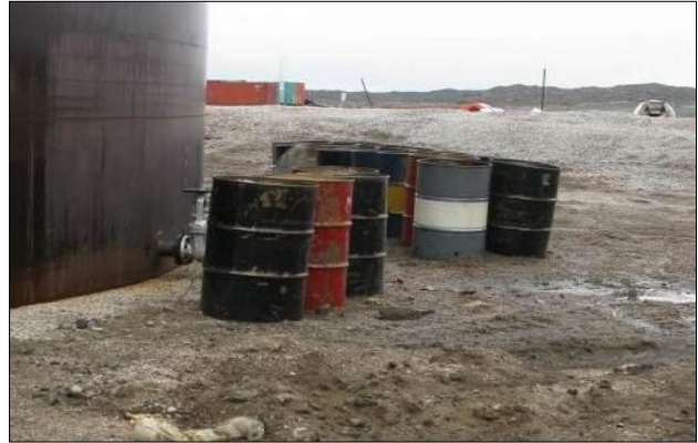
Photo 24: Hydrocarbon contaminated water and debris from within berm being barreled
