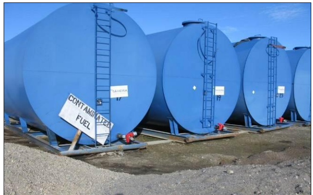
Photo 20: Fuel tanks in waste transfer containment area, note hydrocarbon staining
