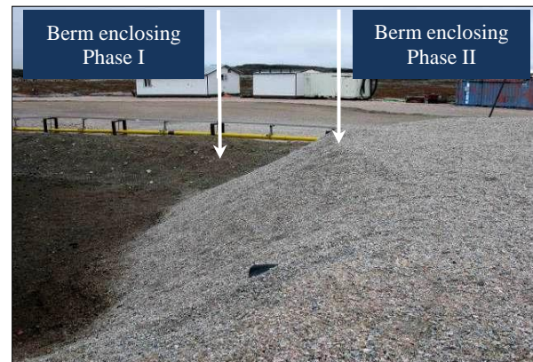
Photo 15: Main fuel tank farm berm between the original Phase I and newer Phase II areas
