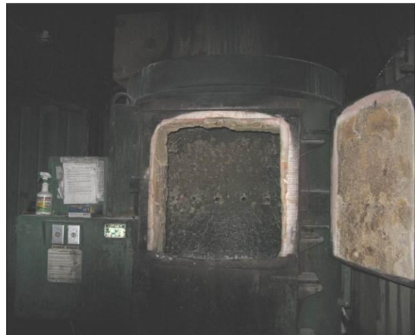
Photo 43: Incinerator unit and chamber
