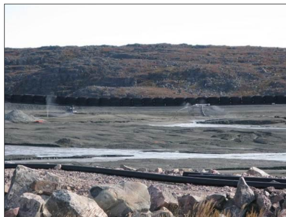
Photo 34: Haul truck tires relocated from berm of mine pit to East Dam
