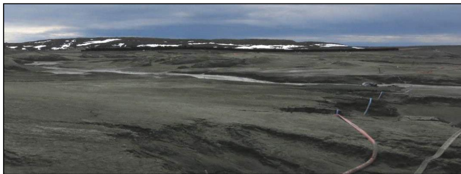
Photo 11: PKCA after spring freshet, top dry, slumping, and developing cracks
