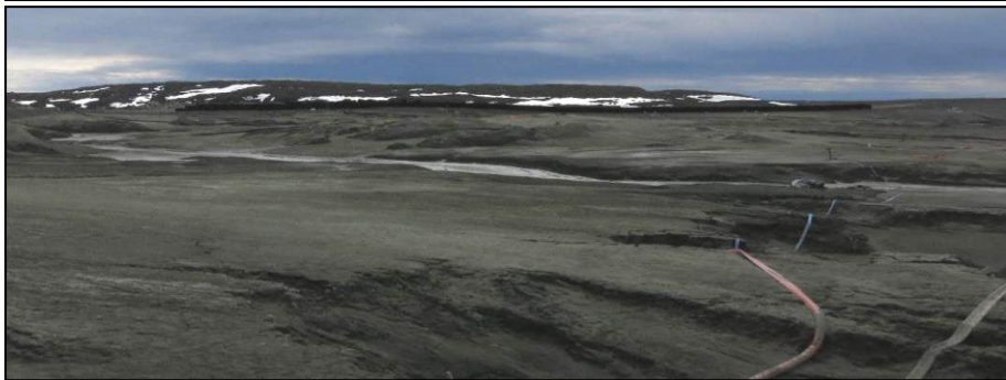
Photo 2: PKCA after spring freshet, top dry, slumping, and developing cracks (2013)
