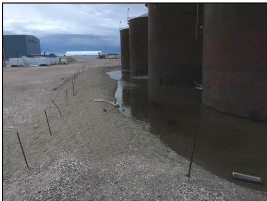
Photo 4: Melt water puddle in bermed area of main fuel tank farm
