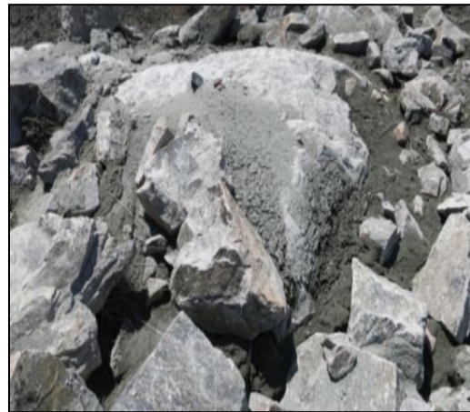
Photo 3: Accumulation of fine processed kimberlite on boulders along Southeast dam
