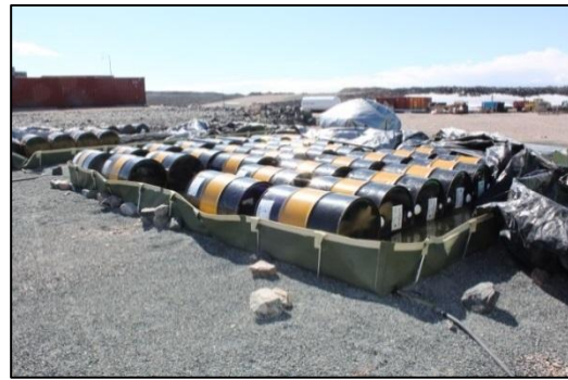
Photo 14: Rock structural support for portable berms near airstrip.
