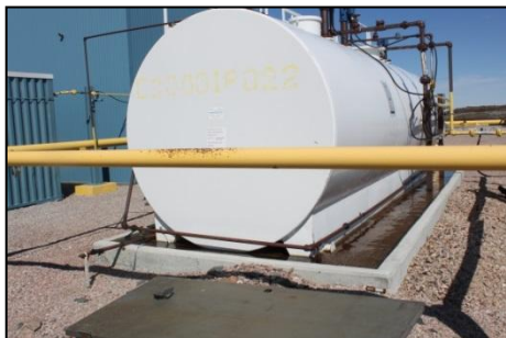
Photo 18: Fuel tank berm at the emulsion plant.
