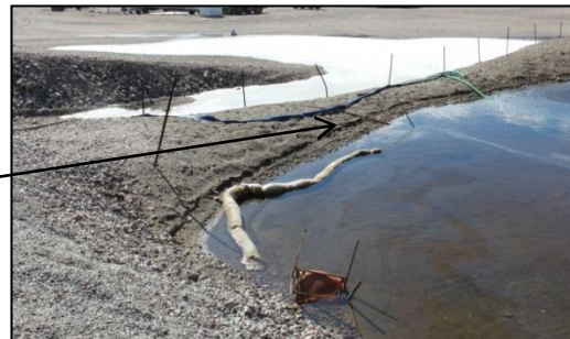
Photo 12: Low spot in berm.
