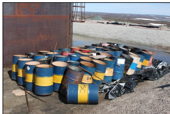
Photo 38: barrels in phase 2 fuel tank farm comparison shot. Tops blown off, water in barrels.
