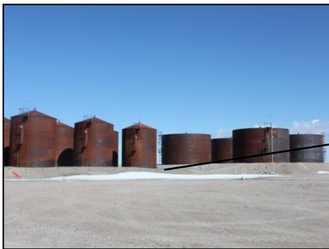
Photo 11: Low spot in the berm surrounding main fuel tank farm Phase 1.
