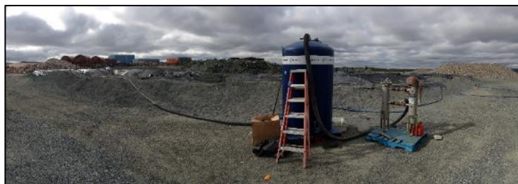
Photo 25: On-site water treatment system for contractor camp greywater
