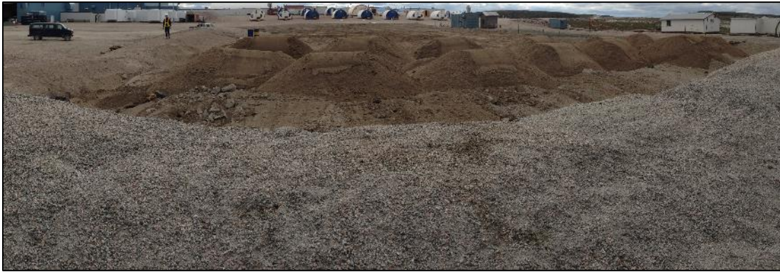
Photo 14: Contaminated soils stored in former Phase 1 tank farm berm to be capped and covered for long-term storage
