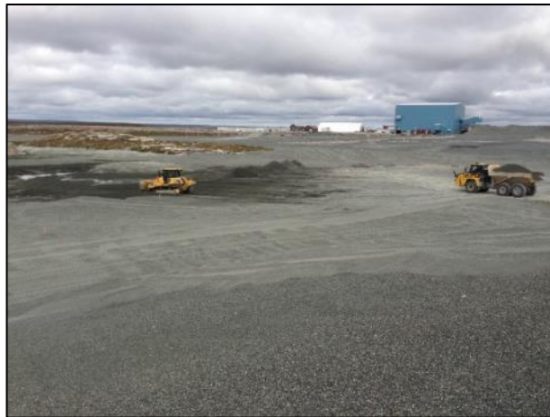
Photo 32: Coarse material being applied over the PKCA
