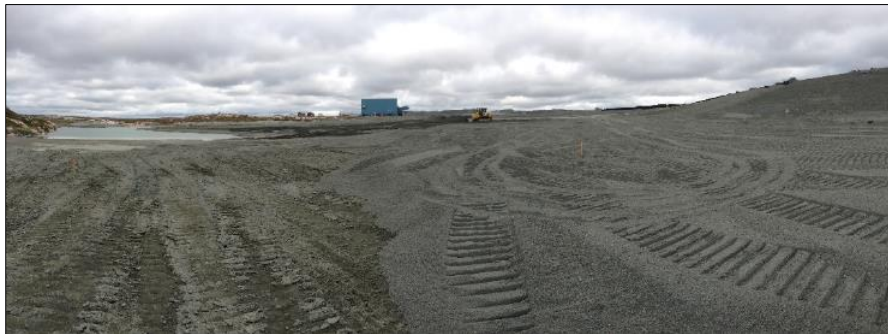
Photo 5: Coarse aggregate (material on right) being applied over processed kimberlite tailings (material on left)
