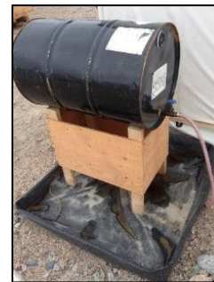
Photo 20: Fuel barrel and containment berm located in the stabilization contractor's soft camp
