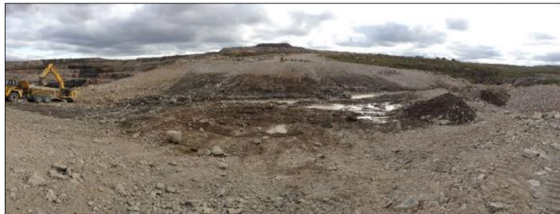
Photo 30: Heavy machinery removing C1 diversion near the open pit
