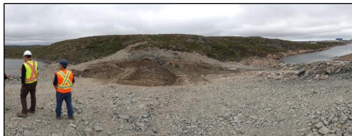
Photo 12: Breached segment of the West Dam where blasting occurred as part of stabilization operations
