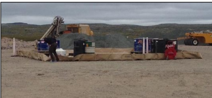
Photo 19: Temporary berm containing fuel barrels near the airstrip
