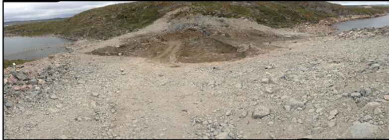
Photo 26: West Dam breach as observed during the 2017 site visit
