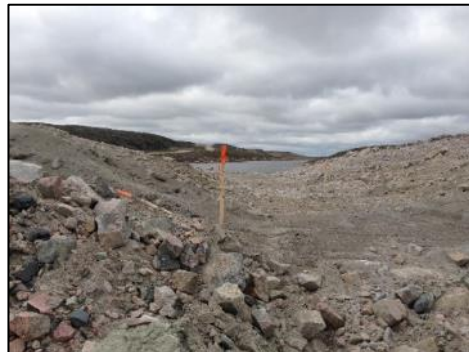
Photo 29: Divider Dyke A breach outflow looking into Cell B/C
