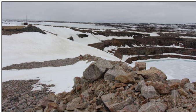
Photo 8: View of the break in the berm surrounding the open pit
