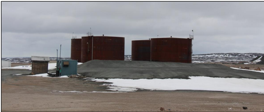
Photo 11: Phase I berm containing contaminated soil
