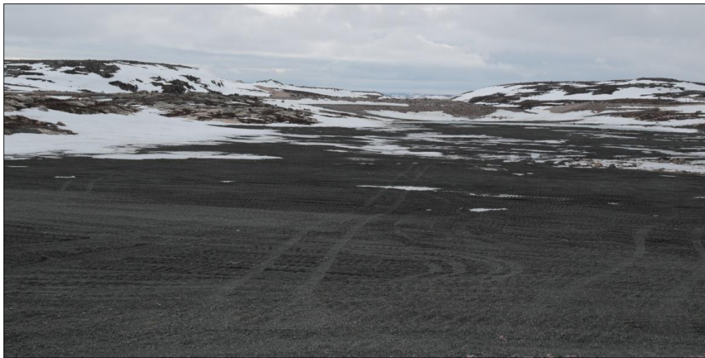
Photo 5: Coarse kimberlite cover on processed kimberlite tailings
