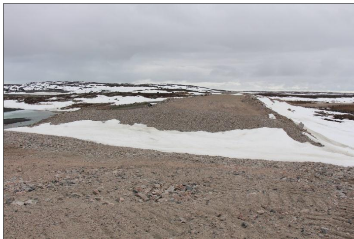
Photo 9: Breached segment of the Divider Dyke A
