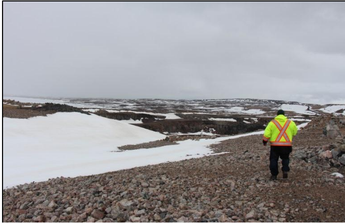
Photo 15: Removal of C1 Diversion and breach of pit wall to re-route water into open pit
