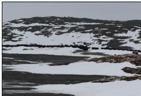
Photo 4: Tire berm used to mitigated dust deposition from PKSA
