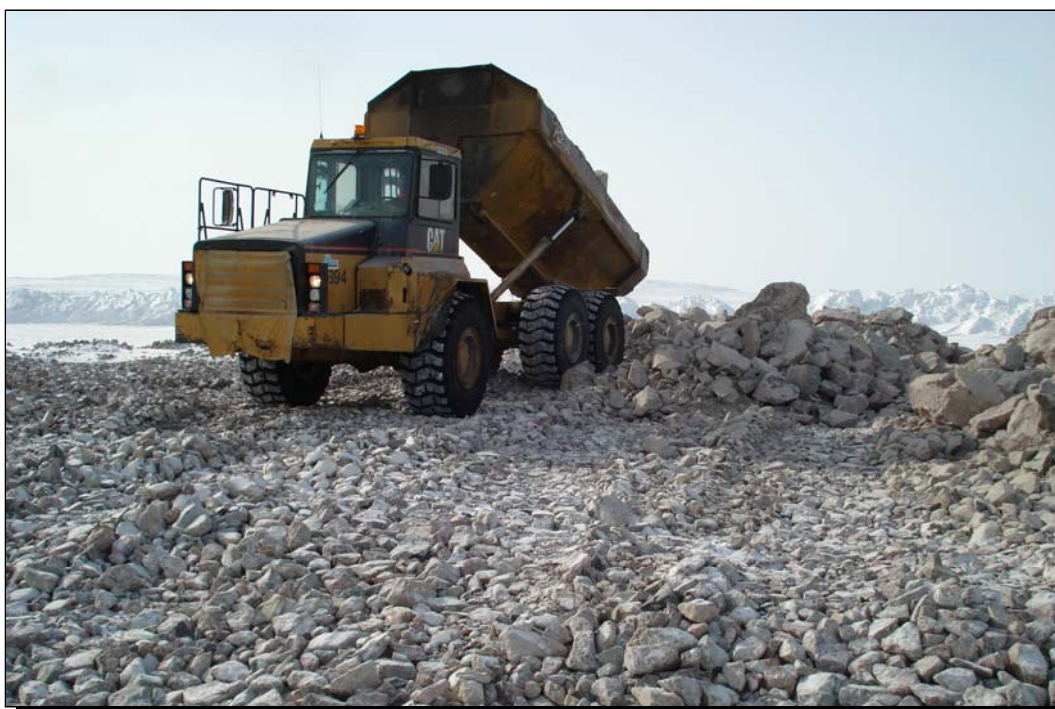
Photo 4 Carat Lake – Dumping rock (ROM) on six inch crush material.
