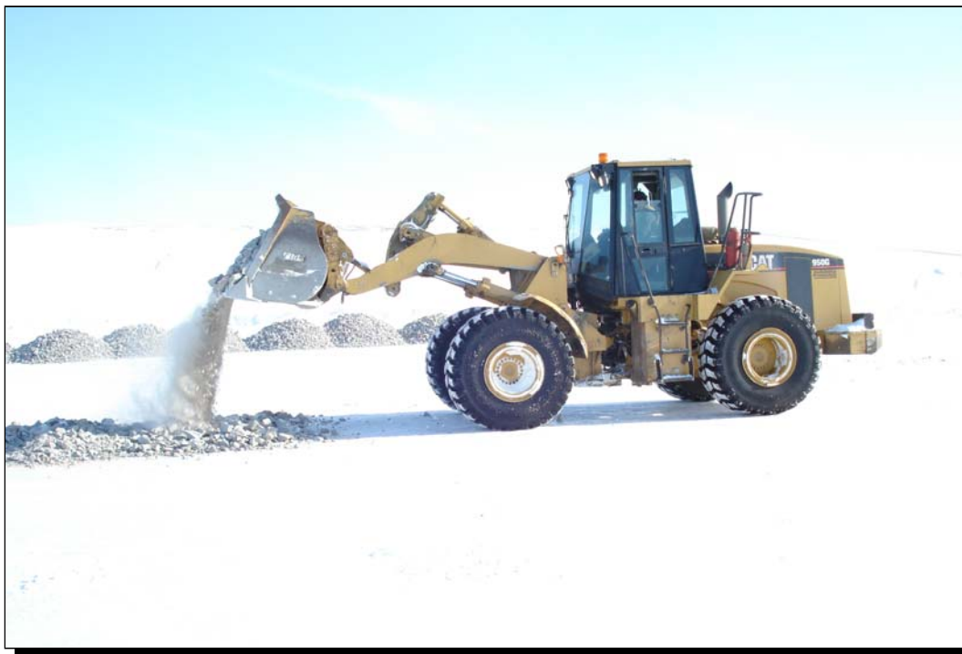
Photo 3 Carat Lake – 950 loader distributes crush material.
