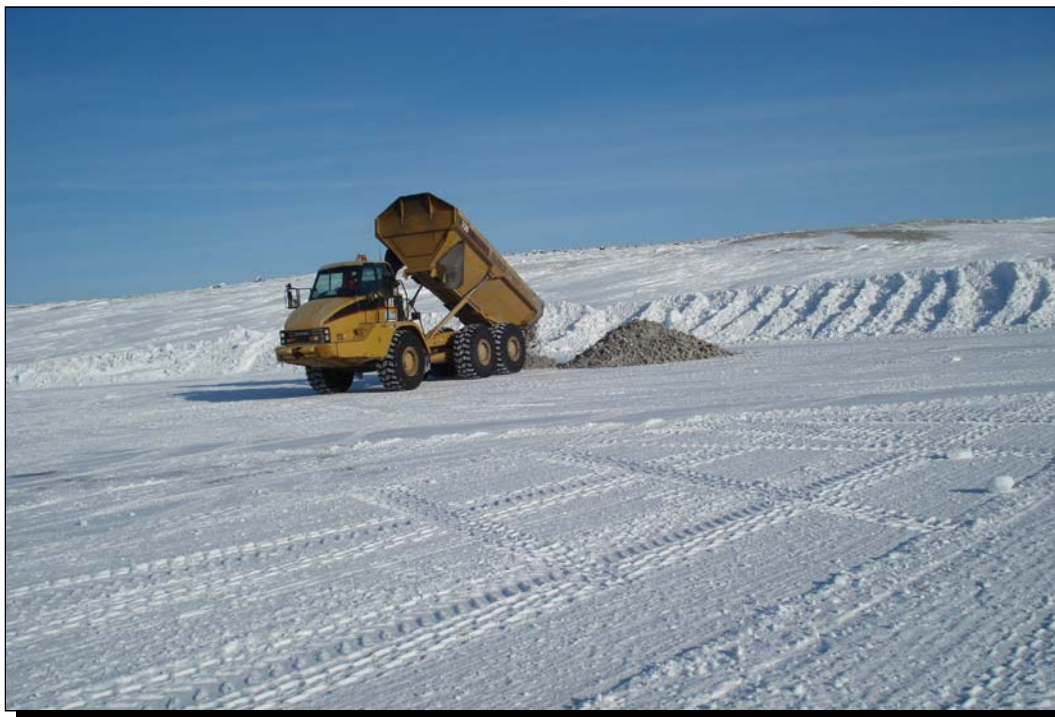
Photo 1 Carat Lake – Dumping six inch crush material on shore fast ice.
