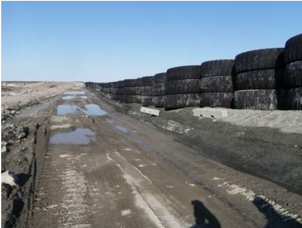
Photo 9 – Tire wall along the Southeast Dam – monitor during snow melt
