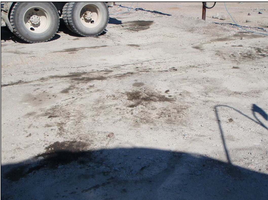
Photo 16 – Truck Shop Parking Area
