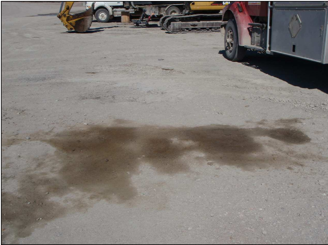
Photo 17 – Truck Shop Parking Area
