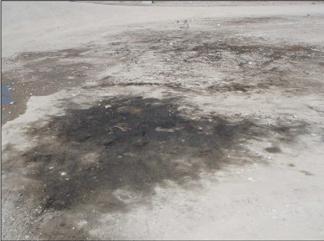
Photo 15 – Truck Shop Parking Area
