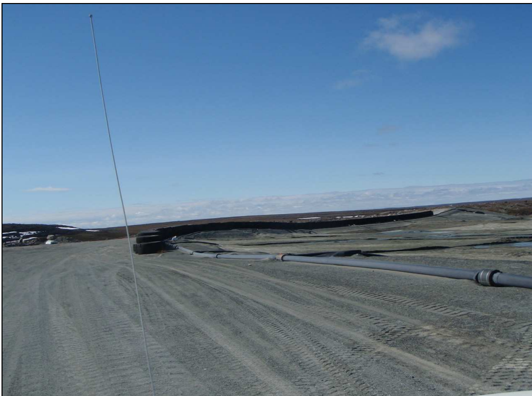
Photo 18 – East and Southeast Dam Tirewall
