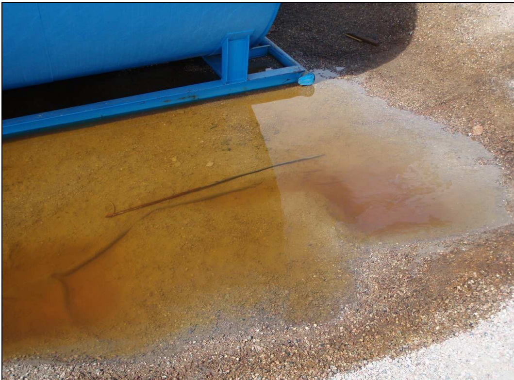
Photo 11 – Airstrip Secondary Containment Berm
