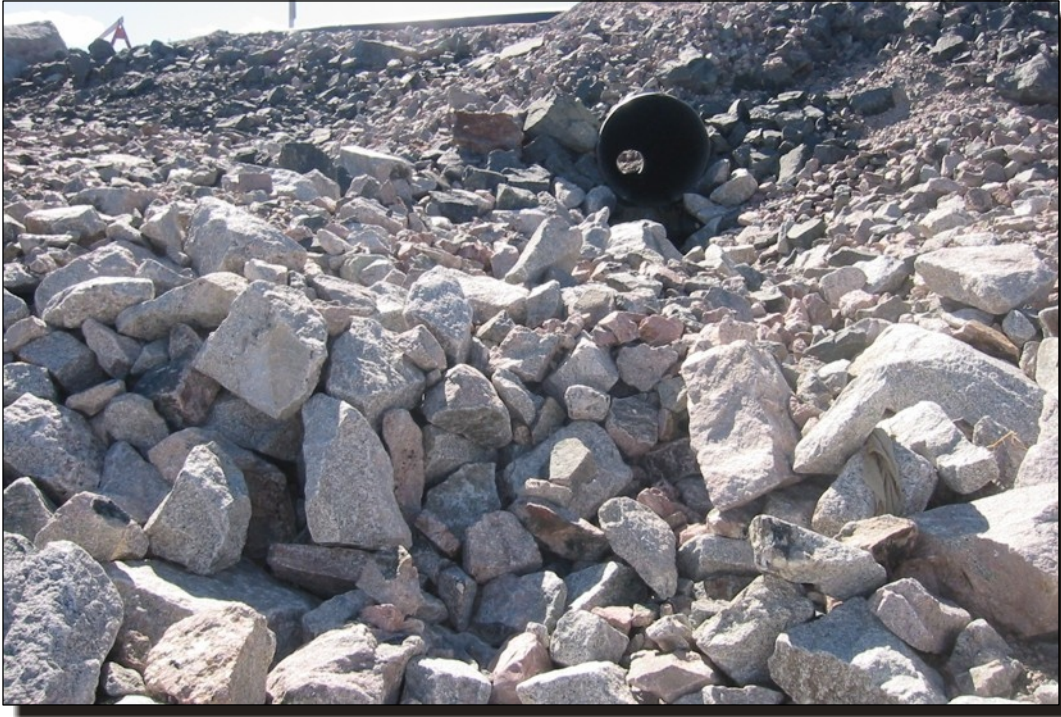
Photo I9 C1 Diversion - Reach B - rip rap below culvert.
