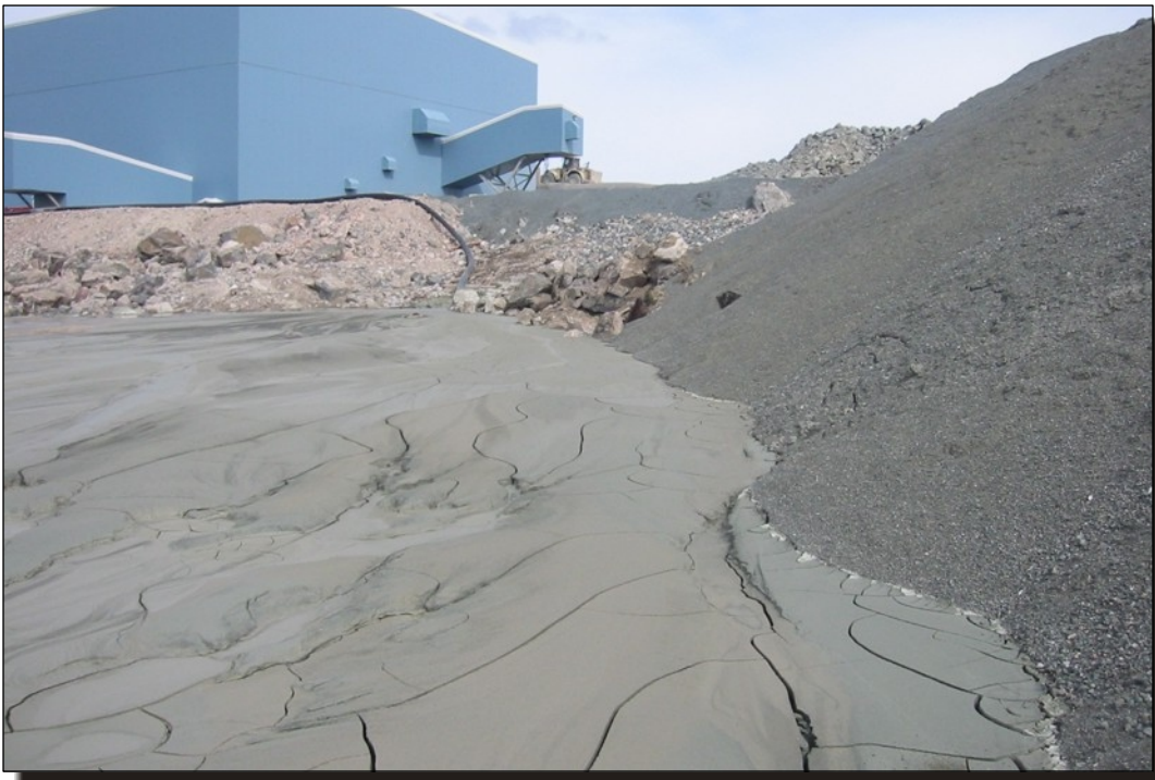
Photo C6 East Dam - Upstream face, fine PK against coarse PK.
