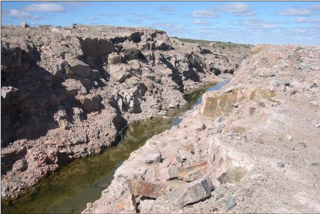
Photo I4 C1 Diversion - Reach A - bedrock cut.
