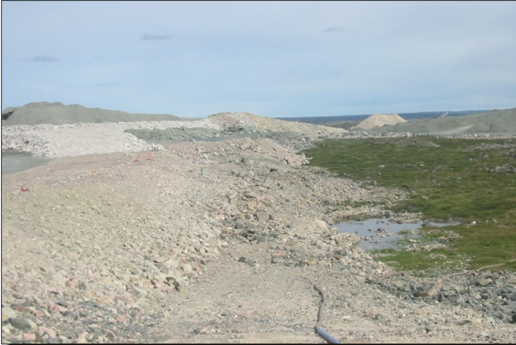
Photo C3 East Dam - Feature ED-1, ponded water at low area at downstream dam toe.
