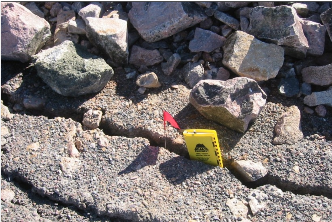
Photo B6 Feature DD-3 - Cracking in dyke filter.
