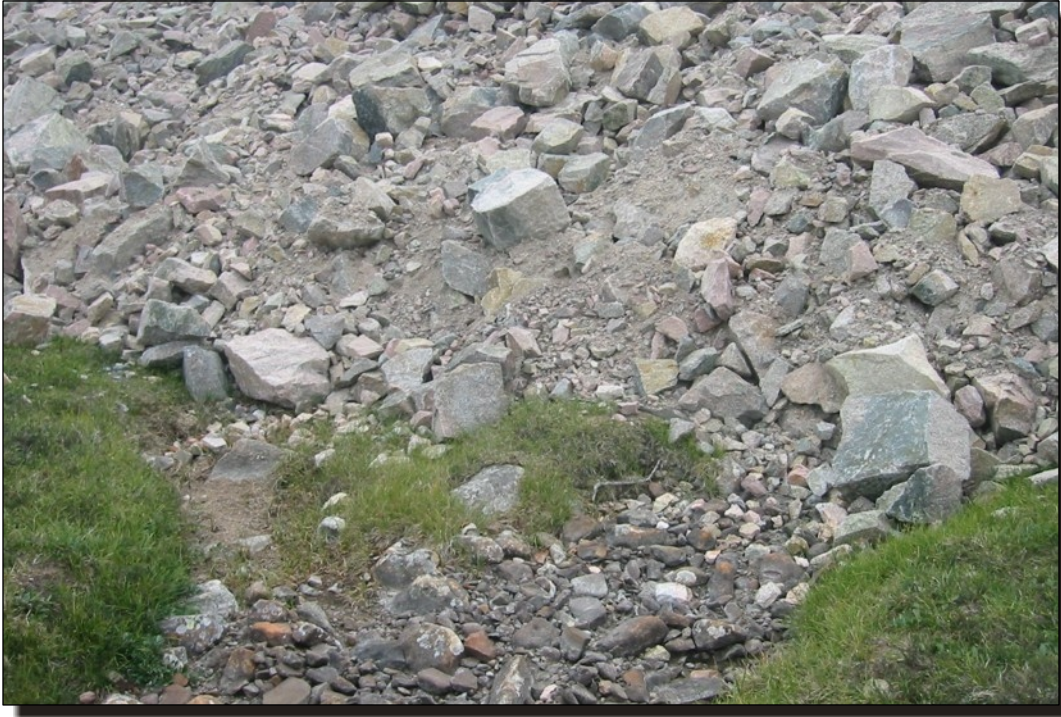
Photo I17 Feature C1-2, Damp area downstream of north berm. No seepage observed.
