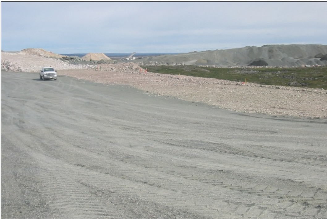
Photo C4 Dam Crest - 200 mm minus material over lined portion of dam, coarse PK in upstream shell.
