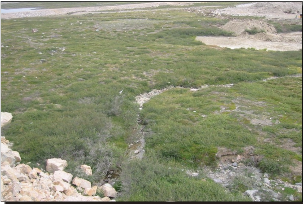
Photo I18 Feature C1-3, Ponded water in remnant stream channel below C1 channel cut off. No seepage apparent.
