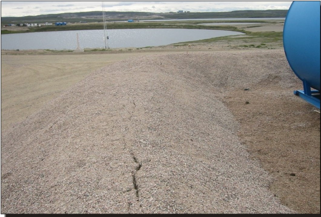
Photo F2 Airstrip tank farm - settlement cracks.
