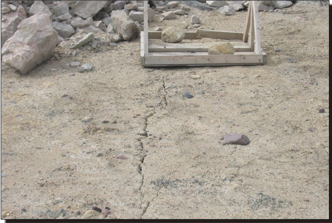
Photo E5 Landfill - surface crack.
