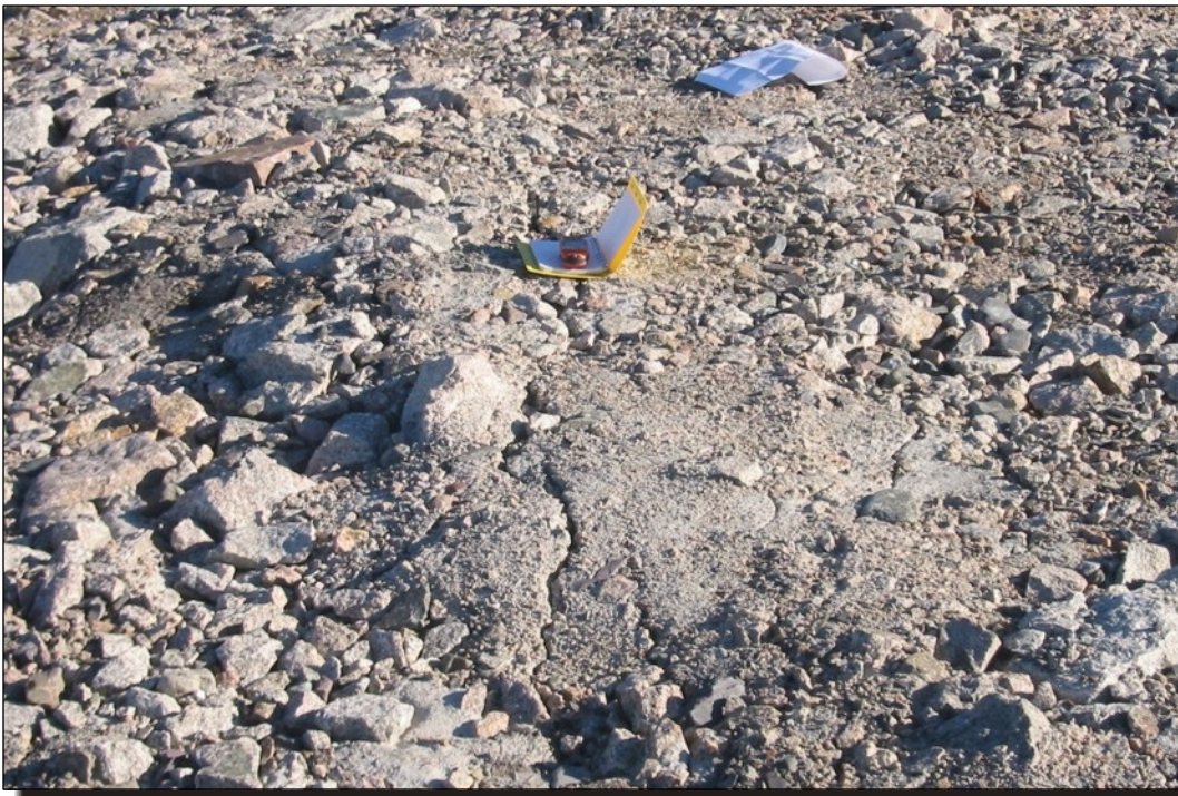
Photo A4 West Dam - Feature WD-1, isolated cracking in downstream shell.
