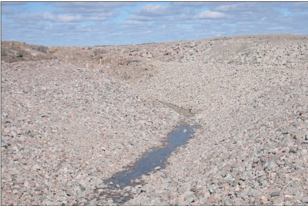
Photo I2 C1 Diversion - start of diversion channel - lined cut off.
