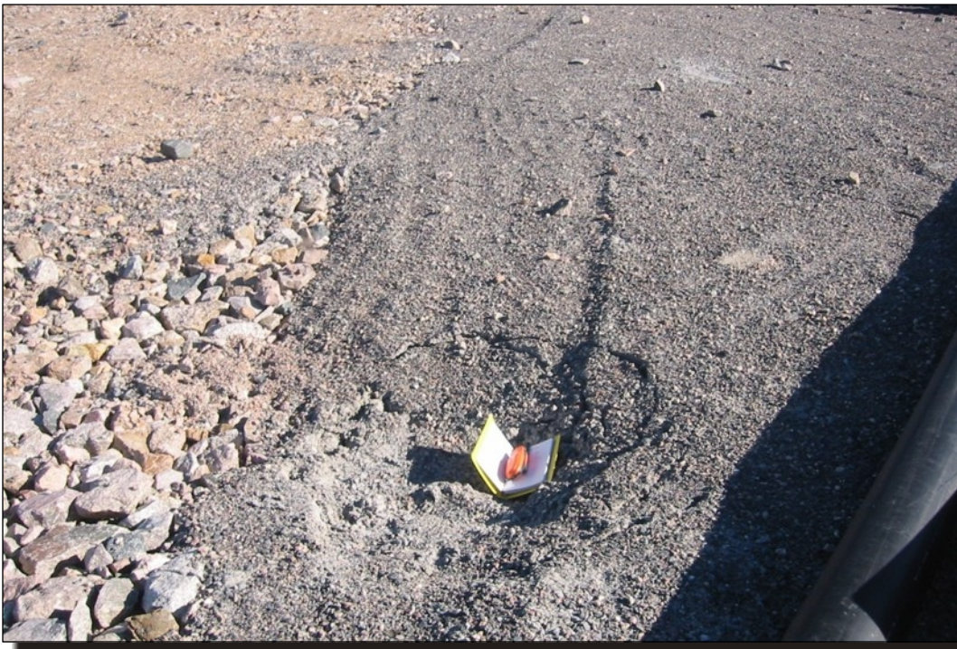
Photo B4 Feature DD-1 - Settlement.
