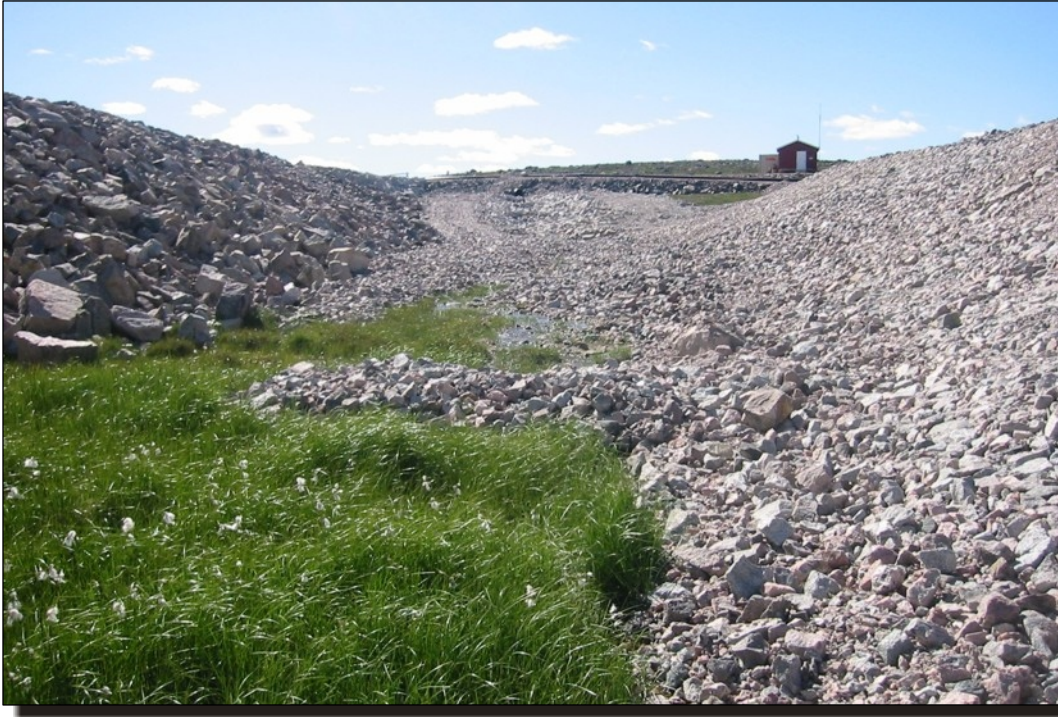
Photo I11 C1 Diversion - Reach C - water diversion berm.
