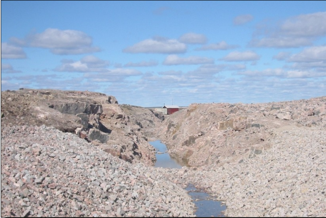
Photo I3 C1 Diversion - flow through reach A - bedrock cut.
