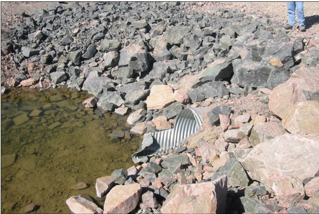
Photo I6 C1 Diversion - Culvert below Reach A - bent culvert end.
