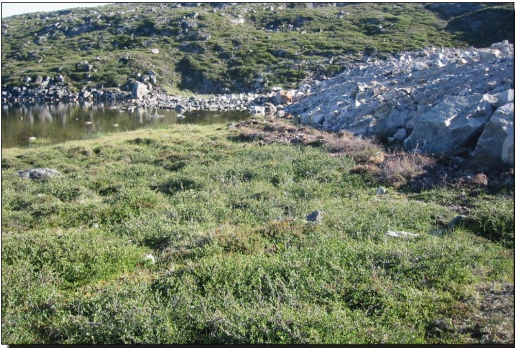
Photo A6 West Dam - Feature WD-3, wet area at downstream dam toe.
