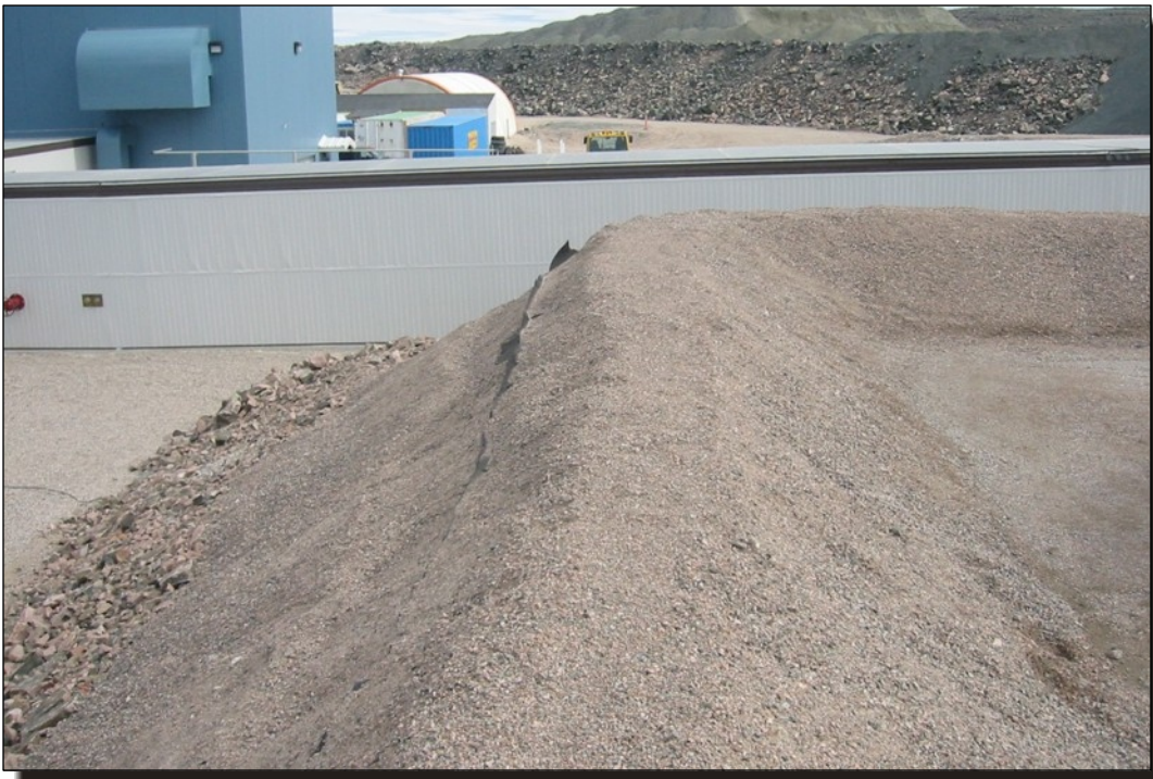
Photo G2 Generator tank farm - liner exposed.
