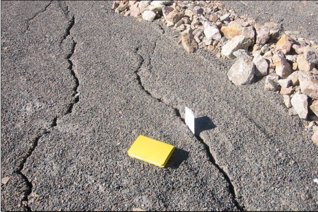
Photo B5 Feature DD-2 - Cracking in dyke filter.
