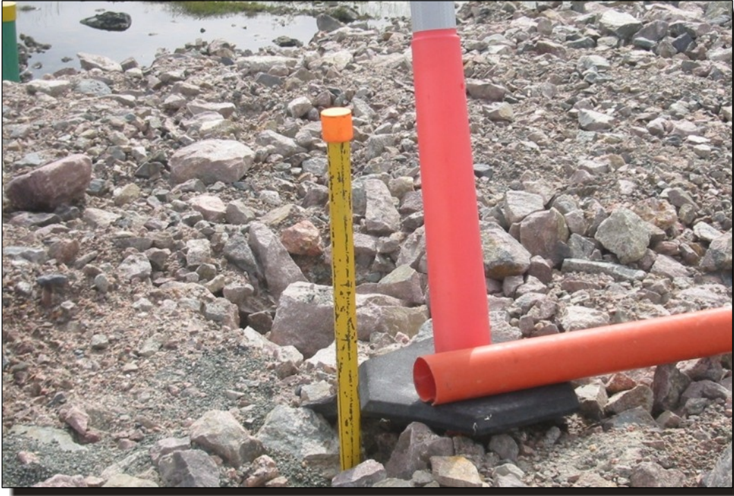
Photo C5 East Dam - Settlement monitoring point.
