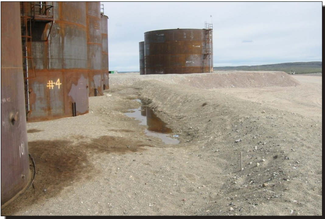
Photo D8 Tankfarm - Feature TF-3, ponded water in tankfarm containment area.
