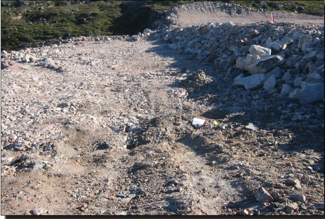
Photo A5 West Dam - Feature WD-2, voids in downstream shell.
