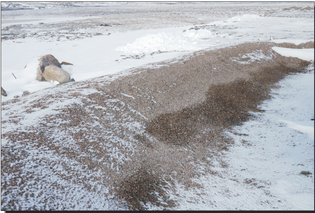
Photo H-2 Soil staining in Airstrip tank containment
