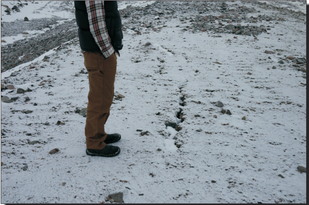
Photo E-7 Cracking noted in Reach C berm
