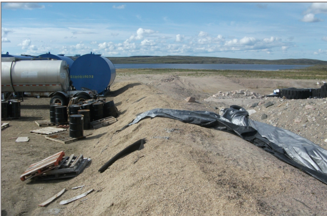
Photo K4: Exposed and damaged liner in center berm
