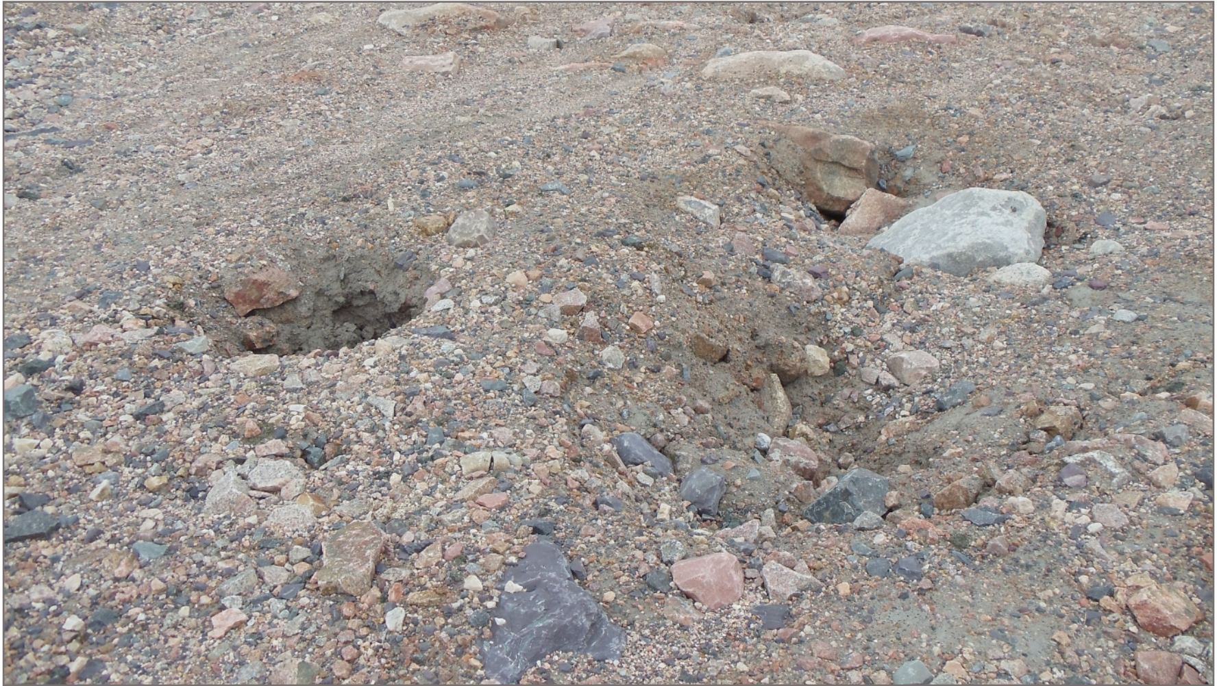
Photo L6: Minor settlement in waste pile 1; settlement is not a concern and does not impact waste rock pile performance
