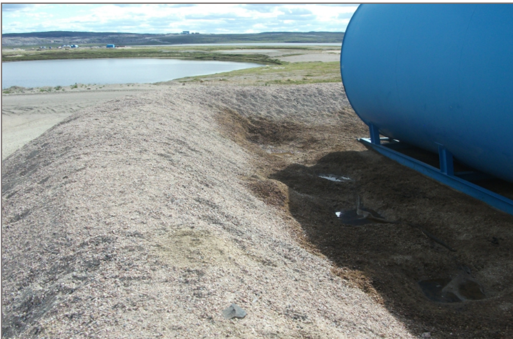
Photo I2: Staining on interior of containment area
