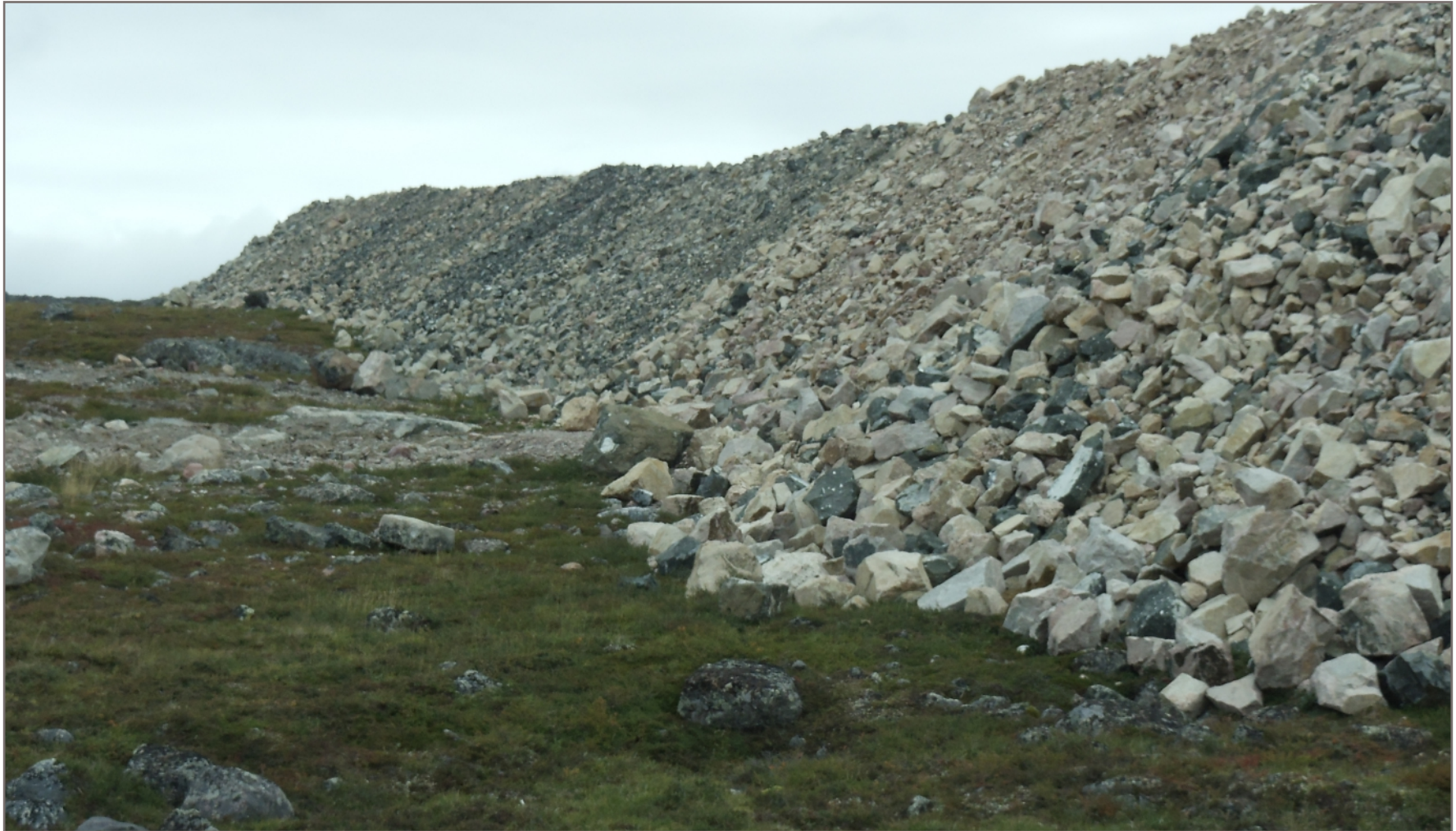
Photo L4: Waste Rock Dump 1 slope in good condition
