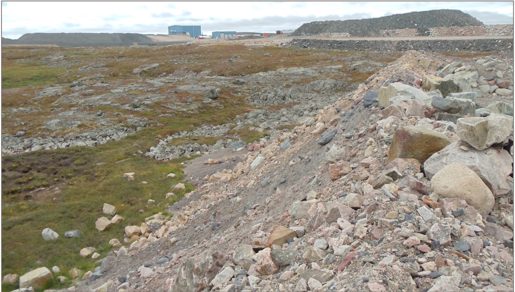
Photo L2: Till pile slope, note some sloughing of ice-rich material at toe; low grade and coarse PK stockpiles in background of photo
