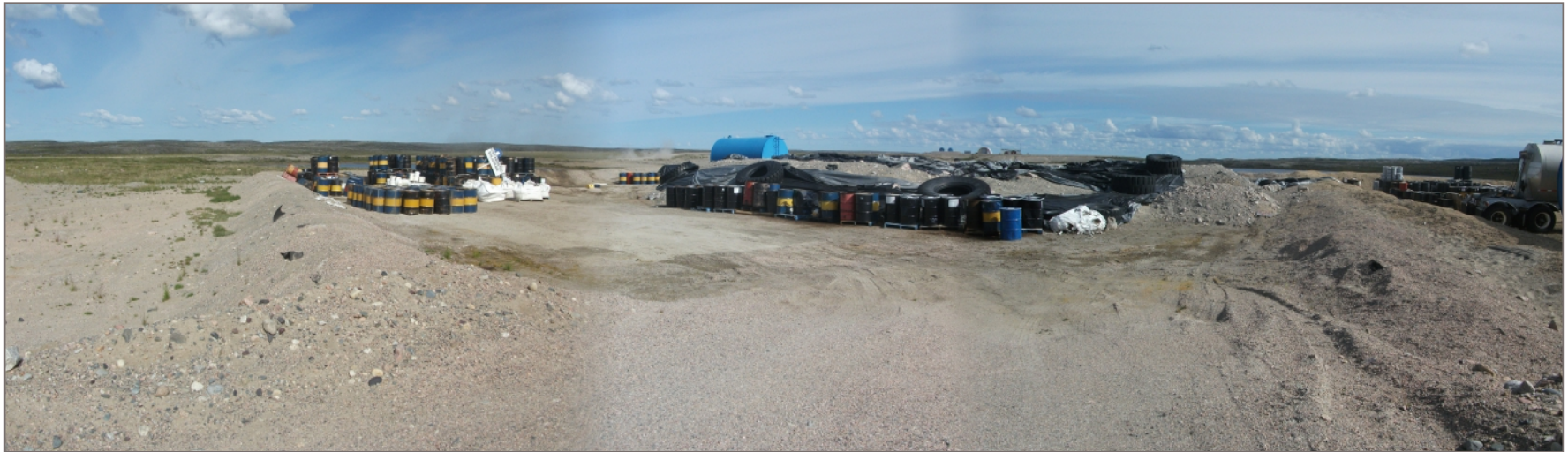
Photo K2: West cell from center berm location; note low spot in center berm in foreground of picture
