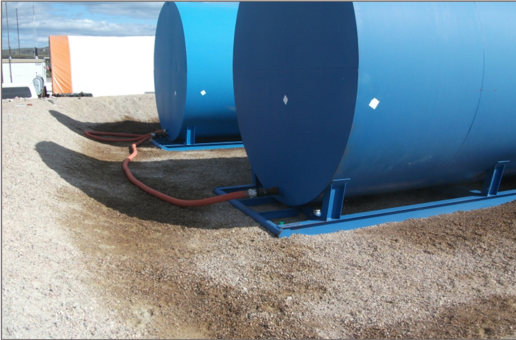
Photo I3: Staining on interior of containment area
