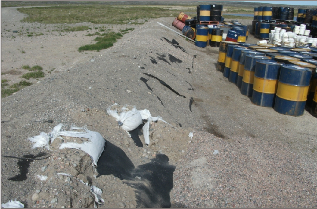
Photo K3: Liner damage in west cell on southwest berm
