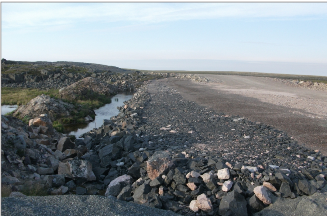
Photo C4: Upstream slope of dyke at south end of structure, no problems noted
