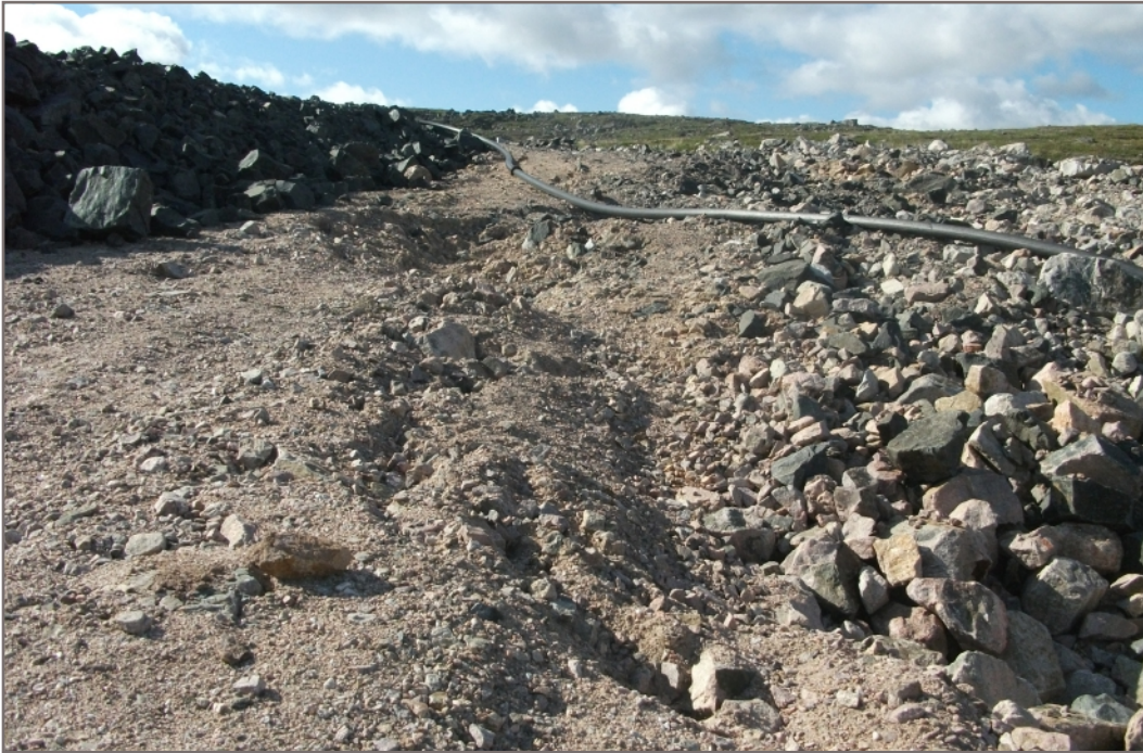
Photo B7: Tension cracking downstream of settlement area; condition appears unchanged from 2009, does not impact dam performance
