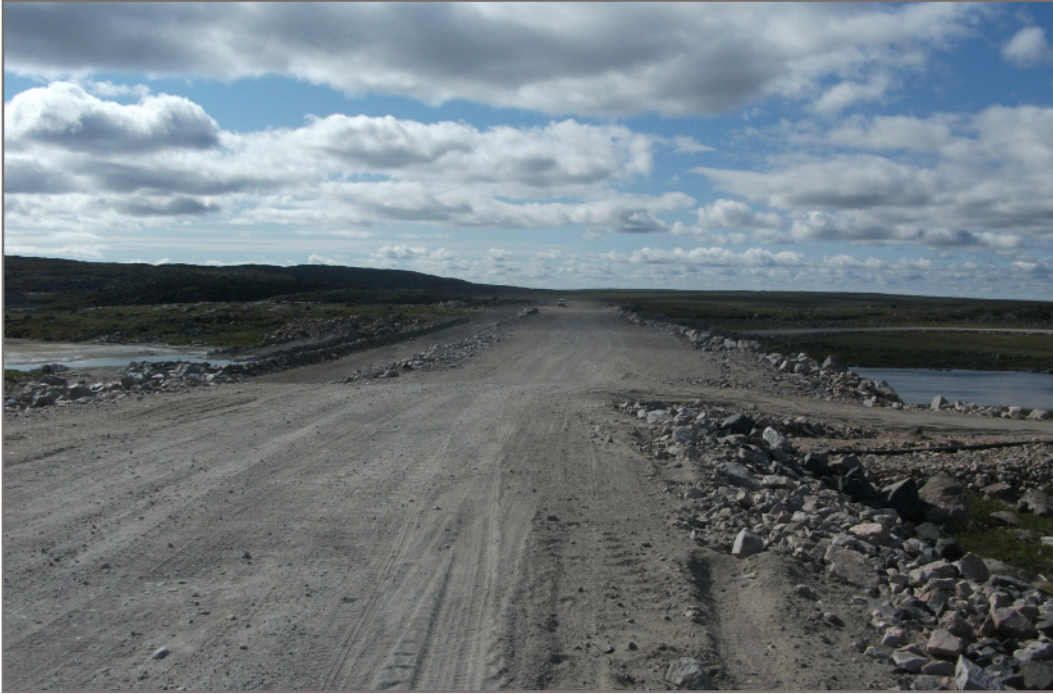
Photo C1: Divider Dyke A facing south; crest is in good condition with no problems noted
