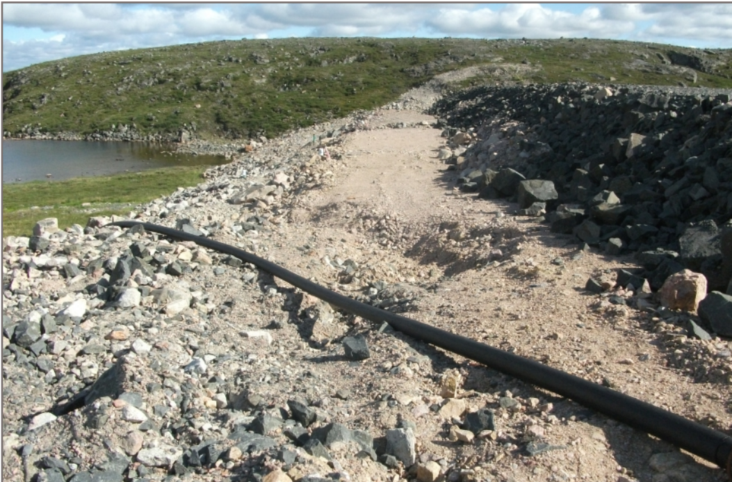
Photo B6: Settlement at south end of dam, on downstream slope; condition appears unchanged from 2009
