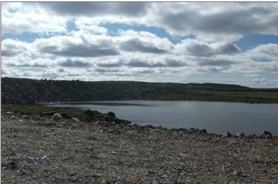
Photo C2: Downstream slope of divider is in good condition
