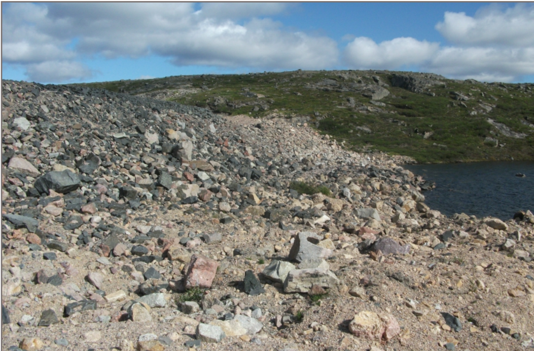
Photo B4: Upstream slope of dam in good condition
