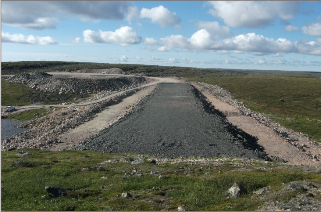
Photo B3: West dam looking south; dam crest in good condition with no problems noted
