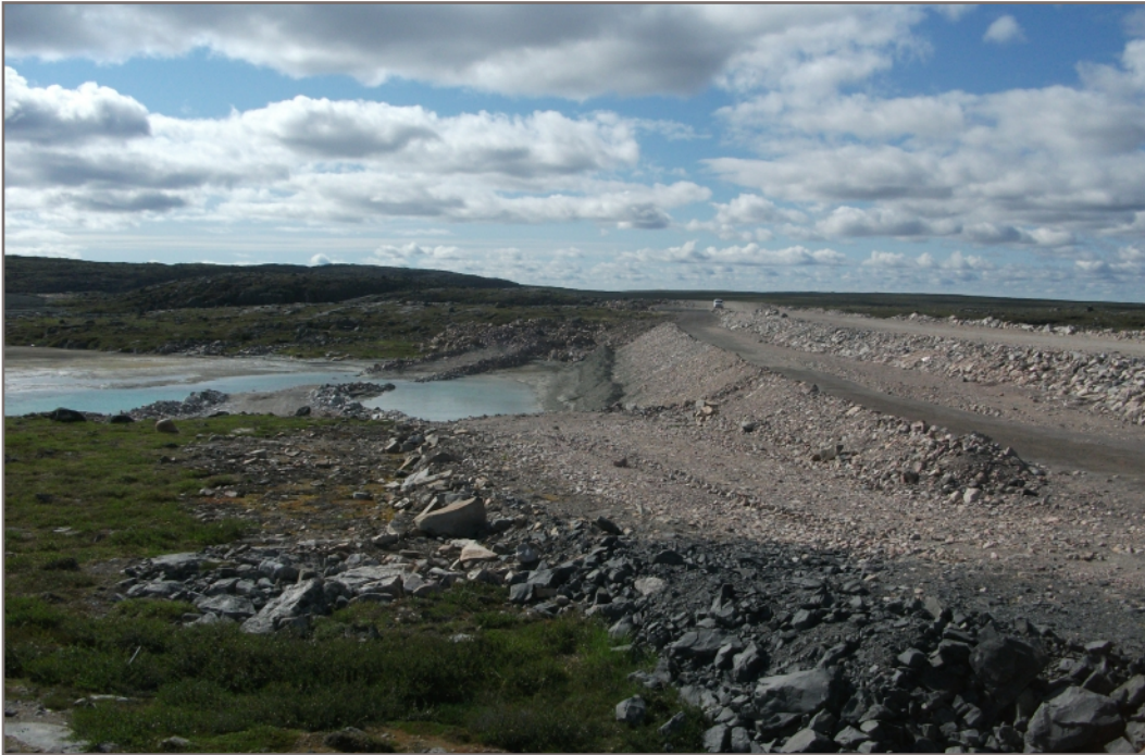
Photo C3: Upstream face of divider dyke; processed kimberlite placed on upstream slope to inhibit seepage through dyke
