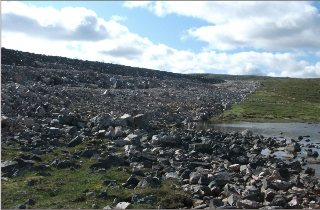
Photo B5: Downs slope of dam generally in good condition. Some settlement and tension cracking at south end of dam. Does not impact dam performance
