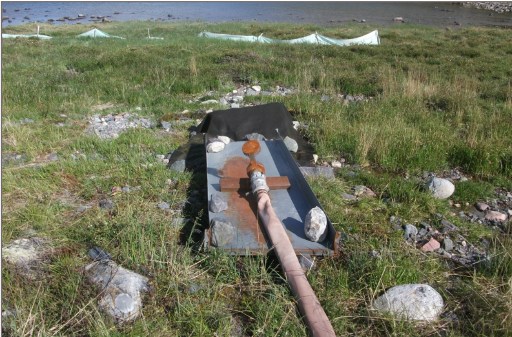
Photo B2: Energy dissipator at discharge location
