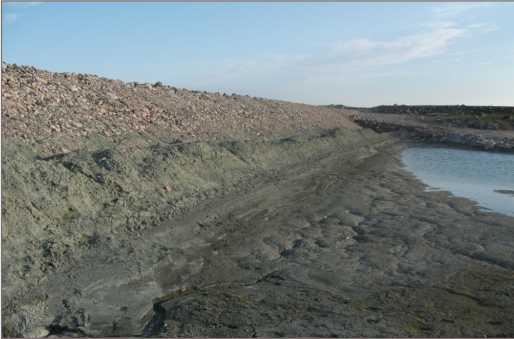
Photo C5: Processed kimberlite placed on upstream face of divider dyke
