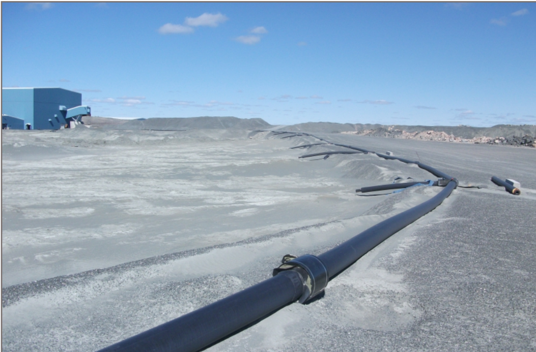
Photo D2: Processed kimberlite deposited on upstream face of dam
