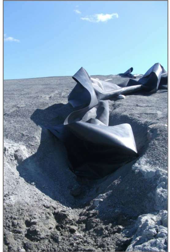
Photo E5: Localized erosion of processed kimberlite cover at discharge location; does not impact dam performance
