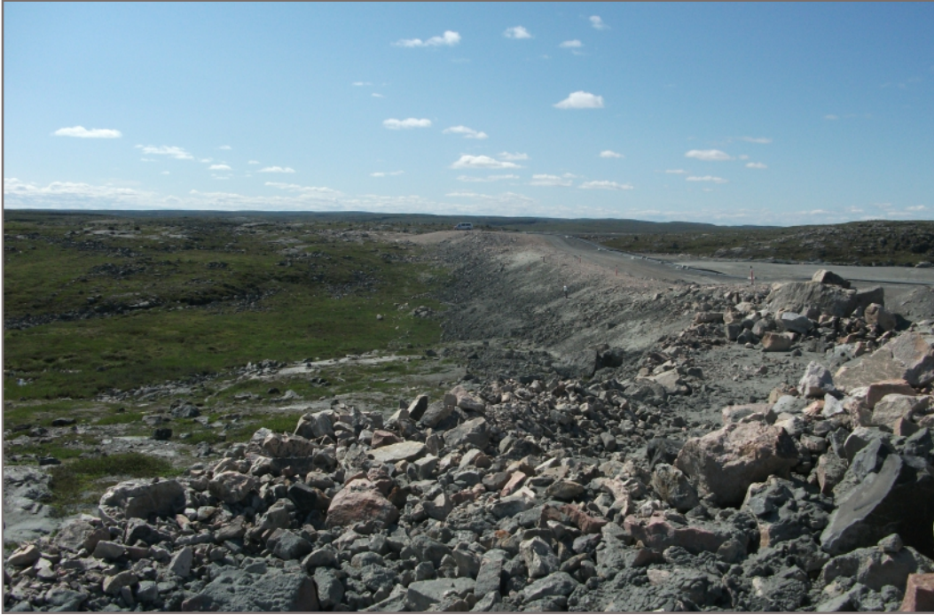
Photo E3: Downstream slope of dam is in good condition
