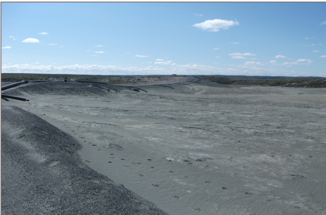
Photo E2: Processed kimberlite discharged on upstream face of dam
