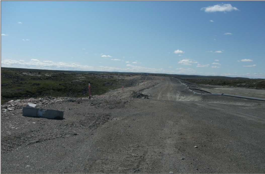
Photo E1: Southeast Dam crest facing southwest; crest is in good condition with no problems noted
