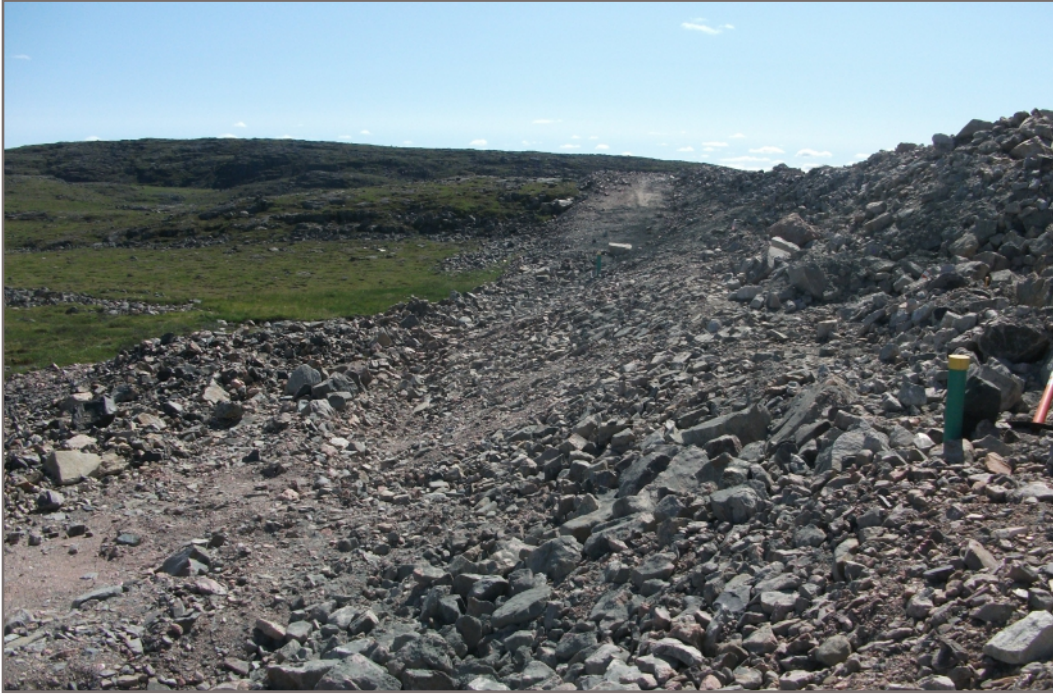
Photo D3: Downstream face of dam is in good condition
