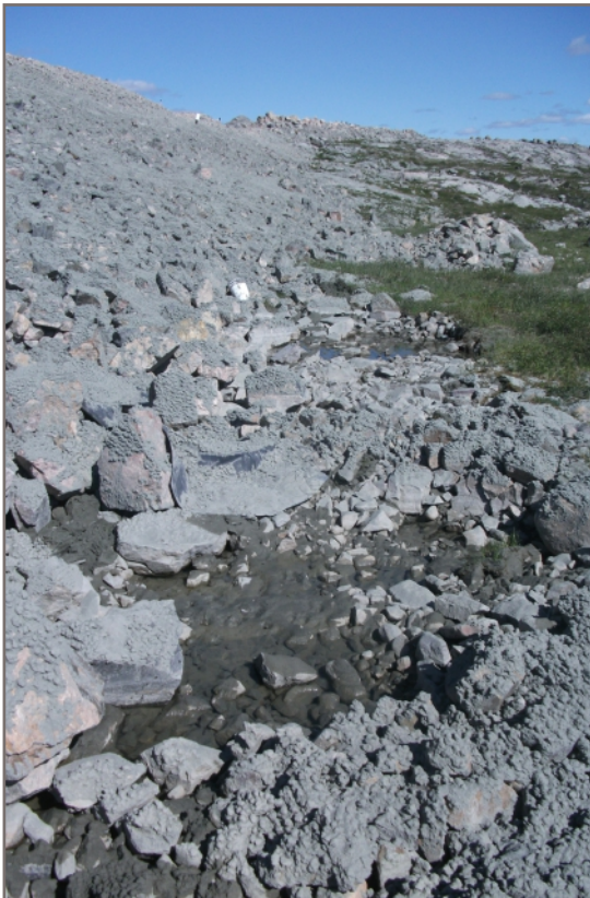
Photo E6: Ponded water adjacent to downstream toe; water collected in topographic lows and not seeping through dam
