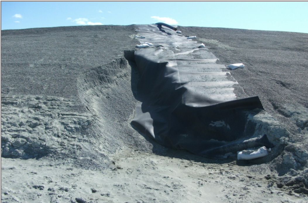
Photo E4: Localized erosion of processed kimberlite cover at discharge location; does not impact dam performance
