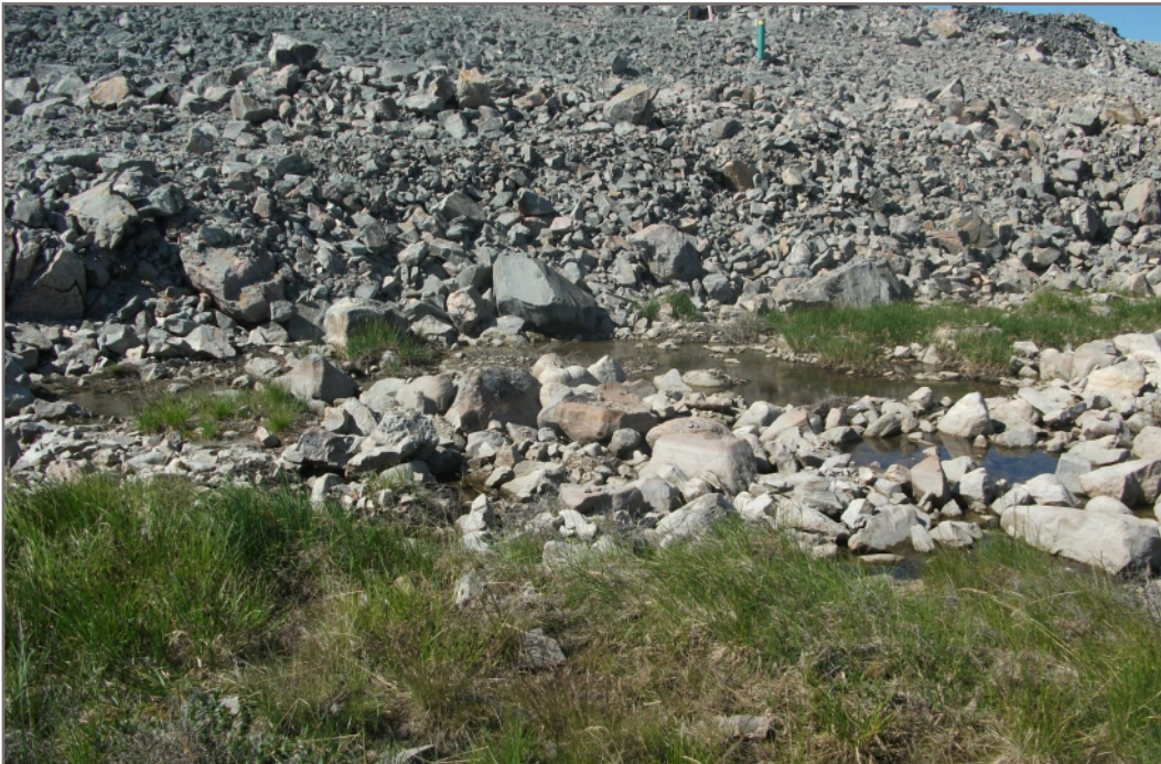
Photo D4: Standing water at downstream toe of dam; water is pooling in a topographic low and not seeping through dam
