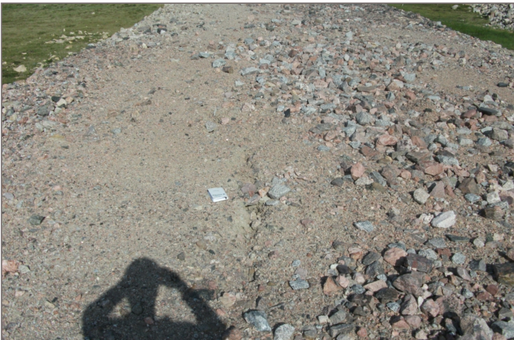
Photo F10: Longitudinal cracking in north berm (typical)
