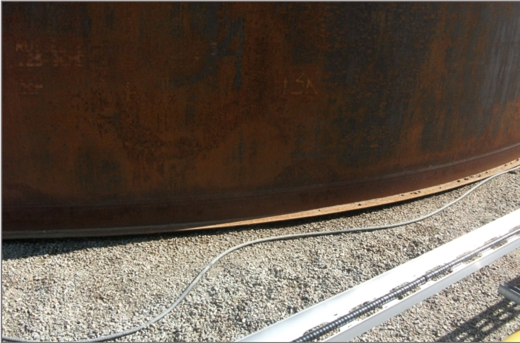
Photo G6: Gap under Tank 9 approximately 50 mm
