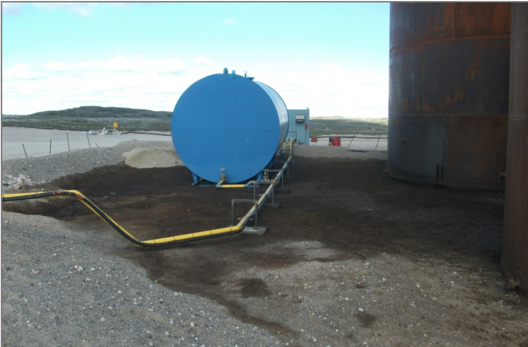
Photo G2: Significant staining in tankfarm area
