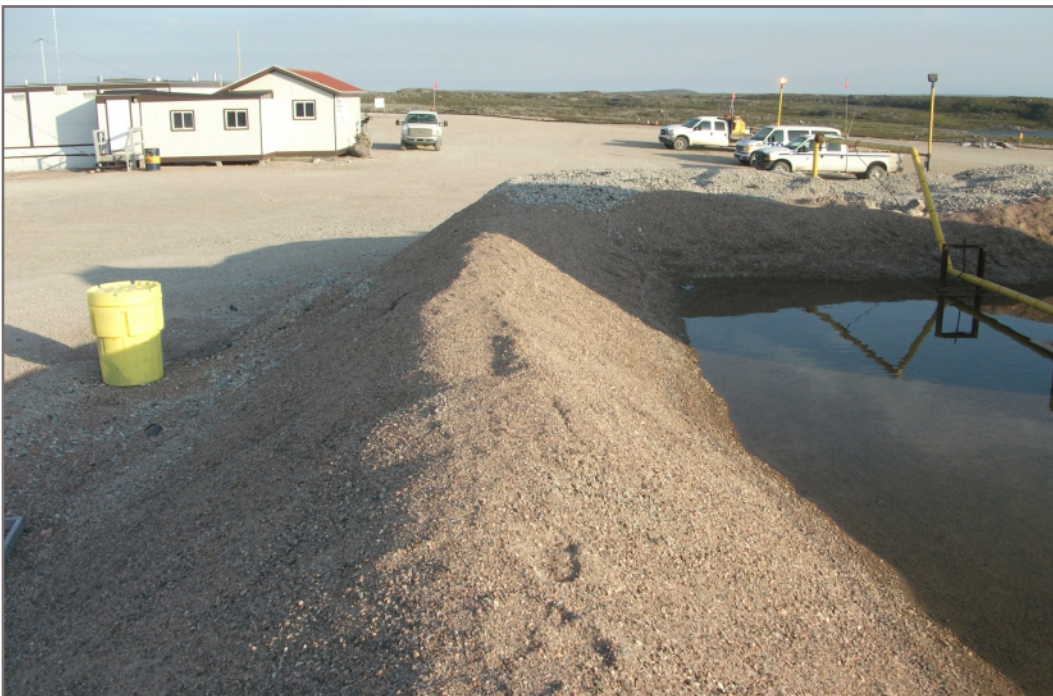
Photo H2: Low spot in generator tank berm
