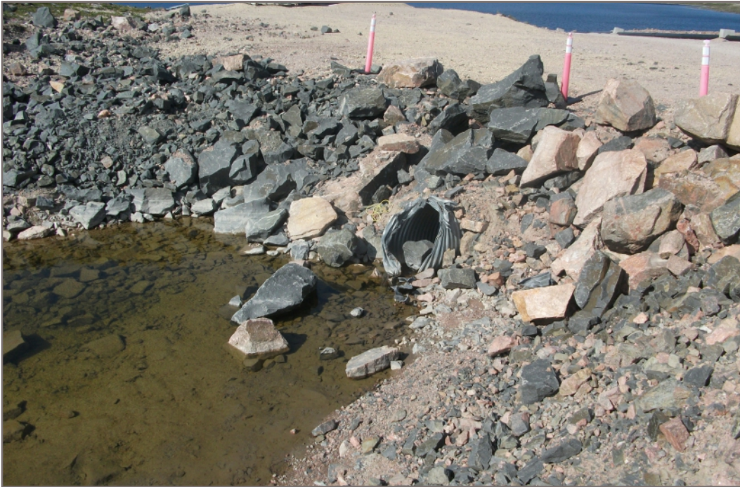
Photo F5: Carat Lake Road culvert inlet damaged; inlet appears to have been trimmed since 2009 to better facilitate culvert flow
