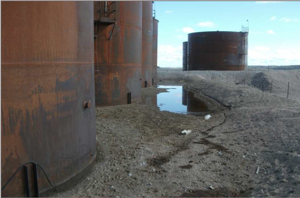
Photo G3: Water collected in northern portion of Phase 1 Tank Farm; low berm near tie-in with Phase 2 Tank Farm
