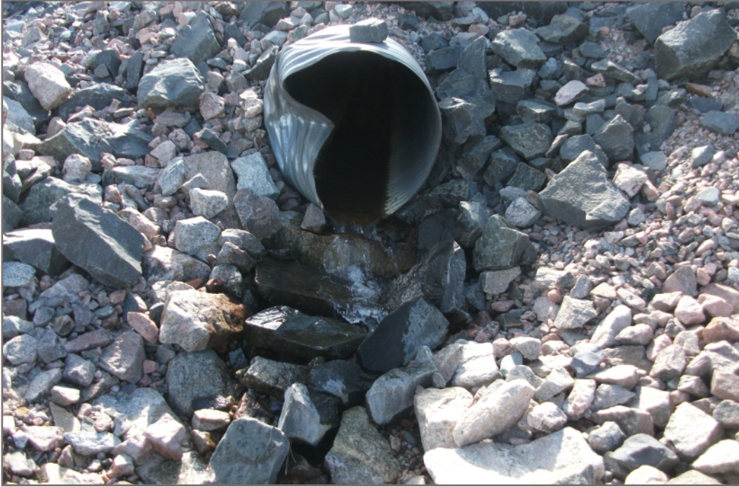
Photo F7: Culvert outlet; condition unchanged from 2009 inspection
