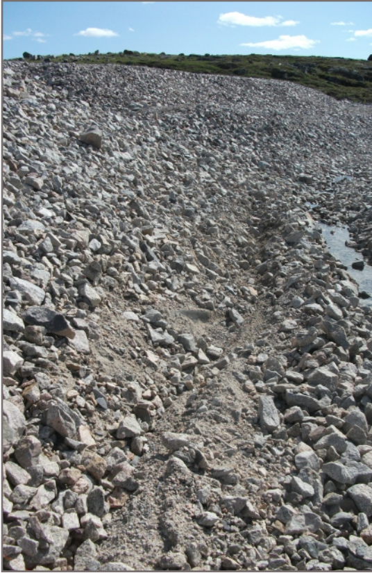
Photo F3: Sloughing of erosion protection at north end of Reach A
