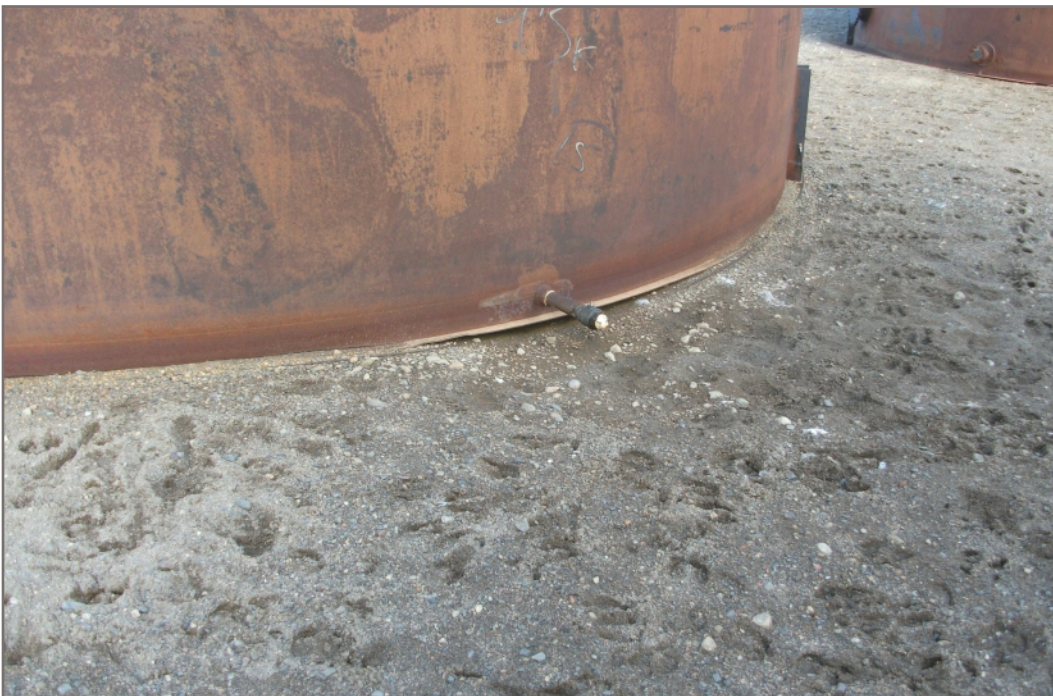
Photo G4: Gap under Tank 4 approximately 50 mm
