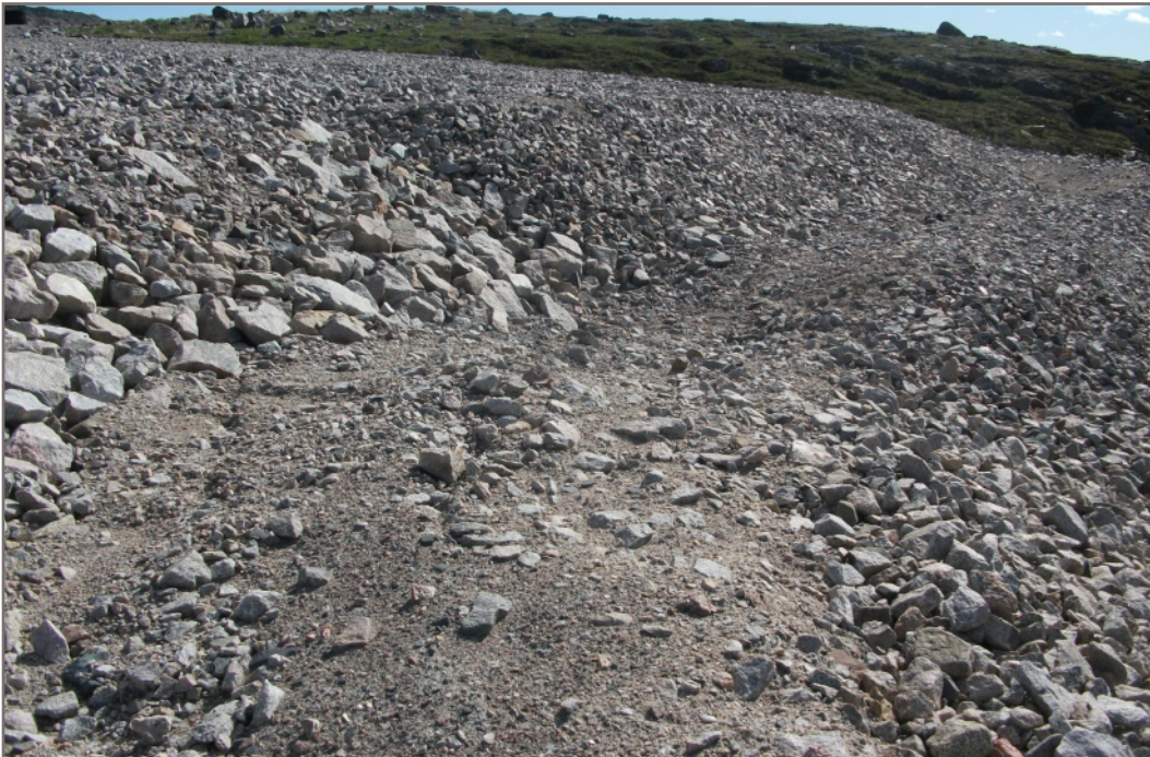
Photo F2: Settlement and tension cracking in inlet fill pad; area appears to have self healed from 2009 inspection
