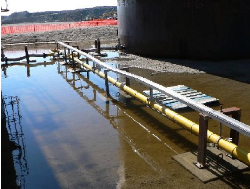
Figure 10: Main Tank Farm transfer Pipelines and pooling Water in the Containment
