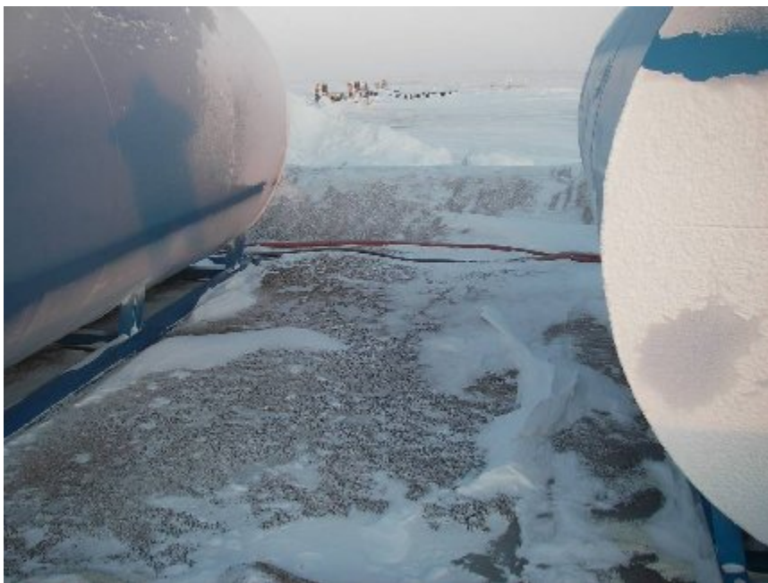
Figure 11: Airstrip Tank Farm showing the discharge hose and contaminated secondary berm liner
