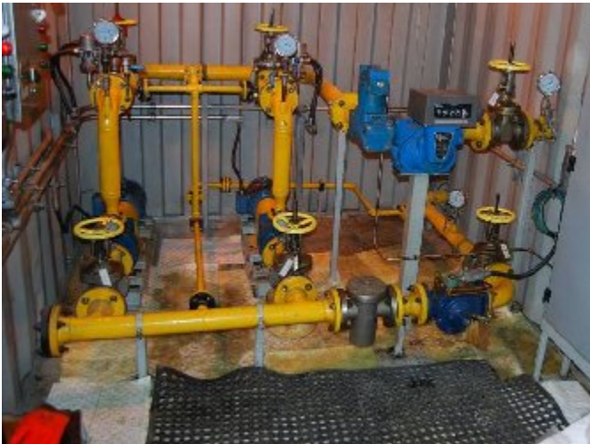
Figure 12: August 2008 leakage from the Pumps in the Fuel transfer Pump Station
