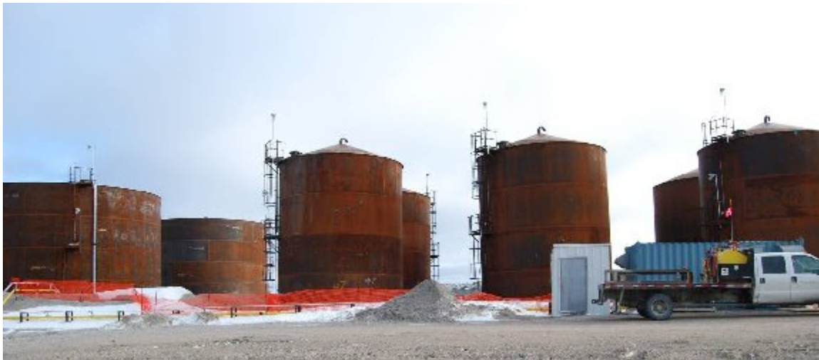
Figure 3: Photograph of the Main Tank Farm showing the large and small bulk Fuel Tanks & Fuel transfer Pump Station
