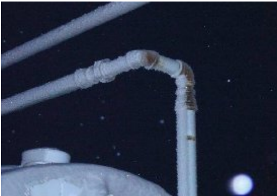
Figure 9: The horizontal 90 degree Swivel on the Truck Shop Tank
