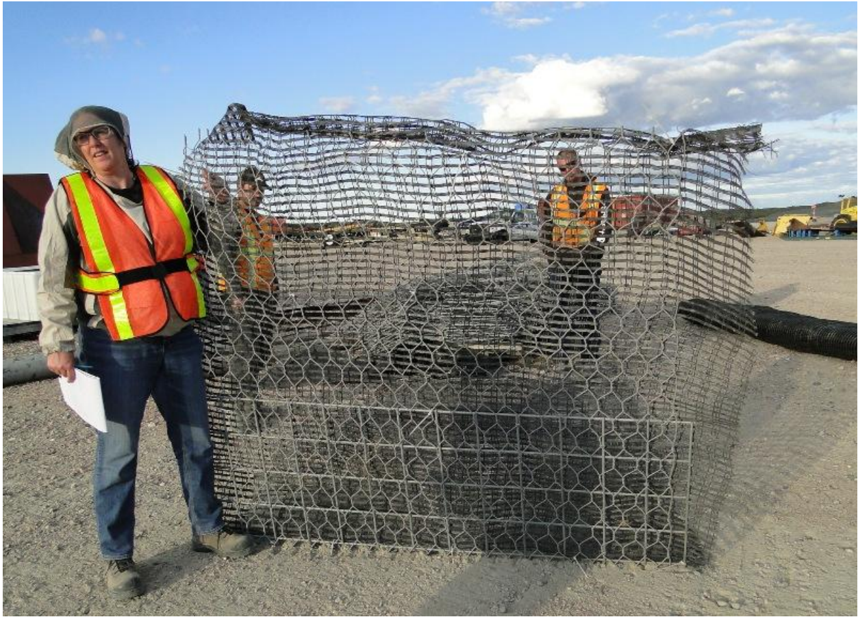
Figure 9. Proposed mitigation measure: windblock/silt fence to be added to tire berms.
