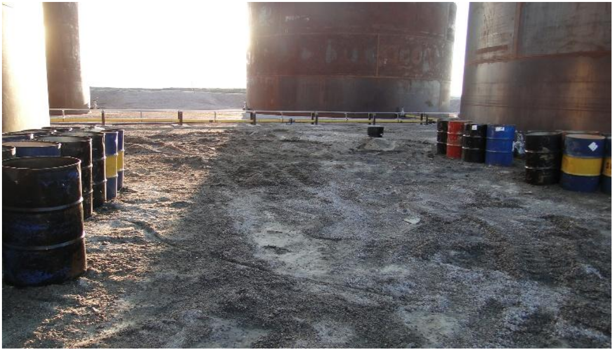
Figure 14. Contaminated material and barrels of contaminated water from oil spill (12-121).
