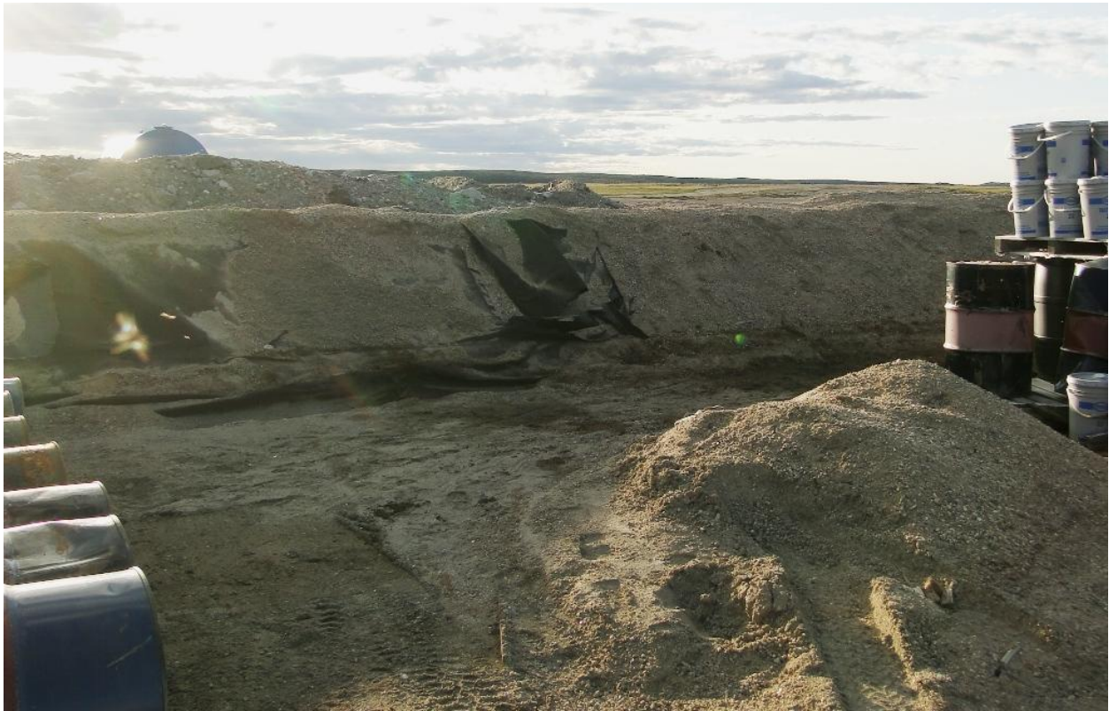
Figure 12. Liner of HWTa is exposed and integrity in doubt (scheduled for replacement this year).
