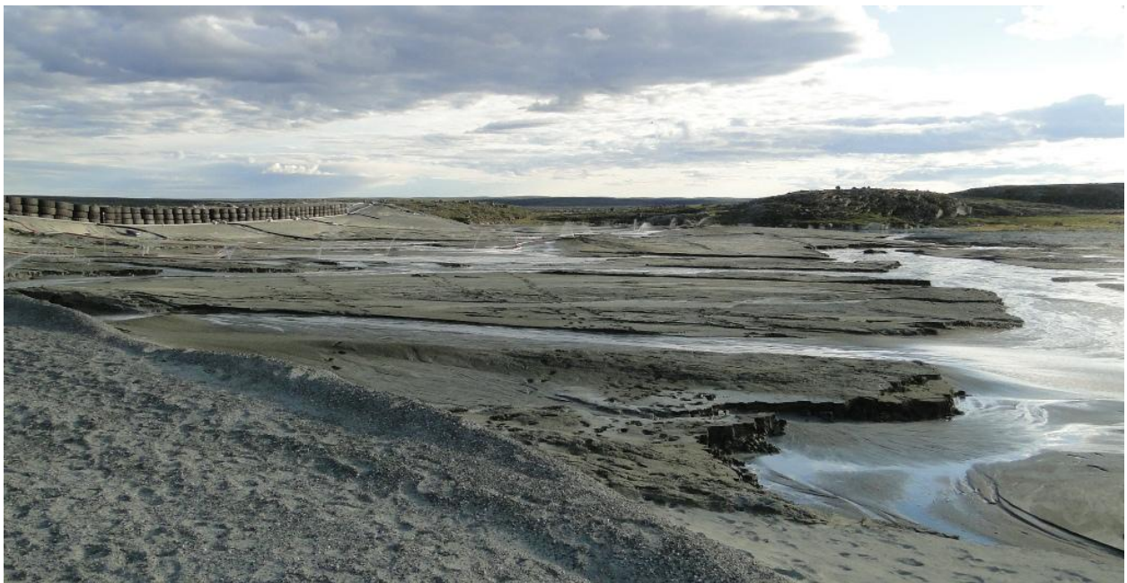
Figure 8. PKCA with new mitigation measures: Tire berm on up-wind side, sprinklers cycling water from Cell B/C to wet the FPK.
