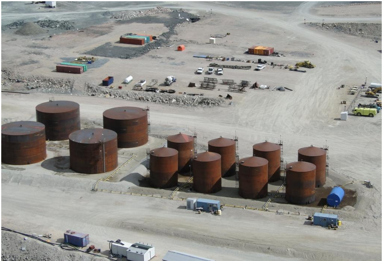
Figure 13. Legacy and contemporary contamination is present in many of the existing berms. This creates the need to constantly manage contaminated water.
