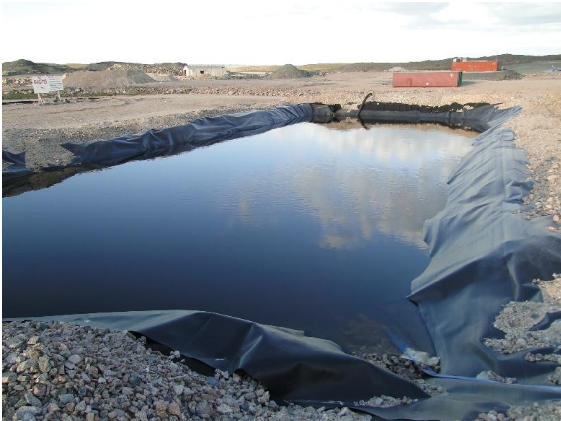
Figure 17. Water treated by the Oztek unit which now meets discharge criteria.
