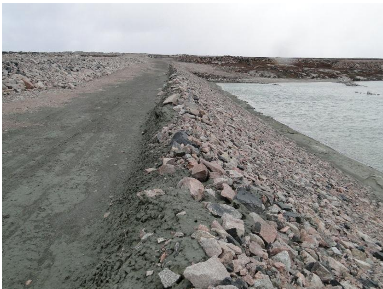
Figure 6. FPK pushing through east wall of Divider Dyke A.
