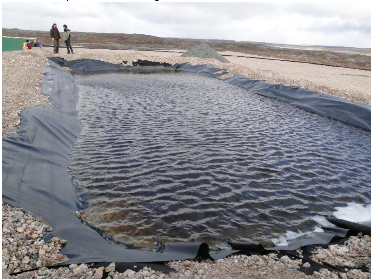
Figure 3. Oztek berm should be pumped out to protect the liner.
