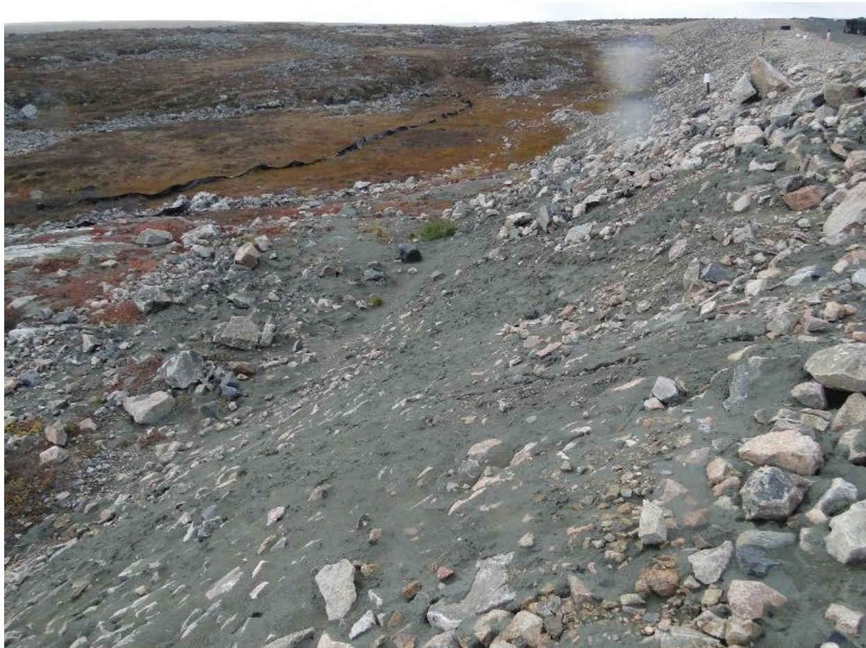
Figure 5. FPK from last winter still remains on the outside slope of the SE dam.
