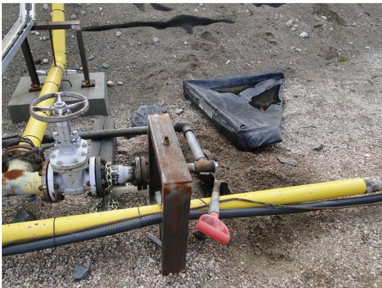
Figure 10. Leakage occurred behind the FTA; contaminated materials not picked up.
