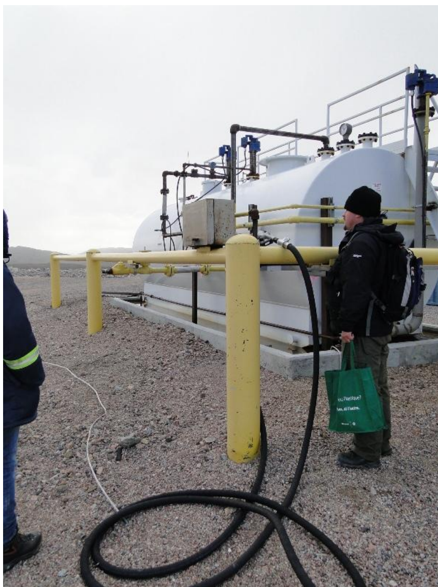
Figure 12. Fuel tank at Emulsion Plant - hose in 'on' position, berm 1/2 full of water.
