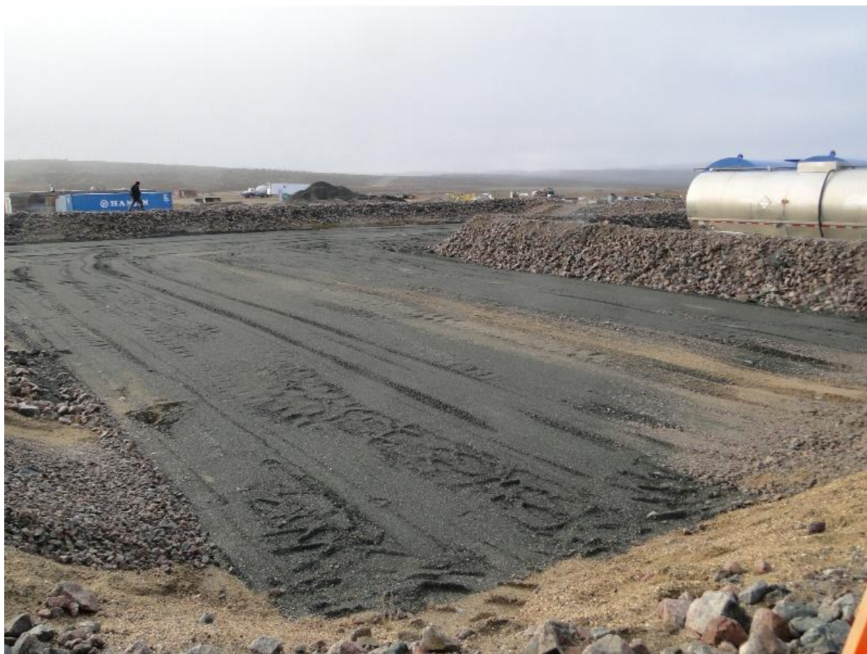
Figure 2. East cell of HWTa, ready for the new liner.
