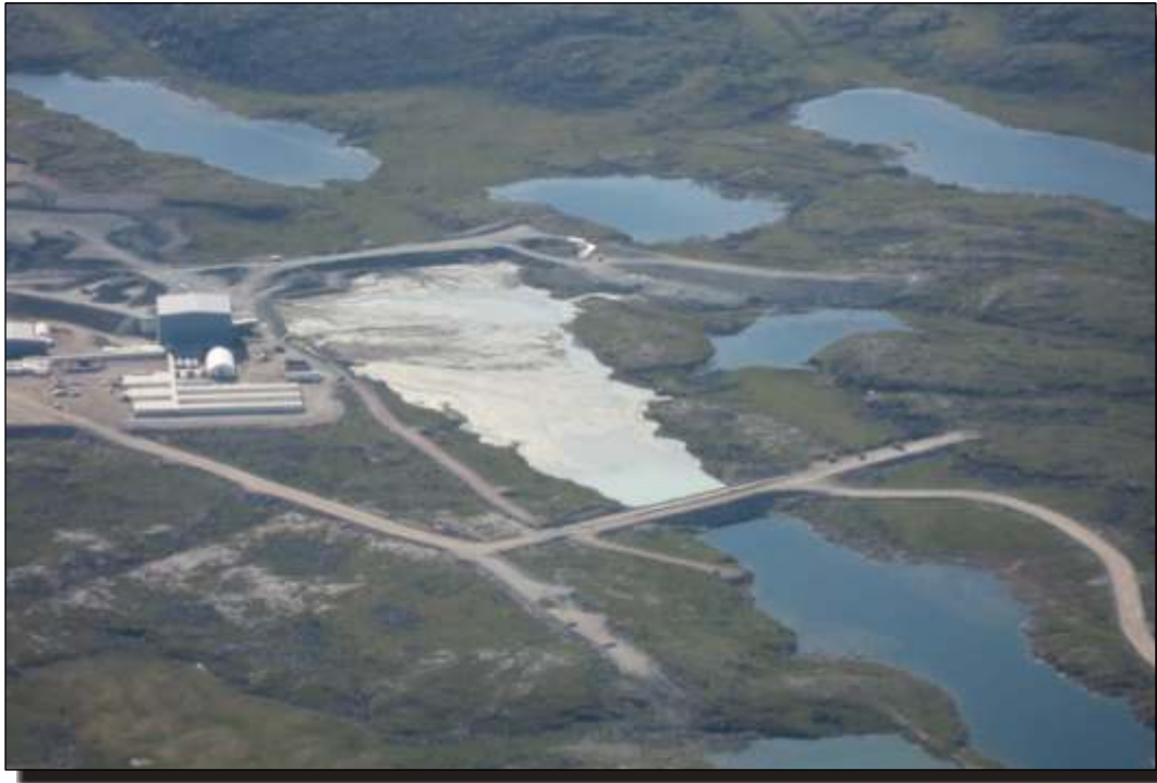
Photo C.1 PKCA, East Dam, Southeast Dam, Divider Dyke, looking east.
