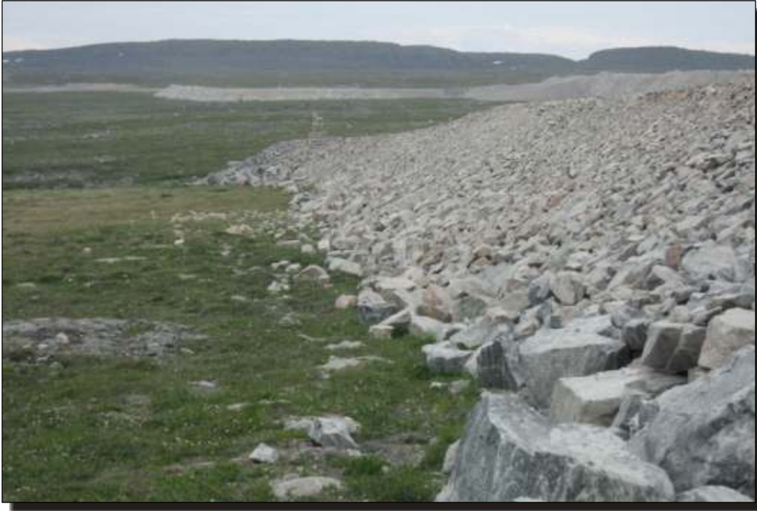
Photo H.17 C1 Diversion - Downstream north berm.
