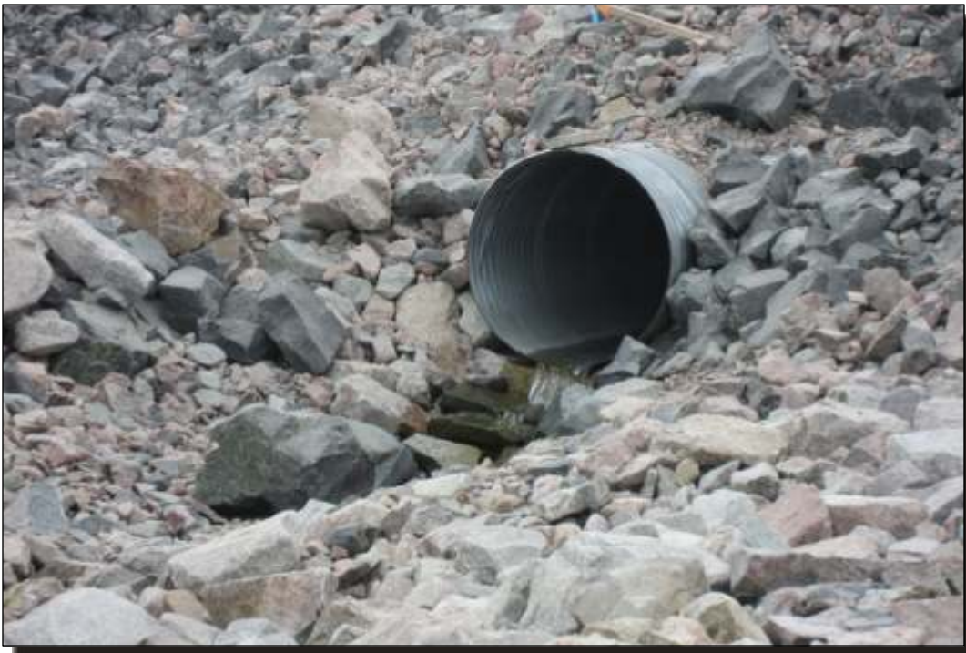
Photo H.8 C1 Diversion Channel - Reach A: Culvert outlet. Low water flow.
