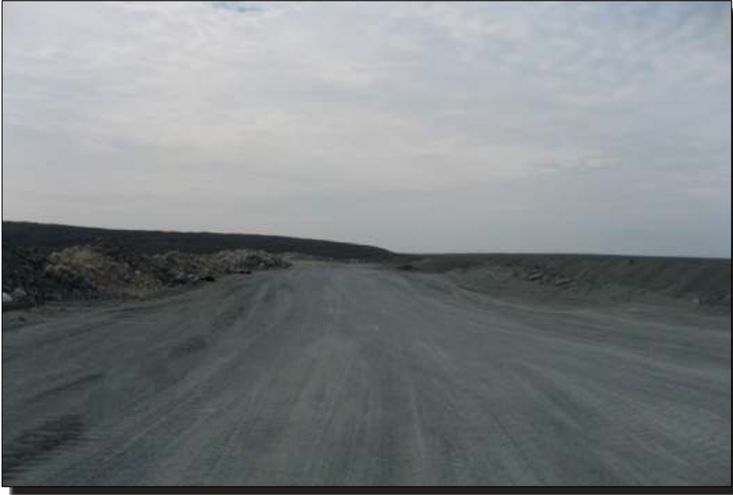
Photo C.6 East Dam: Dam crest.
