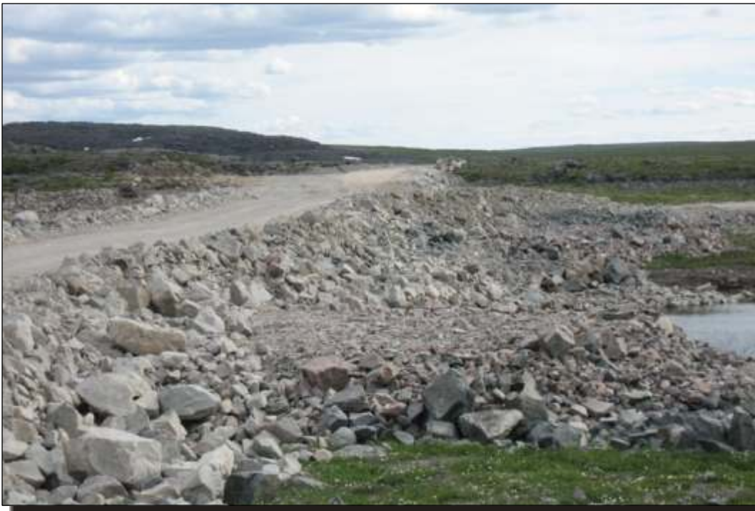
Photo B.4 Divider Dyke A: Downstream slope. Run of mine.
