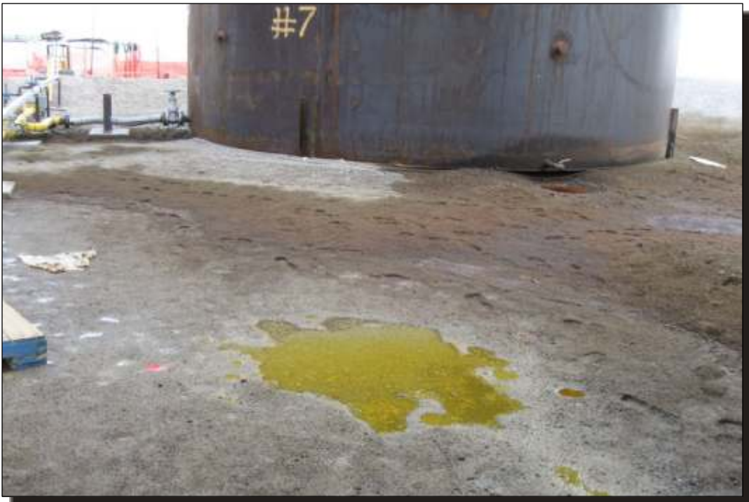
Photo D.4 Phase 1 Tankfarm: Pond with sheen on it between Tank 7 and Tank 8.
