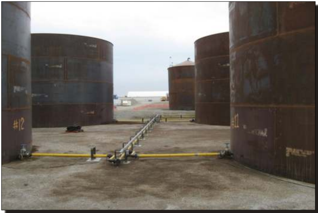
Photo D.10 Phase 2 Tankfarm: Looking south between the tanks.
