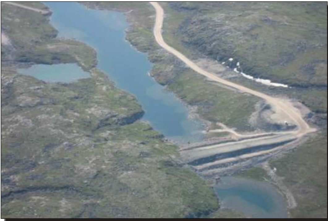
Photo A.2 West Dam: Downstream slope, looking east.
