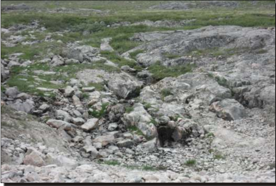
Photo H.1 C1 Diversion Channel - Inlet of C1 Channel: Minimal inflow to channel.
