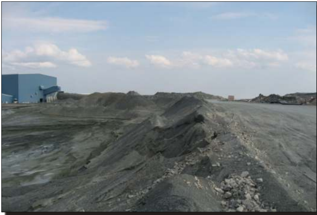
Photo C.2 East Dam: Upstream slope, looking north.
