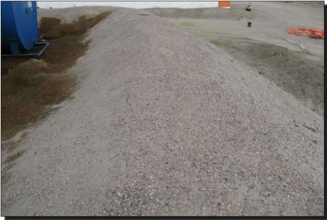
Photo F.6 Airstrip Fuel Tank: Containment Berm Crest.
