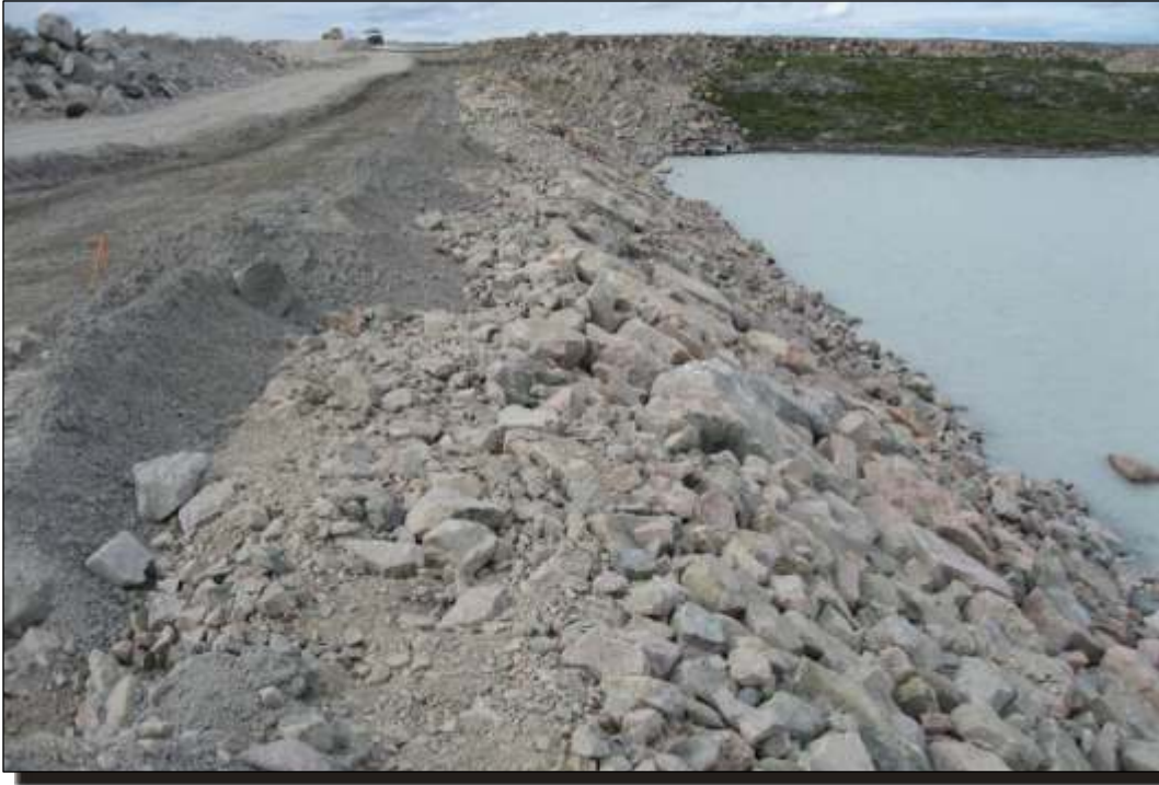
Photo B.3 Divider Dyke A: Upstream slope. Rip-rap, turbid water in Cell A.
