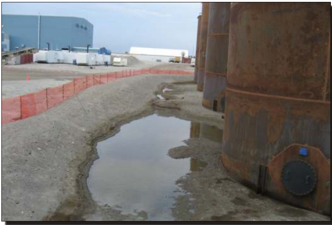
Photo D.5 Phase 1 Tankfarm: Pond along east side of tankfarm.
