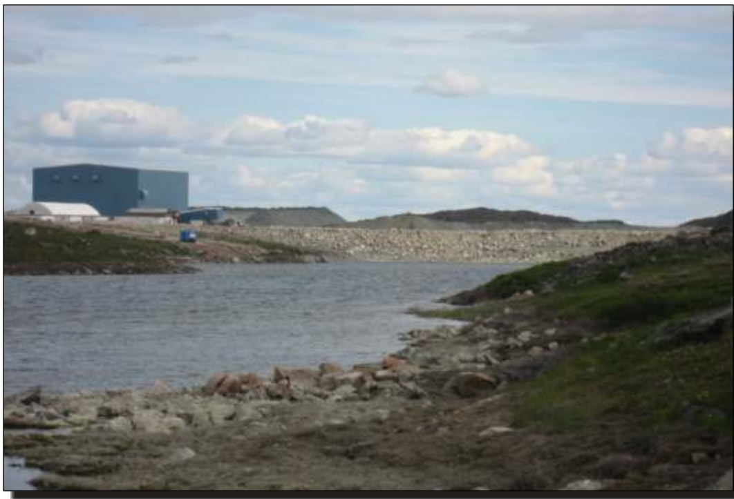
Photo B.2 Divider Dyke A: Downstream side, looking east across Cell B.
