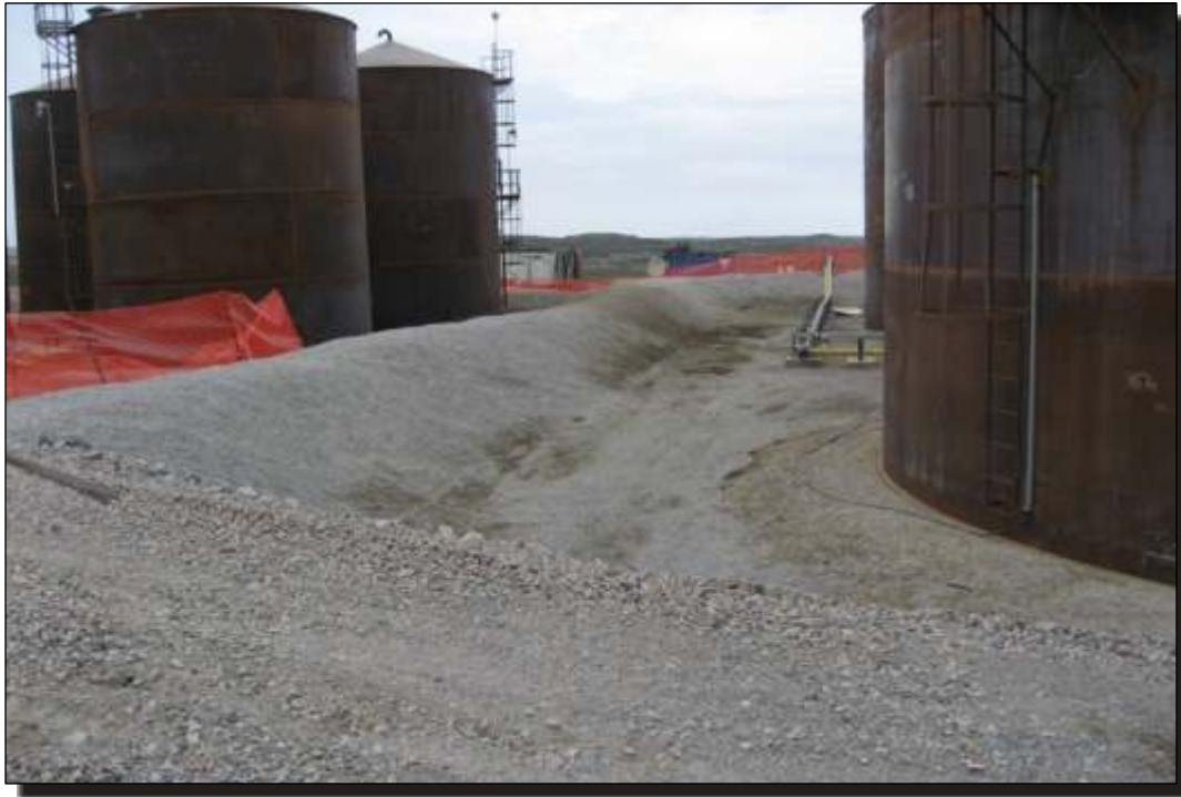
Photo D.11 Phase 2 Tankfarm: South berm, looking west.
