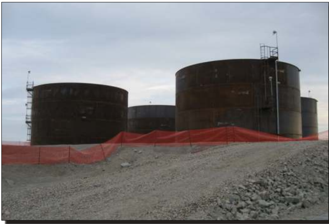
Photo D.8 Phase 2 Tankfarm: Four 1,500,000 litre tanks, looking north.
