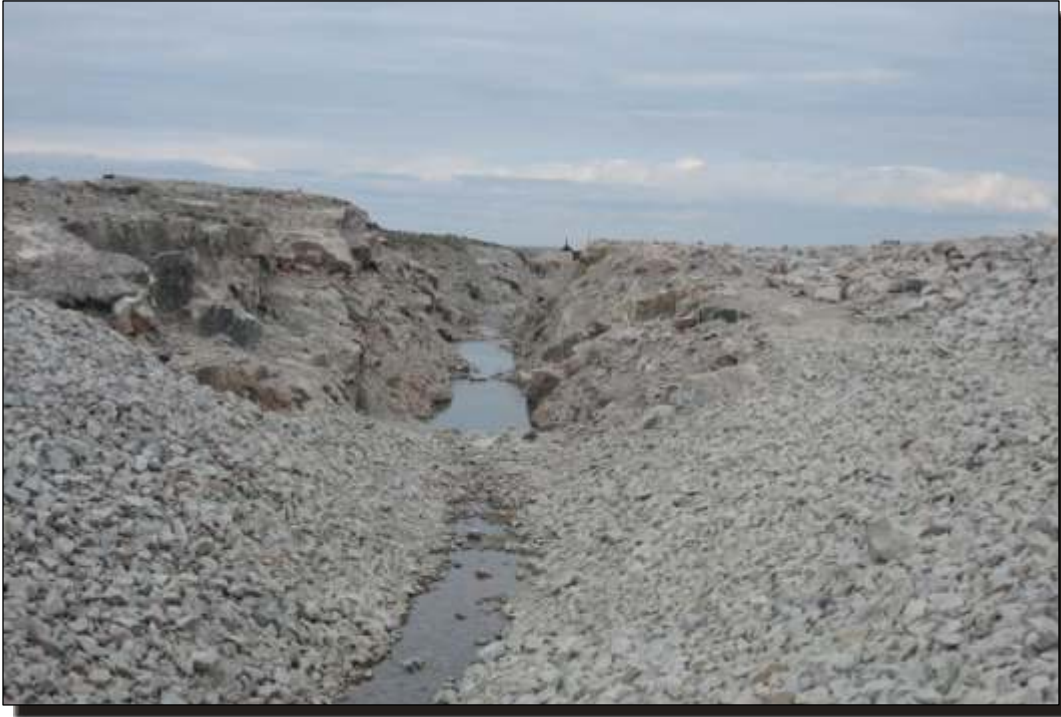
Photo H.5 C1 Diversion Channel - Reach A: Lower reach.
