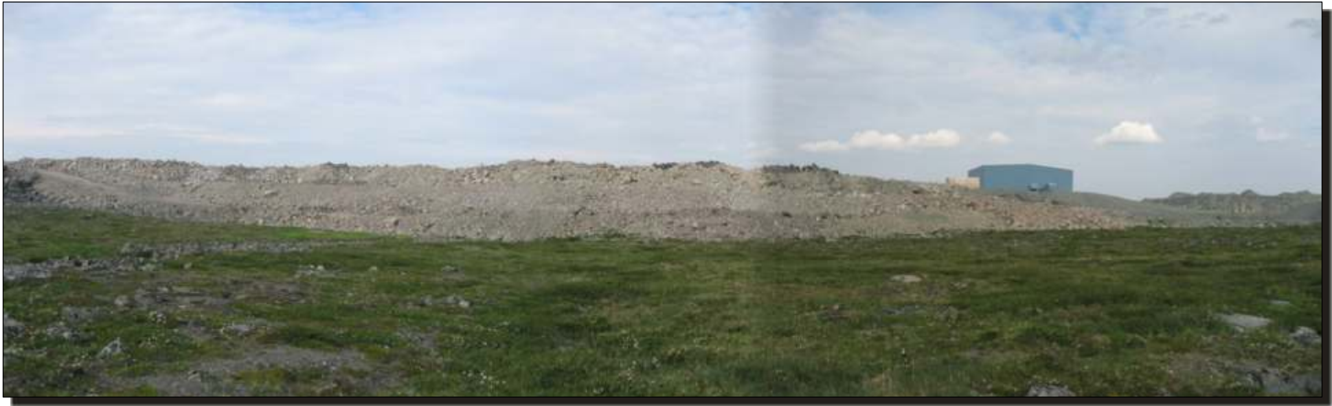
Photo C.3 East Dam: Downstream slope, looking west.
