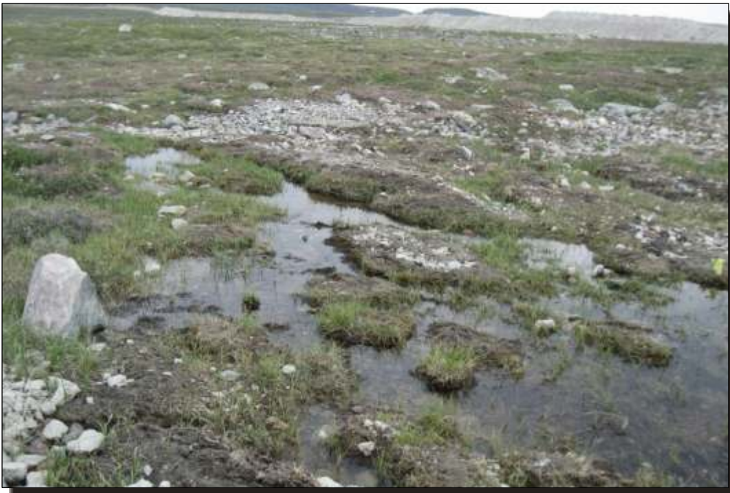
Photo H.14 C1 Diversion Channel - Reach C: Outlet. Ponded water.
