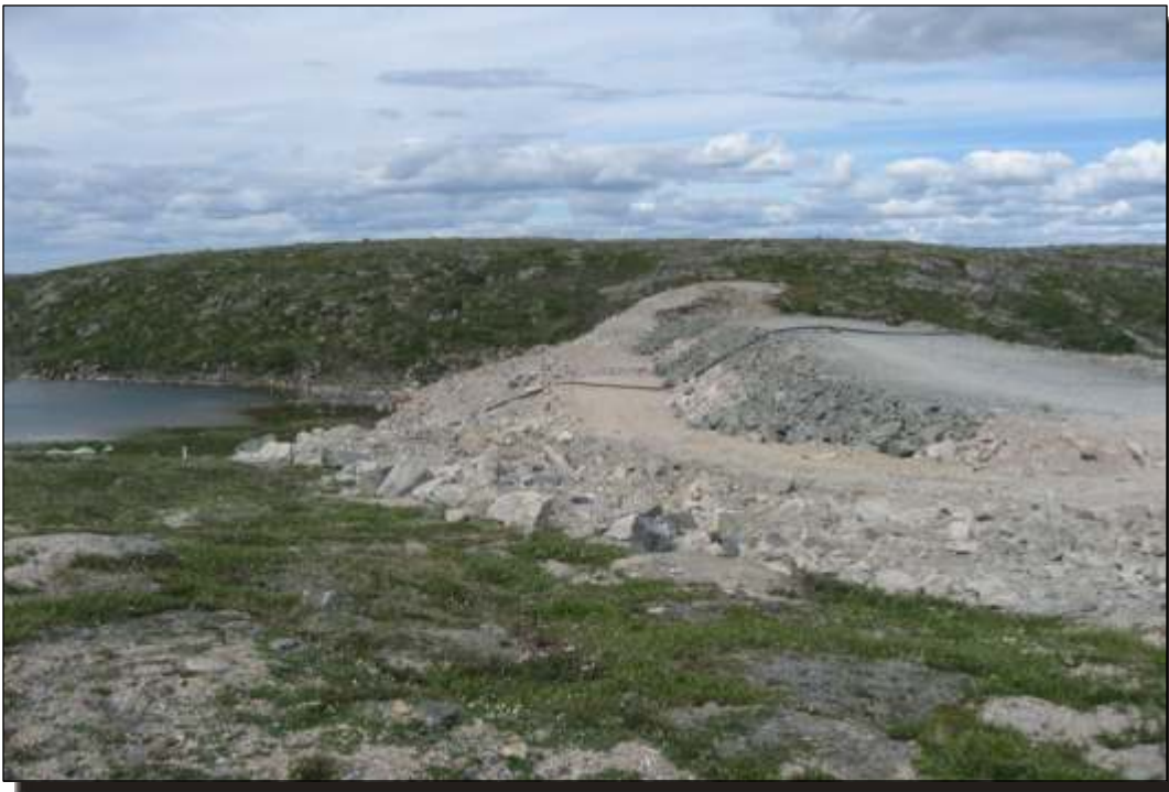
Photo A.4 West Dam: Downstream slope, looking north.
