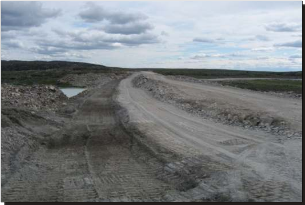
Photo B.5 Divider Dyke A: Dyke Crest. Filter zone excavated prior to replacement.
