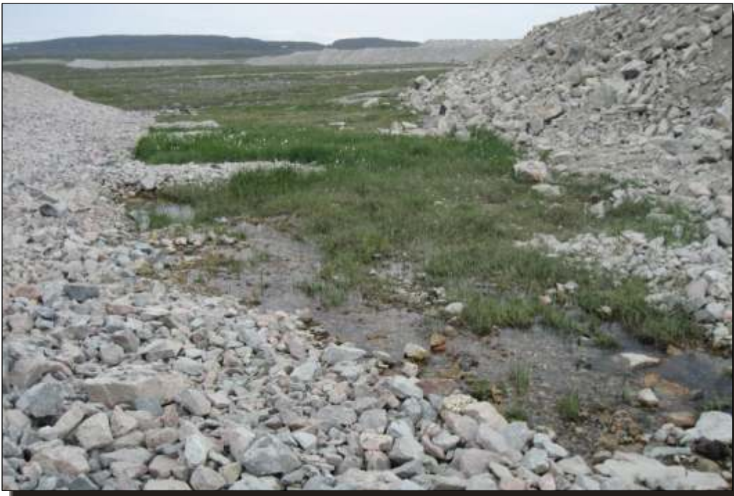
Photo H.10 C1 Diversion Channel - Reach C: Vegetated channel, spurs along north berm.
