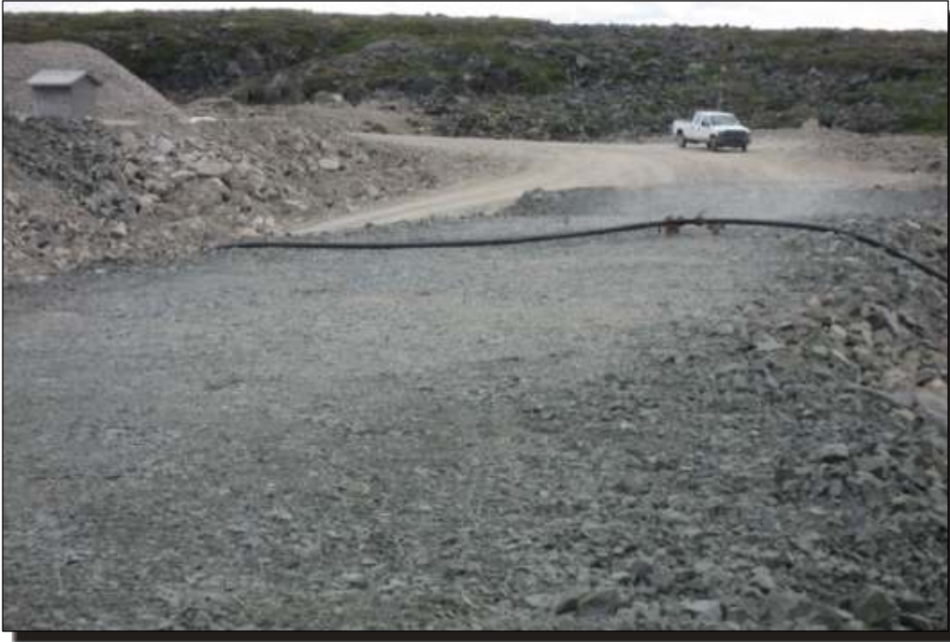
Photo A.7 West Dam: Crest, looking south.
