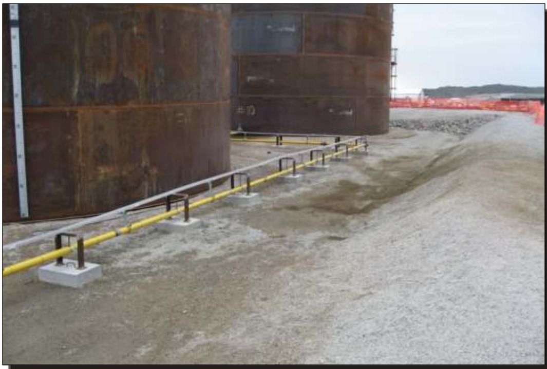
Photo D.12 Phase 2 Tankfarm: North berm, looking west.
