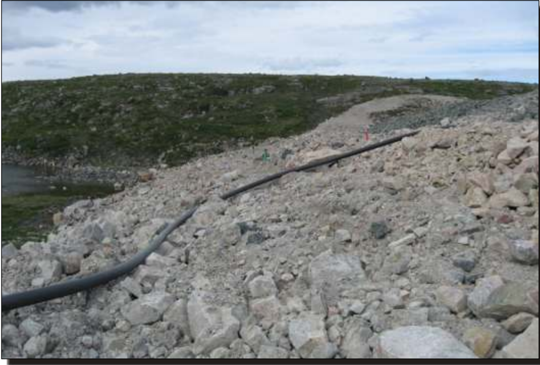
Photo A.5 West Dam: Downstream slope, looking north.
