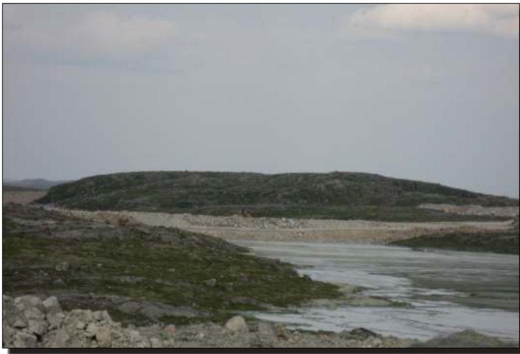
Photo B.1 Divider Dyke A: Upstream side, looking west across process kimberlite deposition area.
