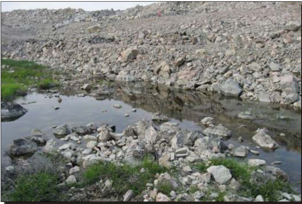
Photo C.5 East Dam: Downstream slope. Ponded water at dam toe.
