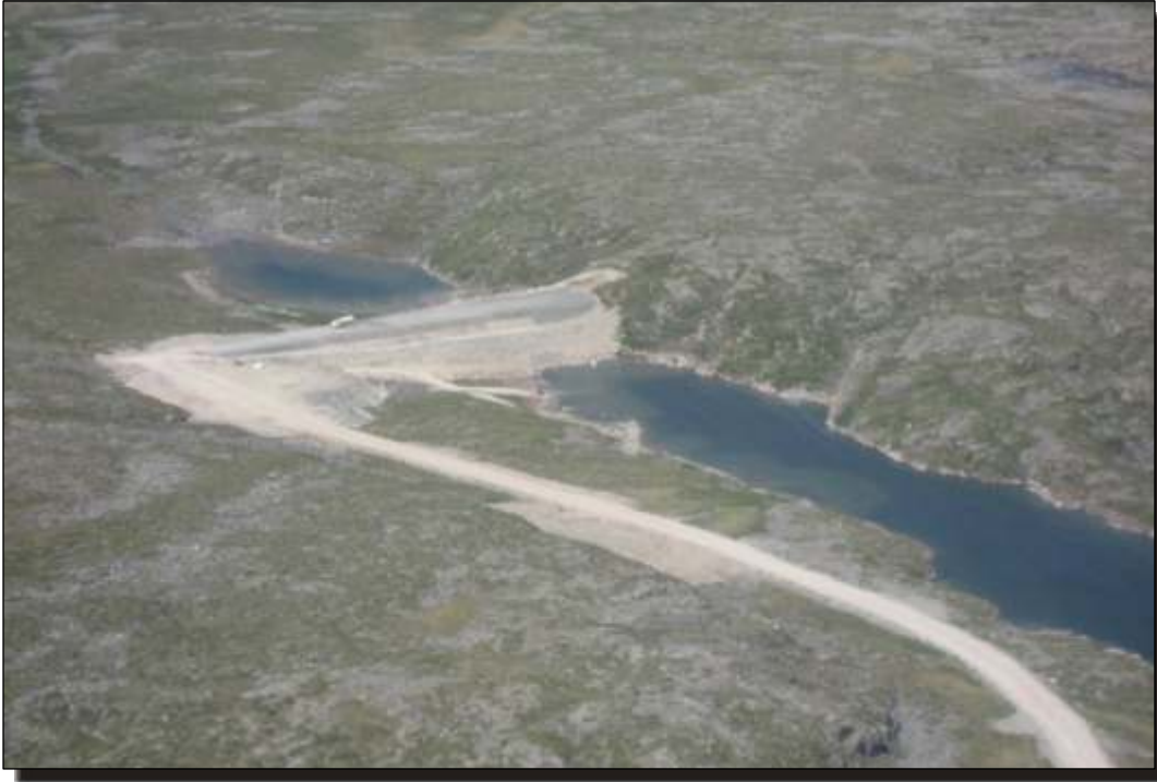
Photo A.1 West Dam: Upstream slope, looking northwest.
