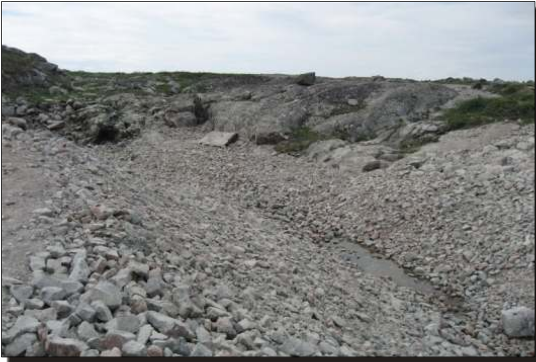
Photo H.2 C1 Diversion Channel - Reach A: Reach Ainlet.
