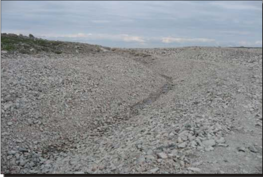
Photo H.3 C1 Diversion Channel - Reach A: Upstream portion.
