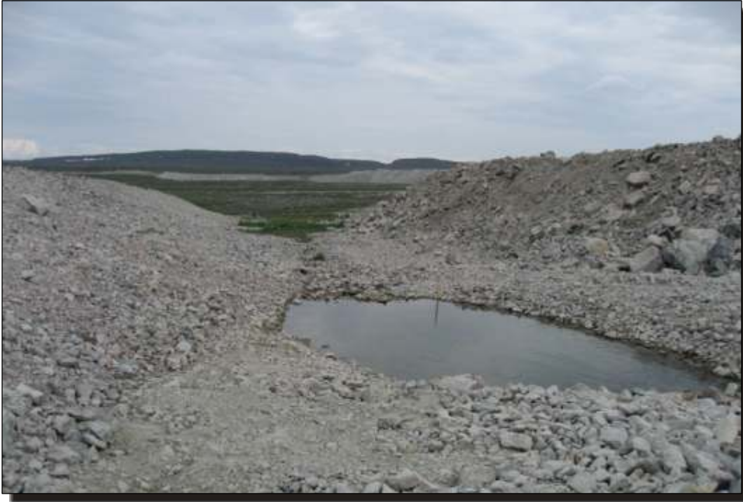
Photo H.9 C1 Diversion Channel - Reach B: Ponded water and coarse rock section.
