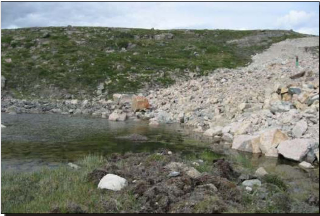
Photo A.8 West Dam: Pond at downstream dam toe.
