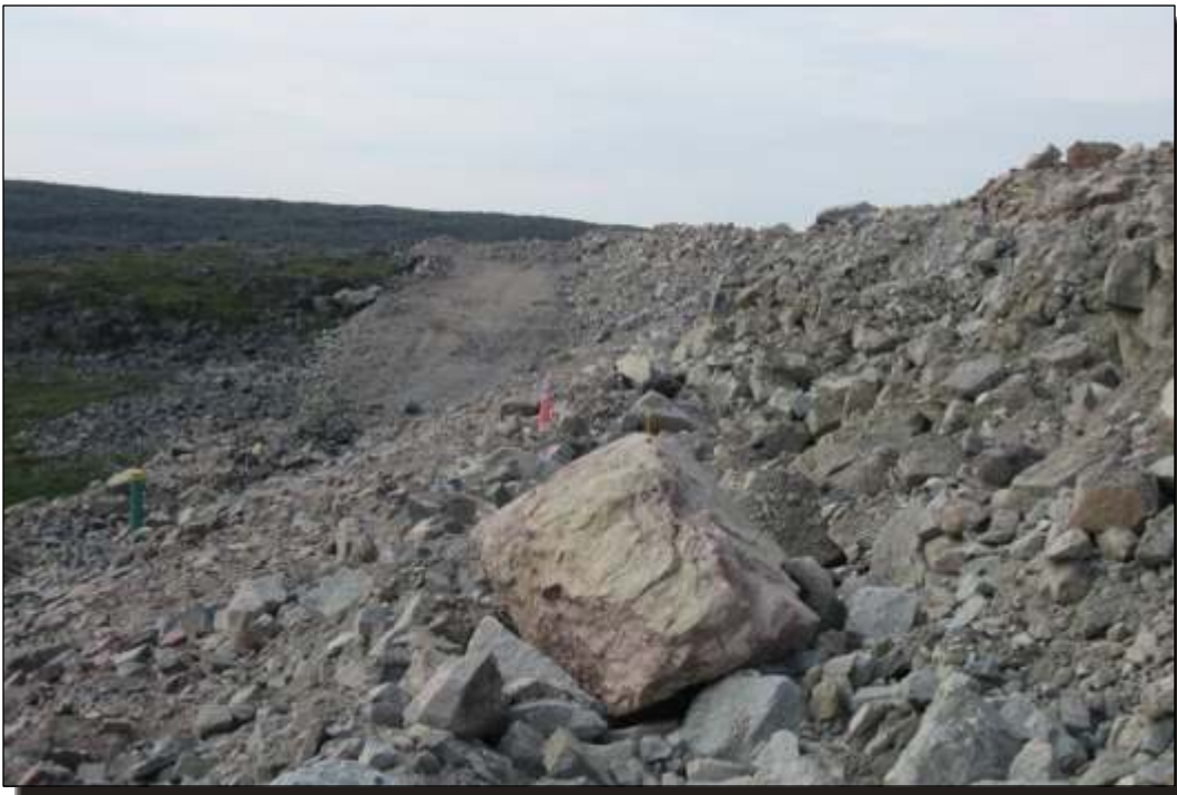
Photo C.7 East Dam: Downstream slope. Settlement monument is yellow pipe.
