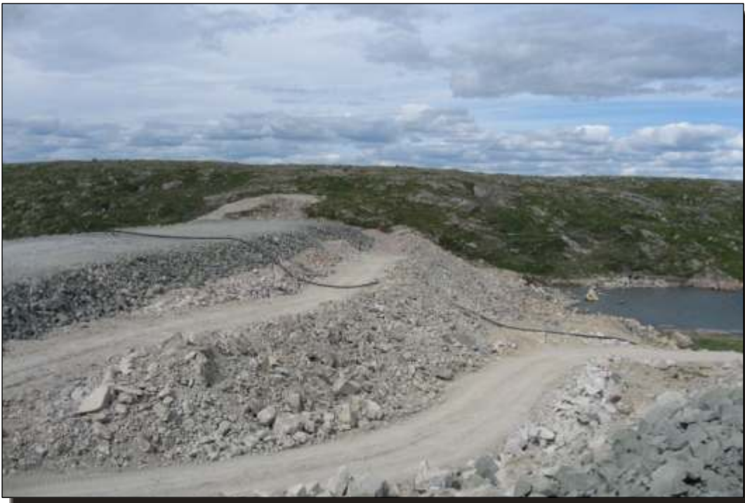
Photo A.6 West Dam: Upstream slope, looking north.
