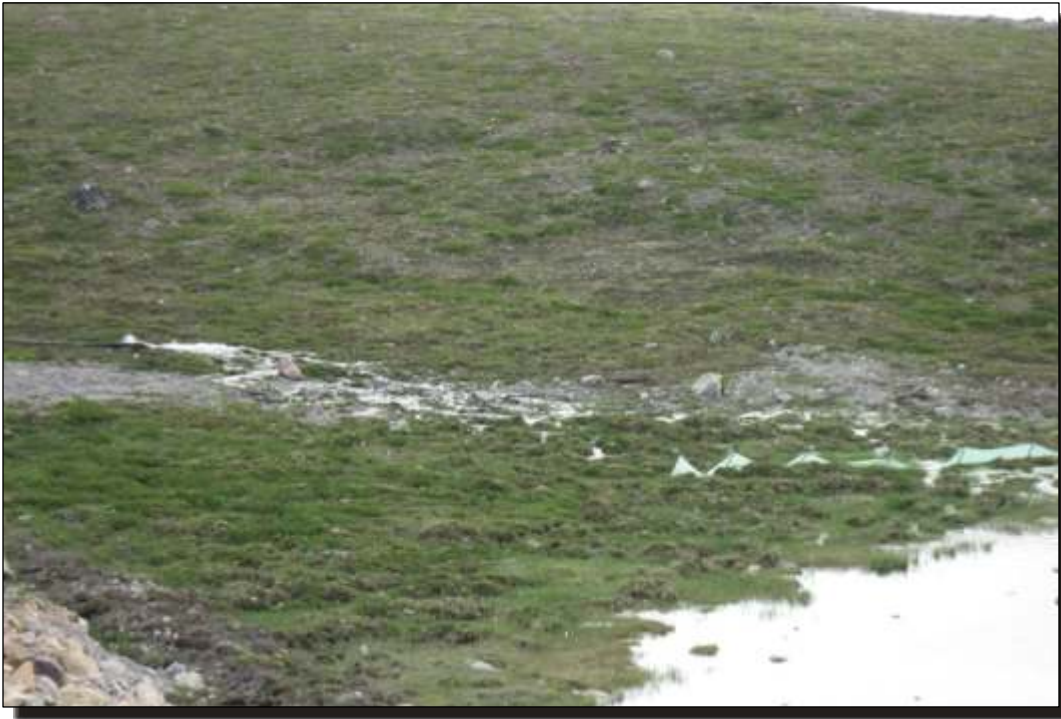
Photo A.3 West Dam: Discharge downstream of the dam.
