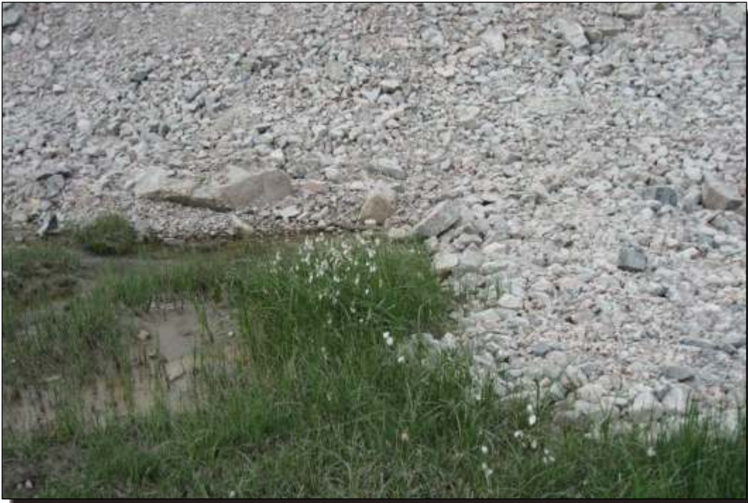
Photo H.11 C1 Diversion Channel - Reach C: Ponded water along spurs.
