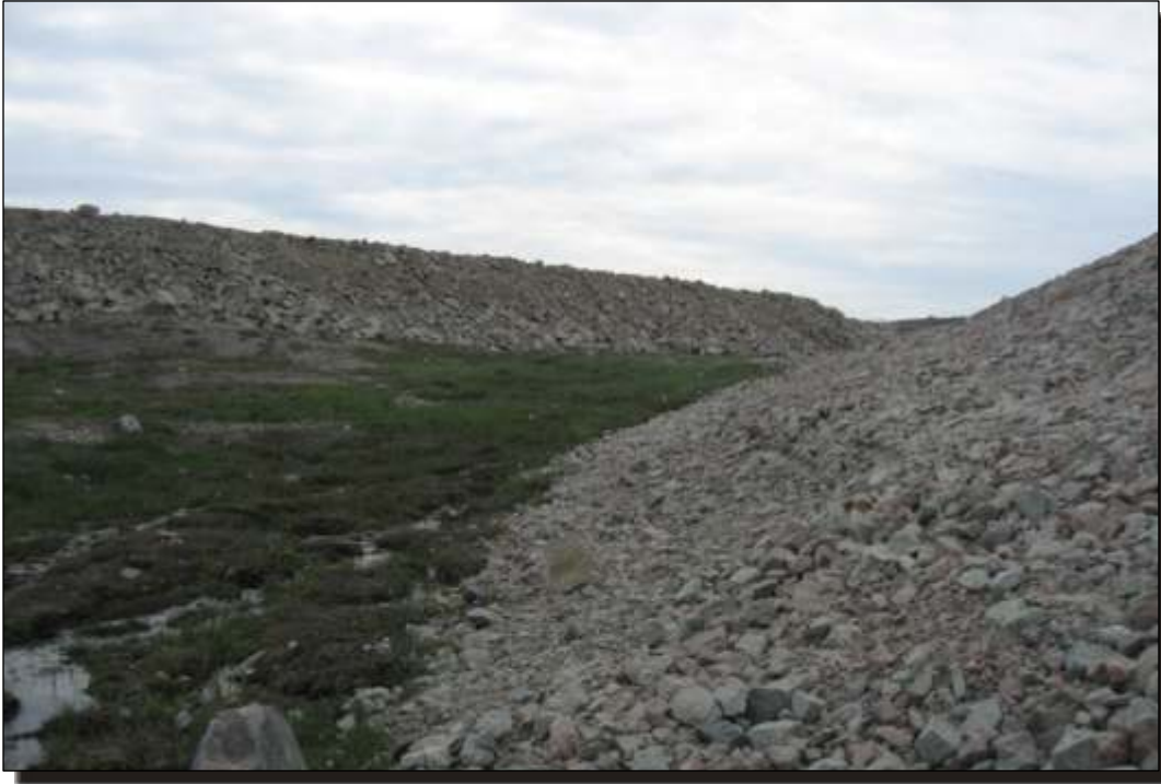
Photo H.15 C1 Diversion Channel - Reach C: Looking upstream.
