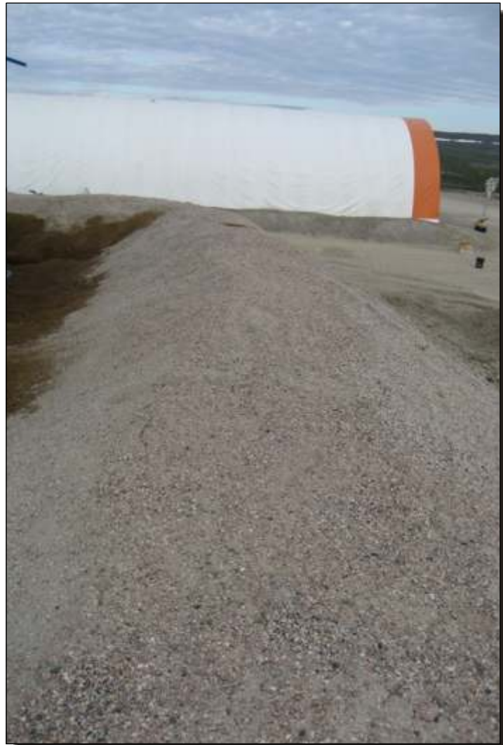
Photo F.5 Airstrip Fuel Tank: Containment Berm Crest.
