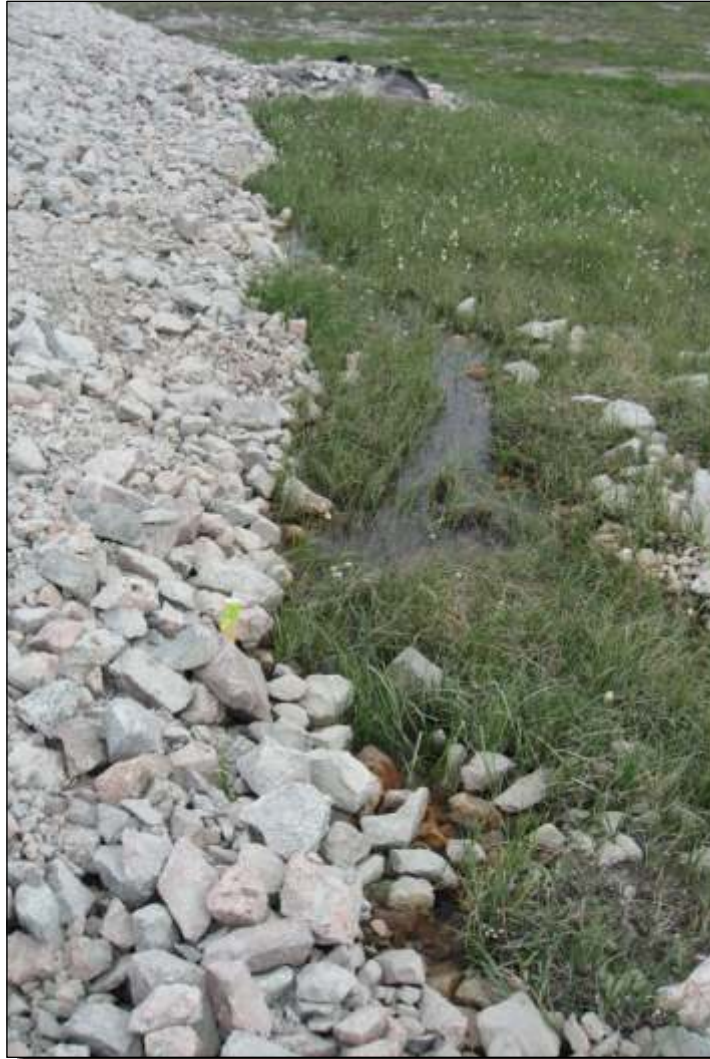
Photo H.12 C1 Diversion Channel - Reach C: Flow adjacent to north berm.
