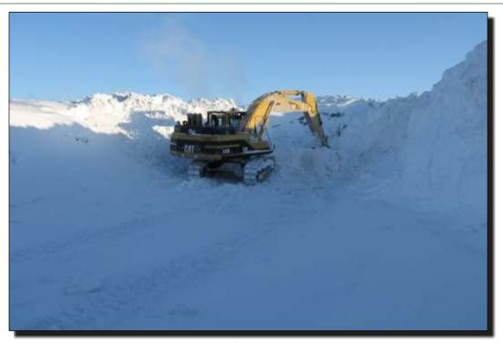
Photo 21 Southeast Dam Excavation of snow from key trench.
