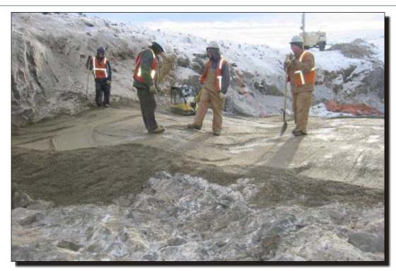
Photo 7 East Dam Placing saturated levelling course.
