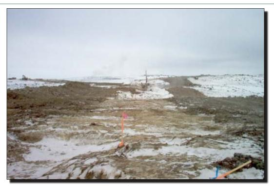
Photo 17 Southeast Dam Drilling percolation holes prior to key trench excavation.
