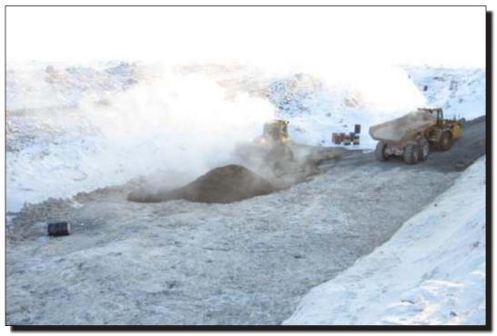
Photo 24 Southeast Dam Placement of levelling course.
