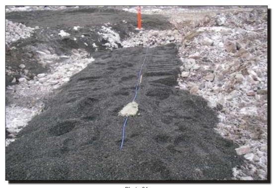
Photo 34 Southeast Dam Horizontal ground temperature cable installation.
