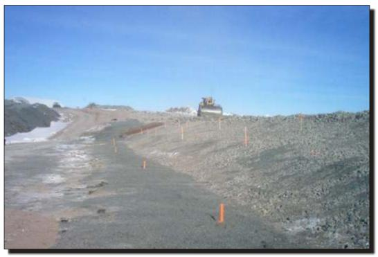
Photo 12 East Dam Construction of run-of-mine rockfill shell.
