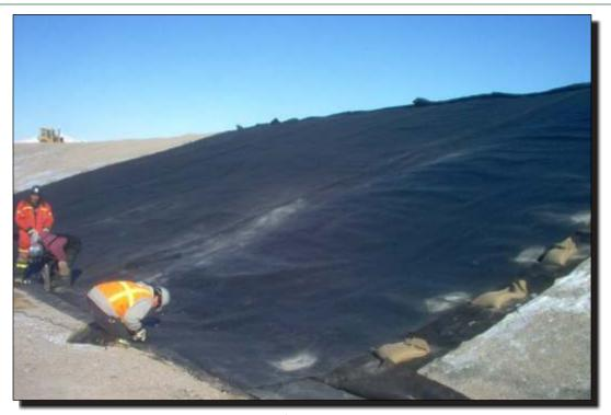
Photo 15 East Dam Extrusion welding of liner hinge.
