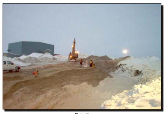
Photo 10 East Dam Placement and compaction of Fillet Zone.
