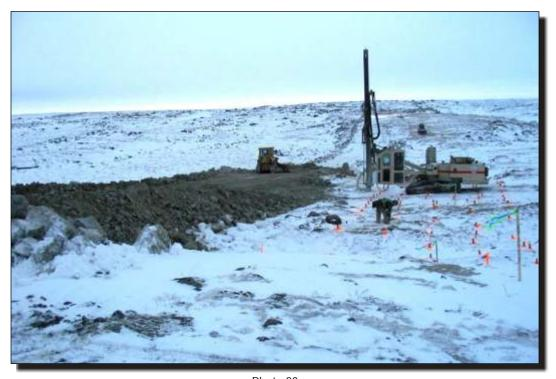
Photo 20 Southeast Dam Drilling holes for key trench blasting.
