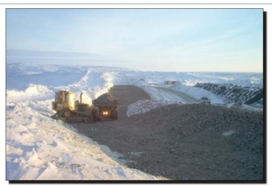
Photo 11 East Dam Transition material placed over key trench material.
