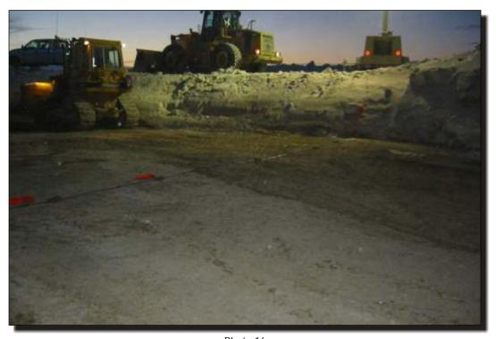
Photo 16 East Dam Installation of horizontal ground temperature cable.
