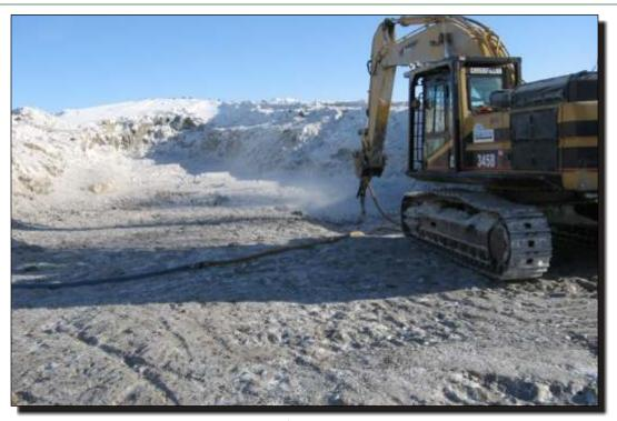
Photo 23 Southeast Dam Excavator cleaning key trench with compressed air and ripper tooth.
