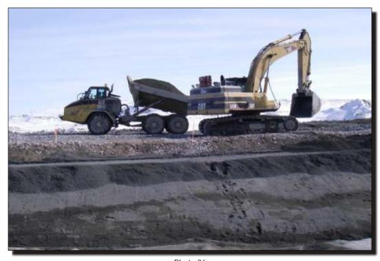
Photo 26 Southeast Dam Placement of downstream liner bedding.
