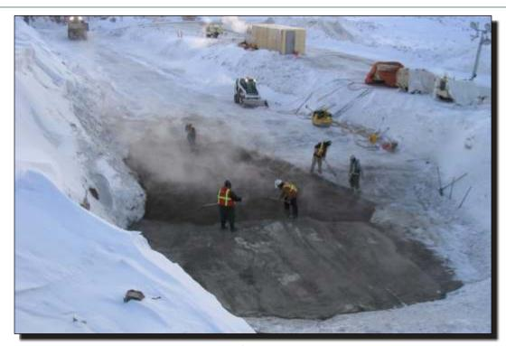
Photo 9 East Dam Levelling course placement.
