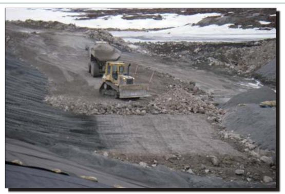
Photo 29 Southeast Dam Placement of till zone upstream of liner.
