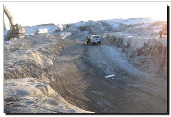
Photo 25 Southeast Dam Fillet zone along upstream side of key trench.
