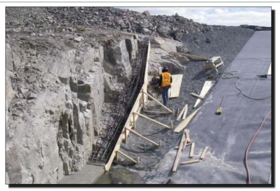
Photo 31 Southeast Dam Re-enforcing steel and formwork for concrete beam.
