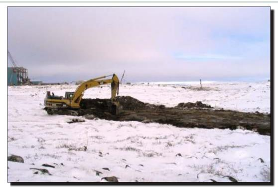
Photo 19 Southeast Dam Grubbing footprint of dam with an excavator.
