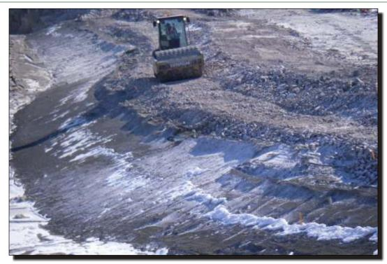
Photo 27 Southeast Dam Placement of transition material.
