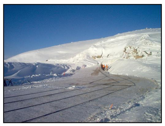
Figure 1. Installation of thermosyphon evaporator loops at West Dam. Aspect: N
