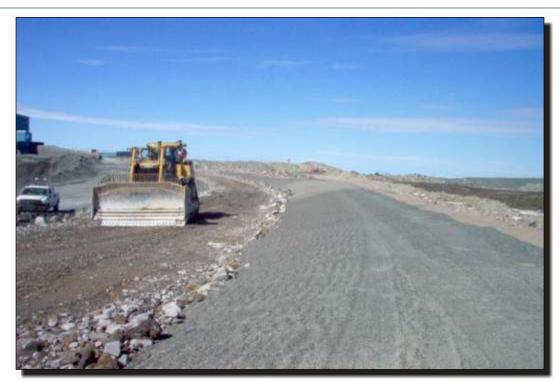
Photo 13 East Dam Placement of upstream till zone.
