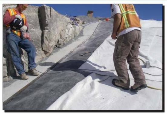
Photo 33 Southeast Dam HDPE Liner attached to concrete beam.
