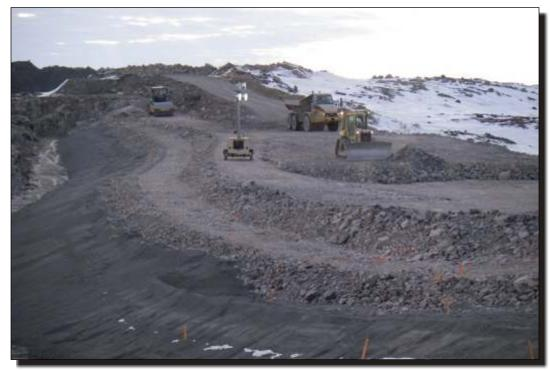
Photo 28 Southeast Dam Placement of run-of-mine rockfill shell.
