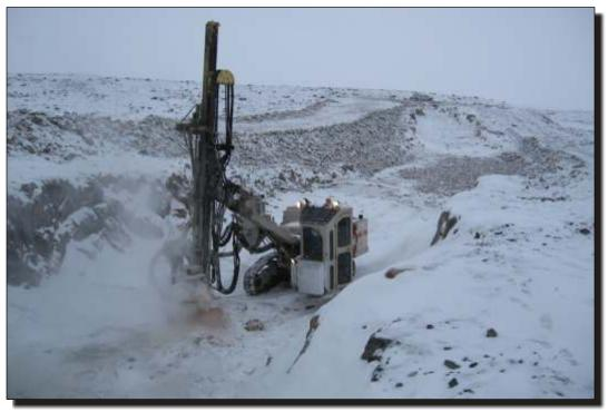
Photo 18 Southeast Dam Drilling percolation test holes after key trench was excavated.
