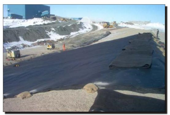
Photo 14 East Dam Installation of second liner phase.
