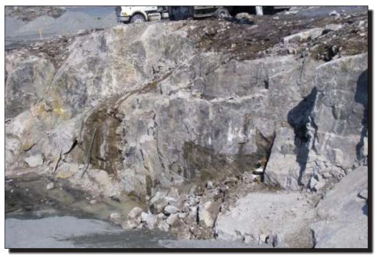
Photo 30 Southeast Dam Removal of loose rock from north abutment.
