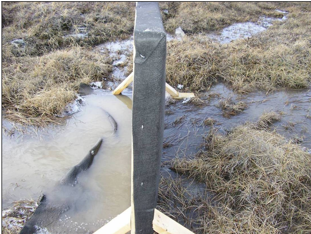
Figure 7 Silt Curtain effectiveness
