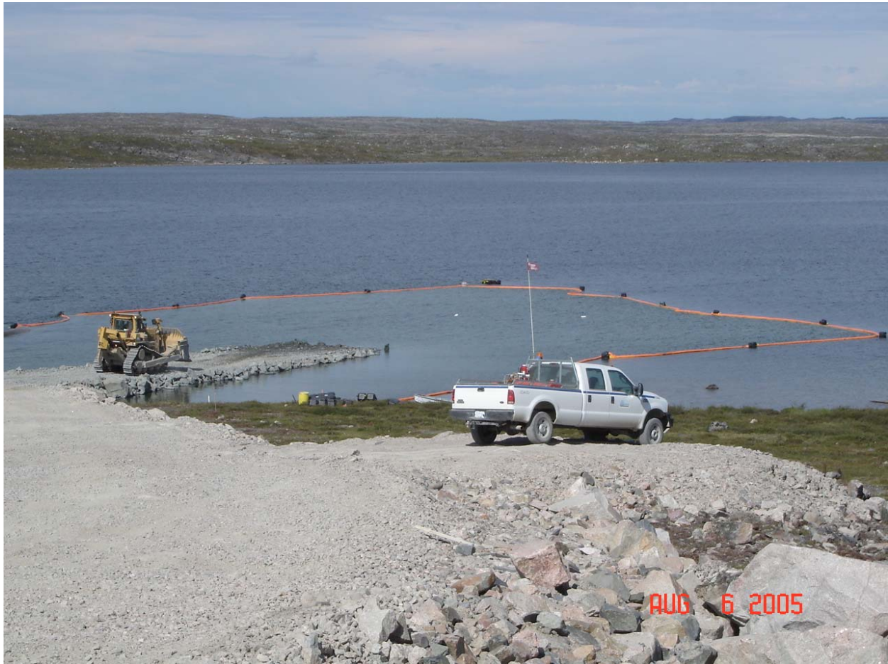
Picture 6: August 6, 2005 looking north on the Carat access road, note the black floats attached to the curtain to prevent it from being pulled below surface.
