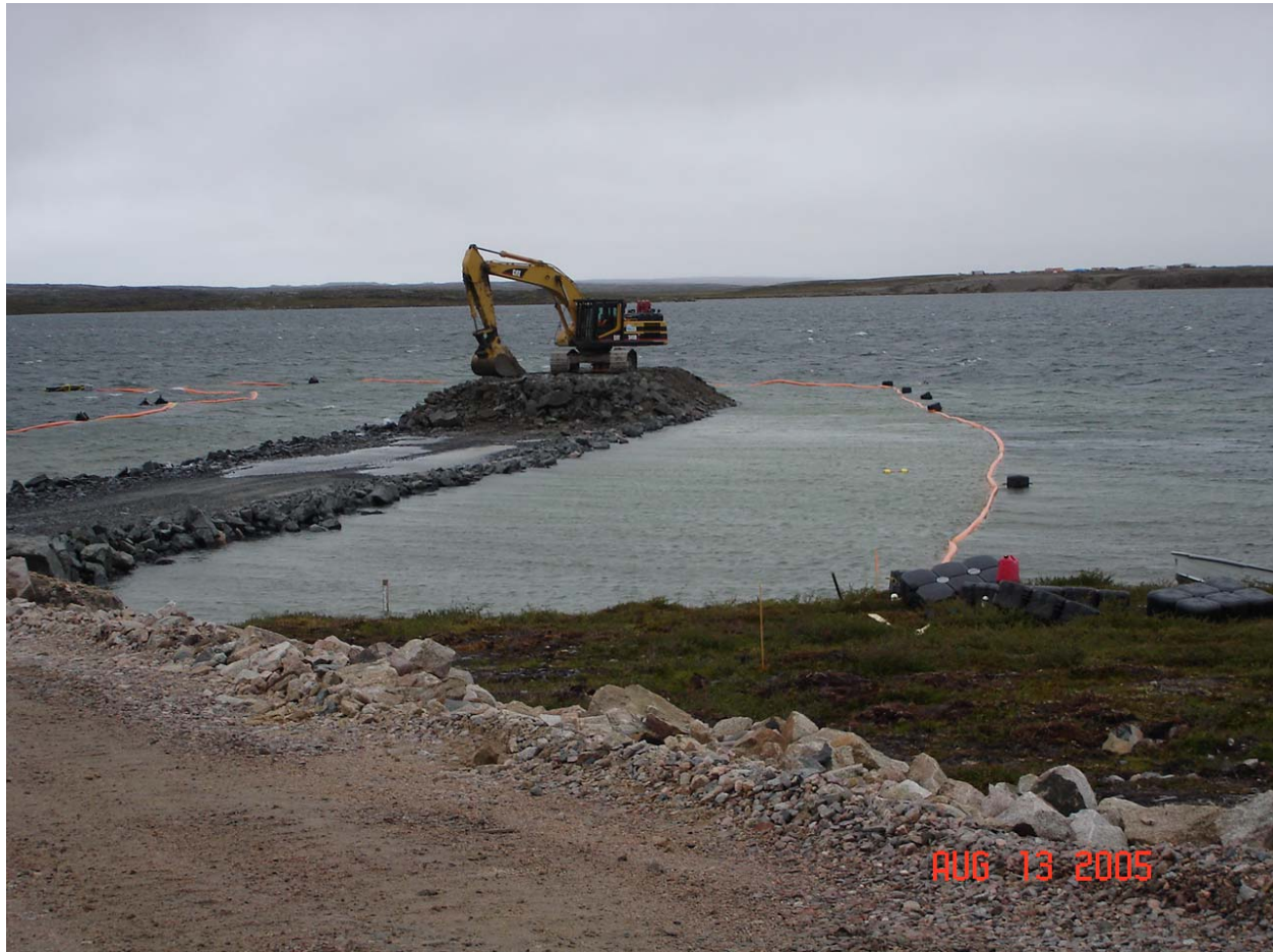
Picture 15: August 13, 2005 looking north from the causeway access road approximately 50m from Carat shoreline. The 345 works at placing the second lift of run of mine on the causeway.
