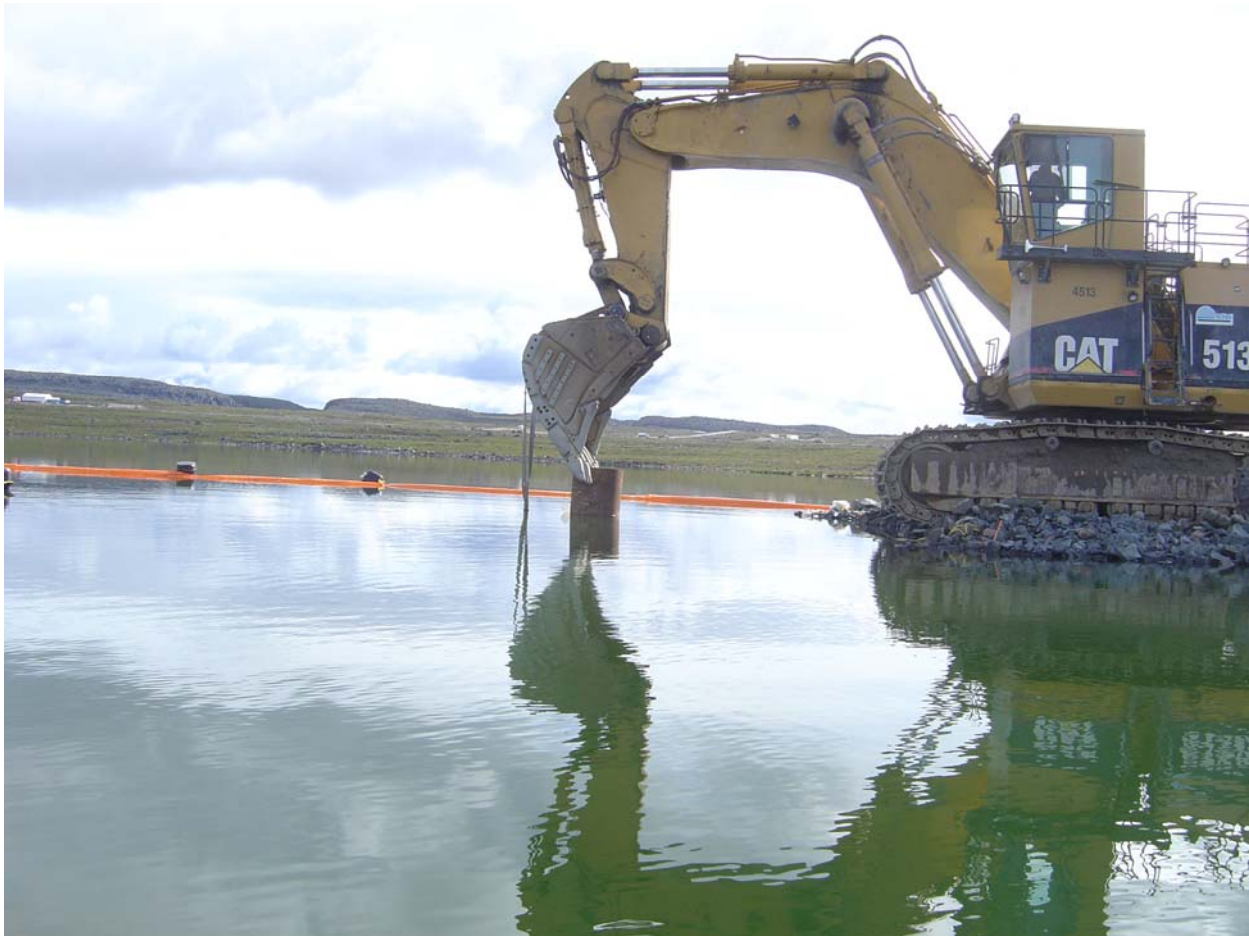
Picture 13: August 9, 2005 looking east from a boat 5130 excavator has placed intake pipe into causeway.
