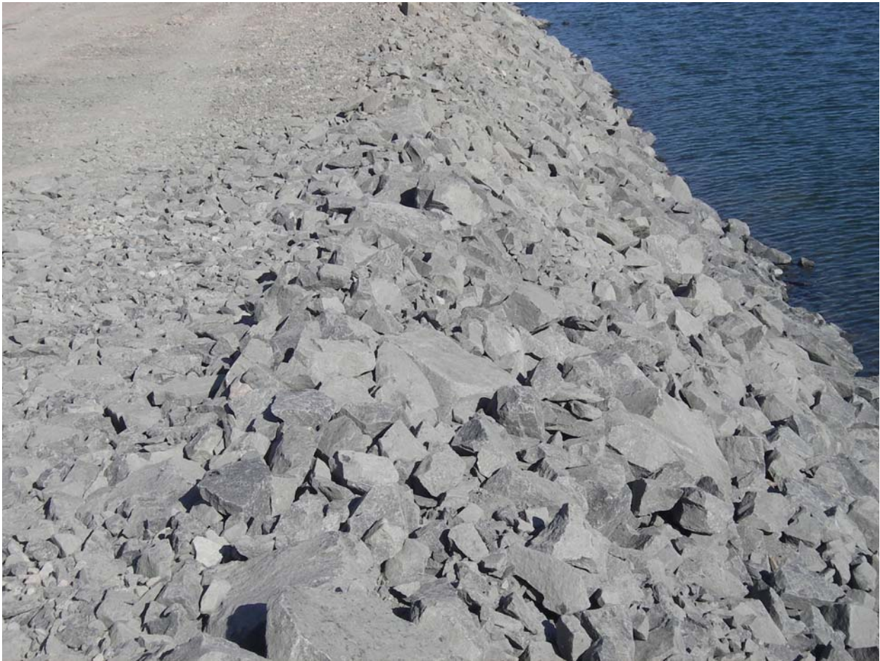
Picture 3: September 6, 2005 looking NE along eastern edge of the causeway, close-up of clean diabase cap material.
