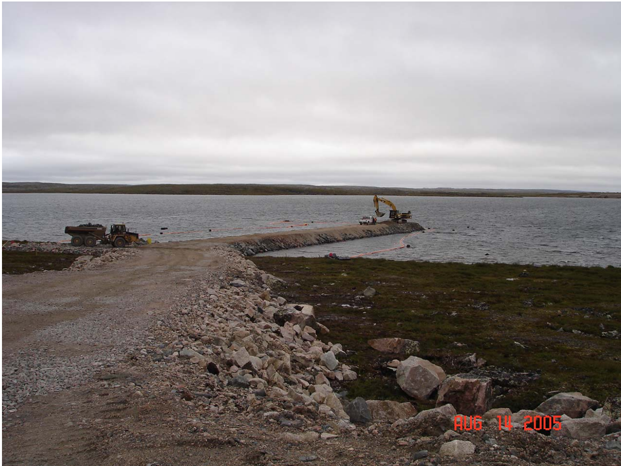
Picture 16: August 14, 2005 looking north down the causeway access road. The 345 works at placing 2" crush on the surface of the causeway.
