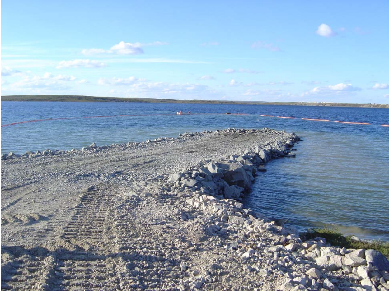
Picture 5: August 5, 2005 end of the day looking north from the end of Carat access road approximately 20m from the Carat Lake shoreline, causeway extends 46m into Carat Lake.
