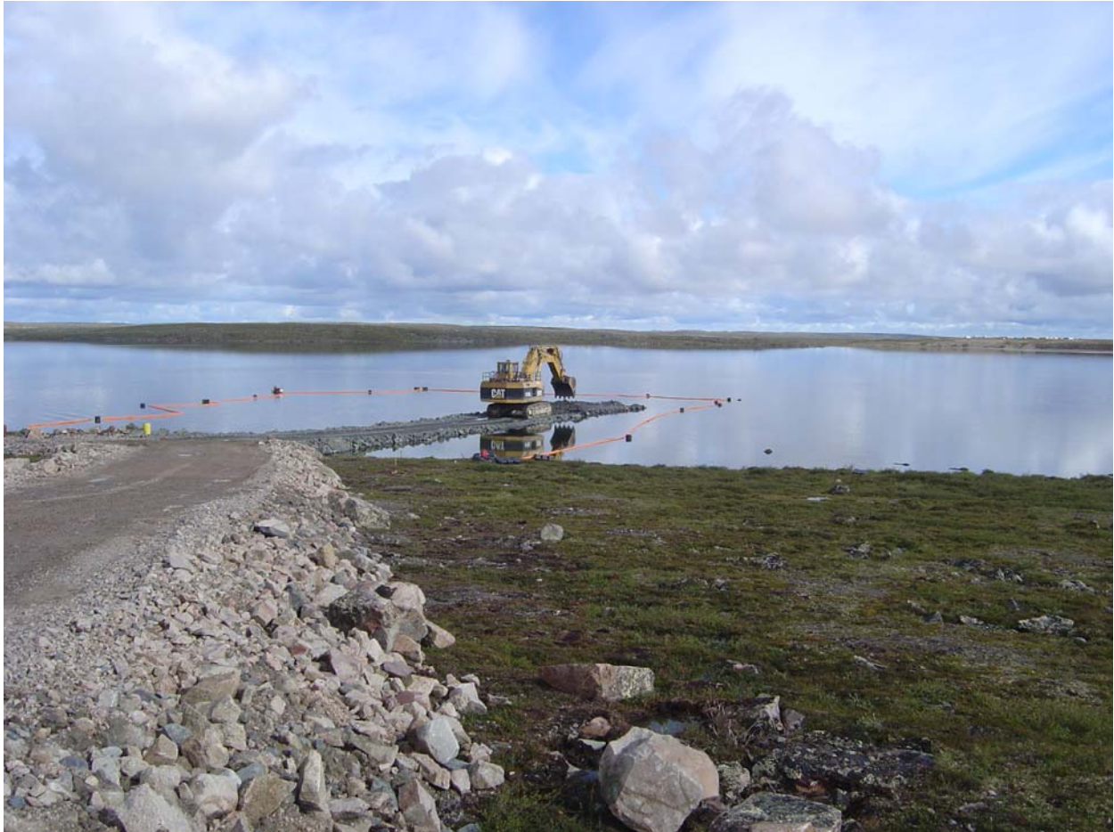
Picture 9: August 9, 2005 looking north along Carat lake access road. The sediment curtain has been repositioned to allow containment around the intake pipe during installation.
