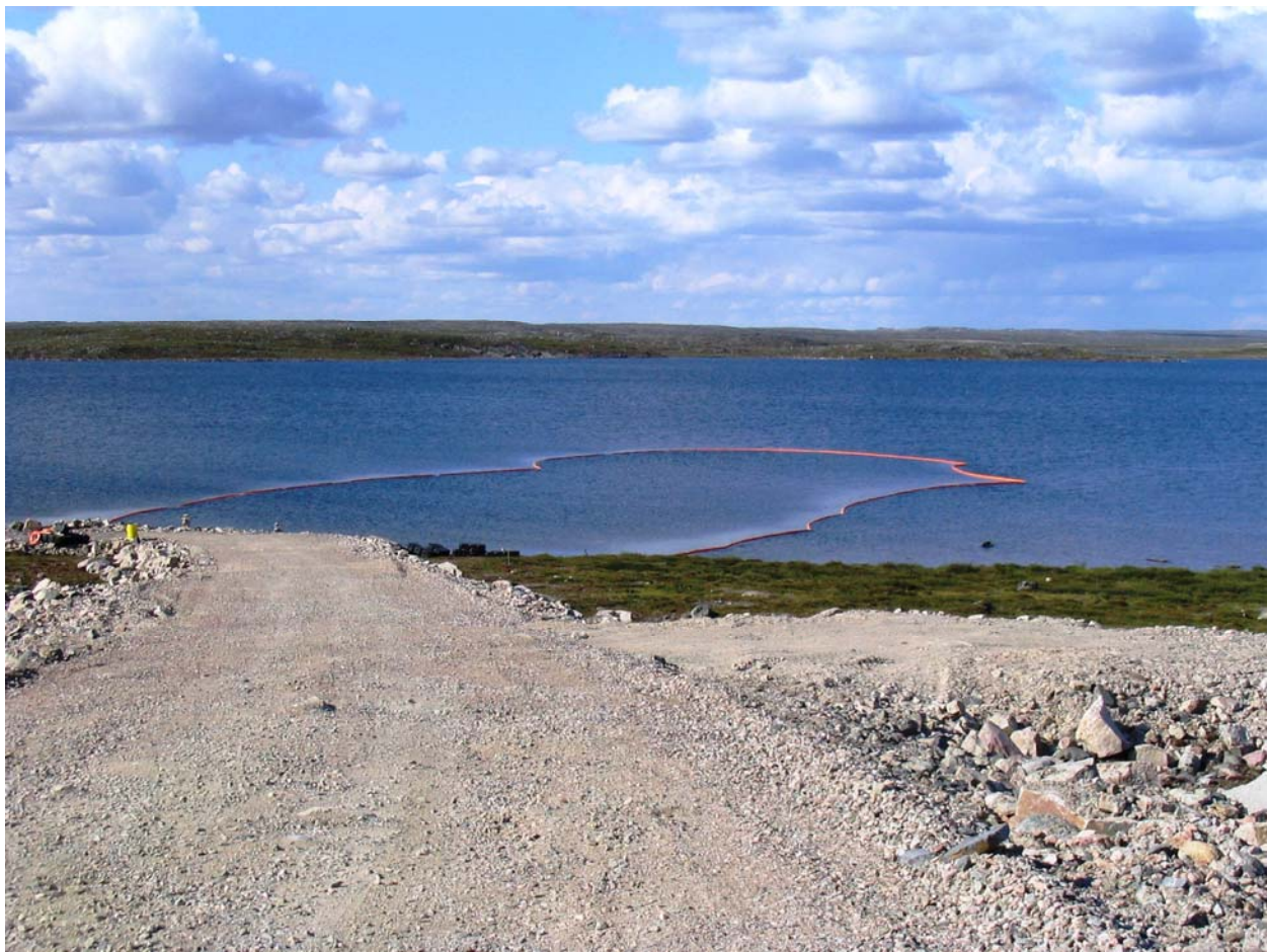
Picture 1: July 29, 2005 looking north from Carat Lake access road at sediment barrier around the construction area prior to construction
