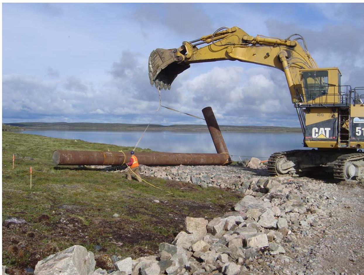
Picture 12: August 9, 2005 looking NW at the end of the Carat causeway access road. The 345 excavator is lifting the intake pipe for placement in the causeway.
