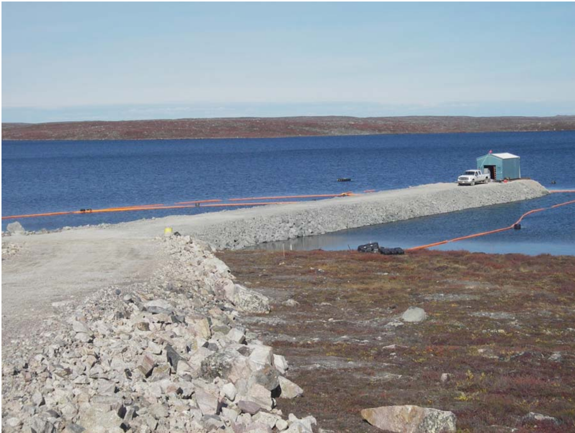
Picture 2: September 6, 2005 looking north on Carat lake access road, causeway capped with clean diabase.
