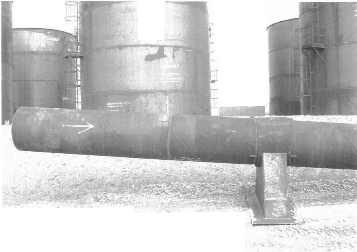
Water intake pipe prior to installation showing the footing to support the pipe above the lake bottom
