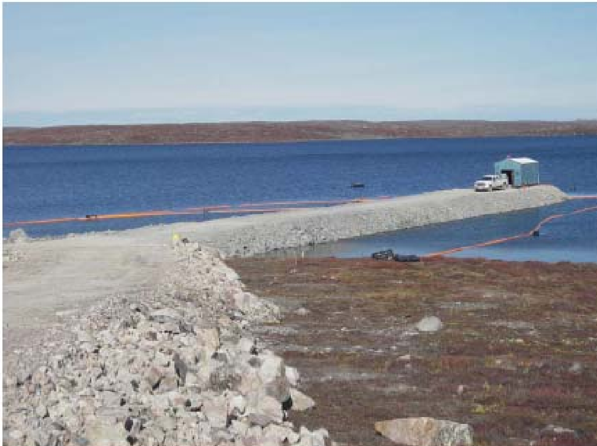
Photo 1: Completed Water Intake Causeway
