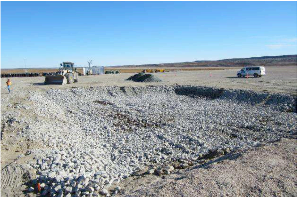
Figure 3: Final excavated area with 6" layer of crush material, view from South West.
