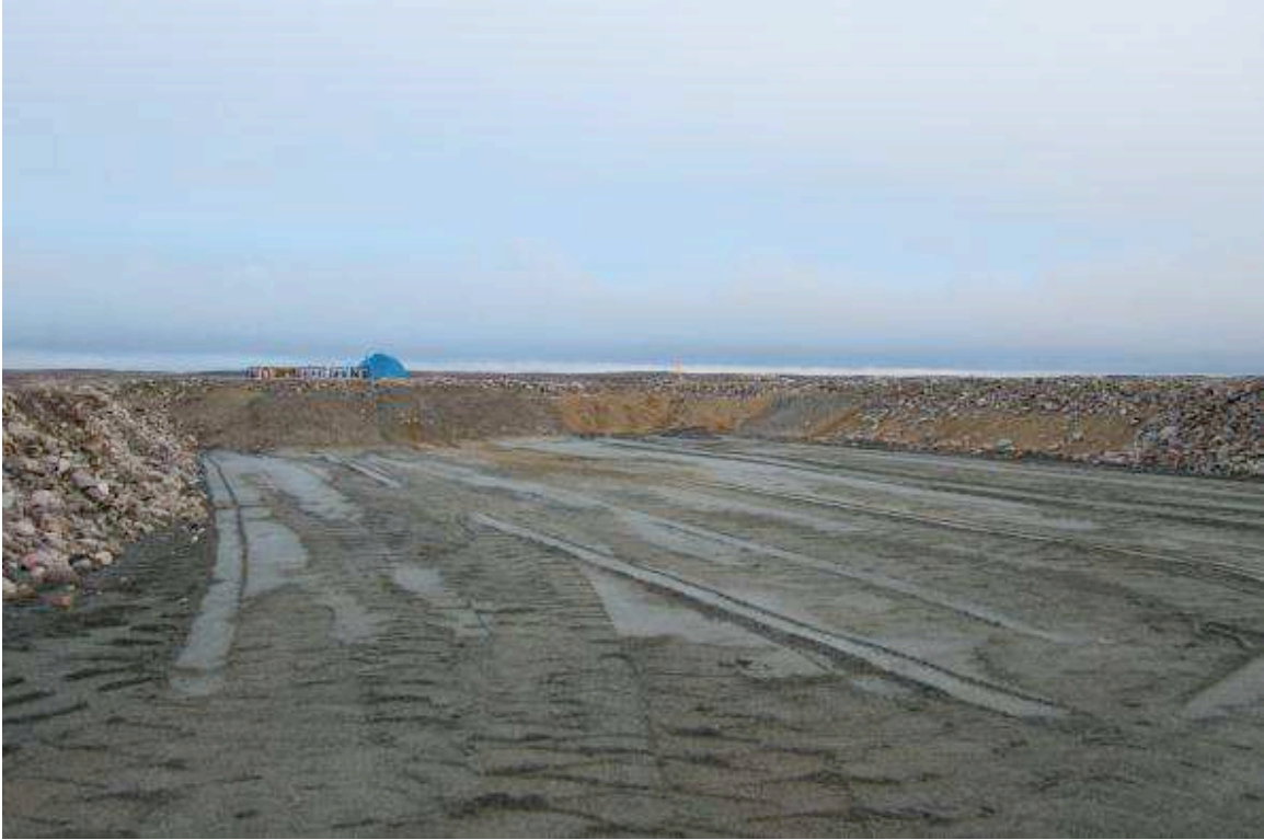
Figure 2: Exposed liner areas with steep slopes were reduced with 2" material.
