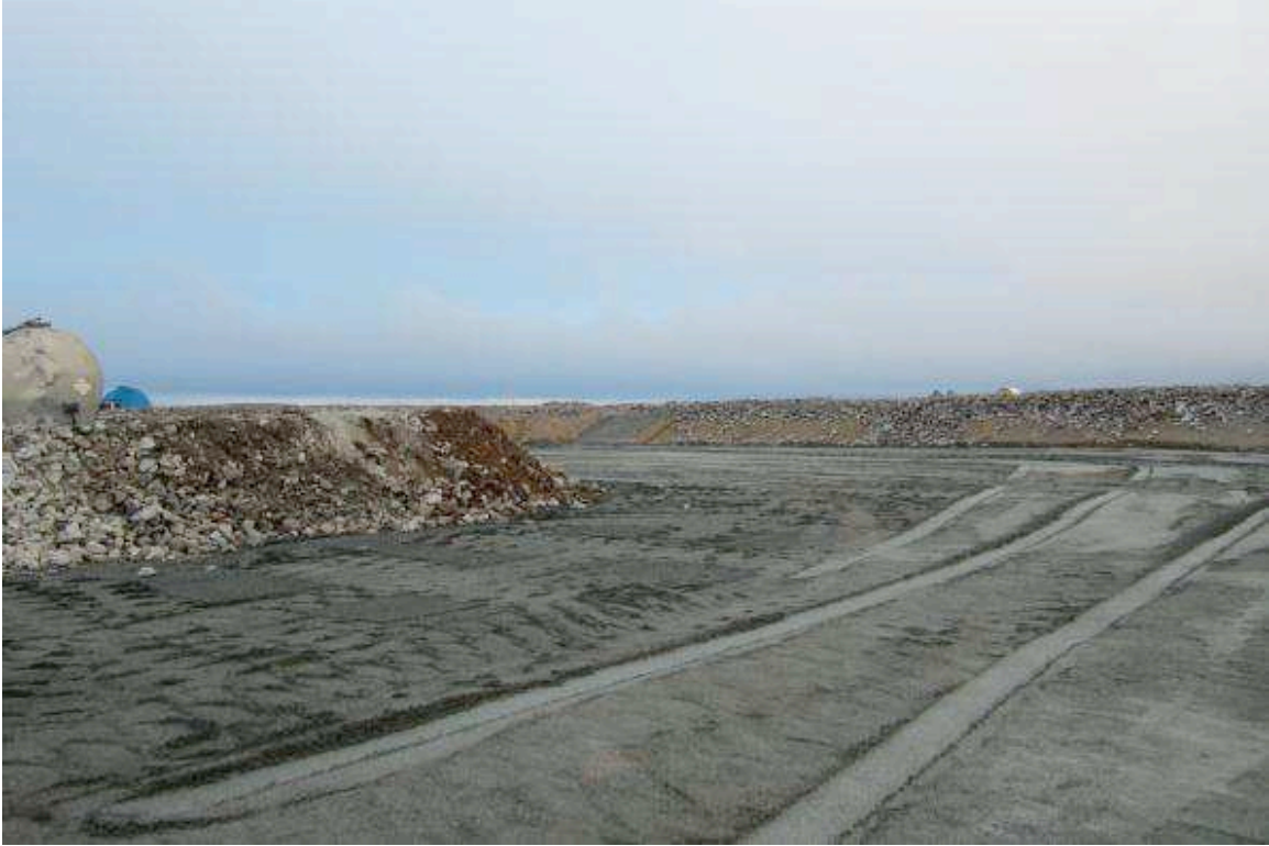
Figure 1: View of the inside L-shaped berm, final elevation. Area prepped and ready for geotextile fabric and liner installation.
