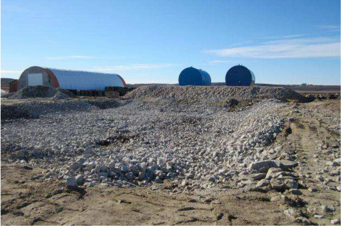
Figure 2: Final excavated area with layer of 6" crush material, view from North West.
