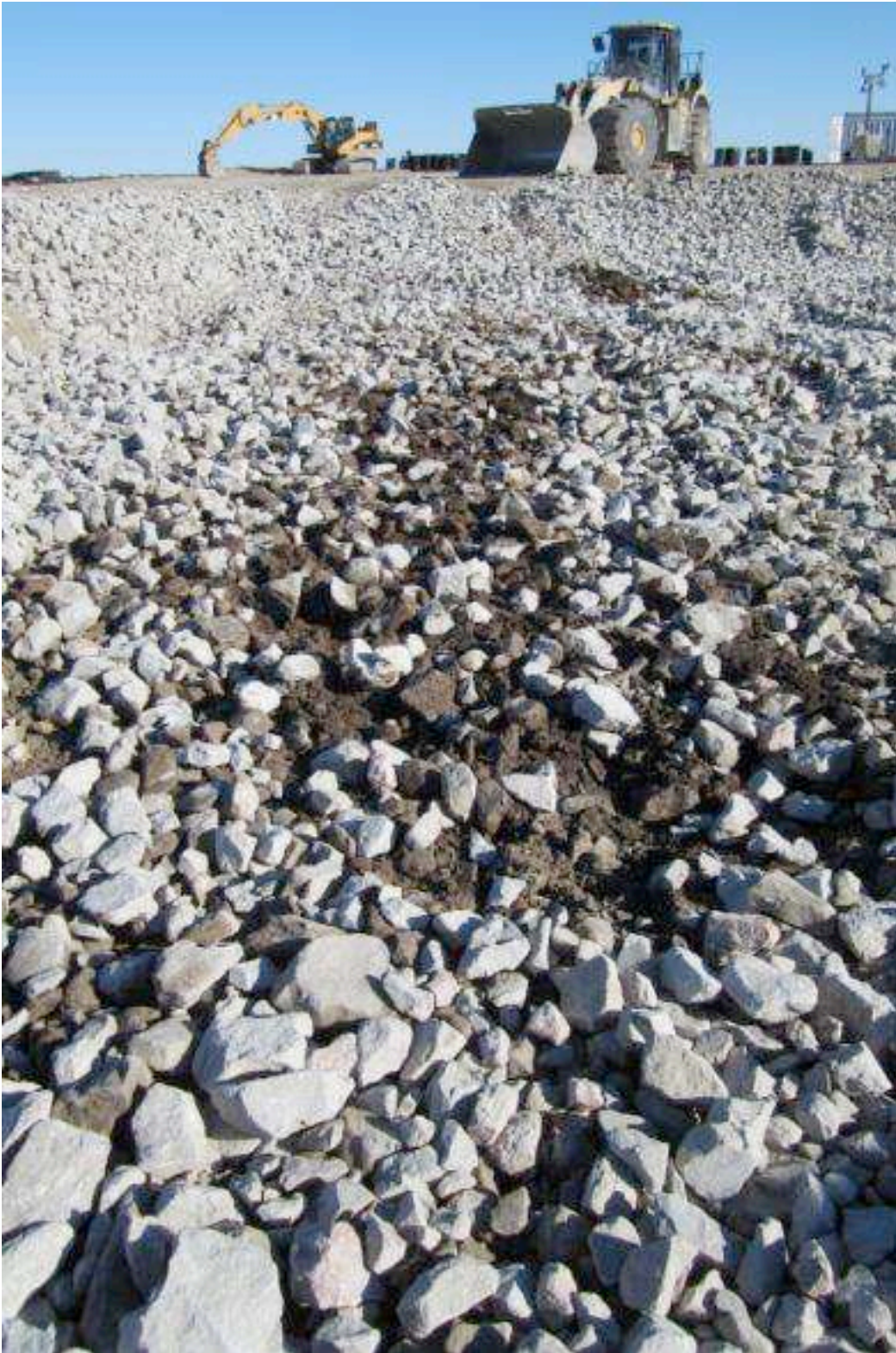
Figure 1: Excavation with layer of 6" crush material.
