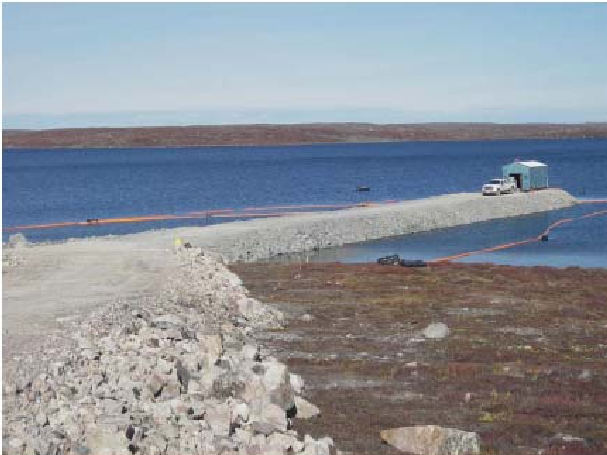
Photo 1: Completed Water Intake Causeway
