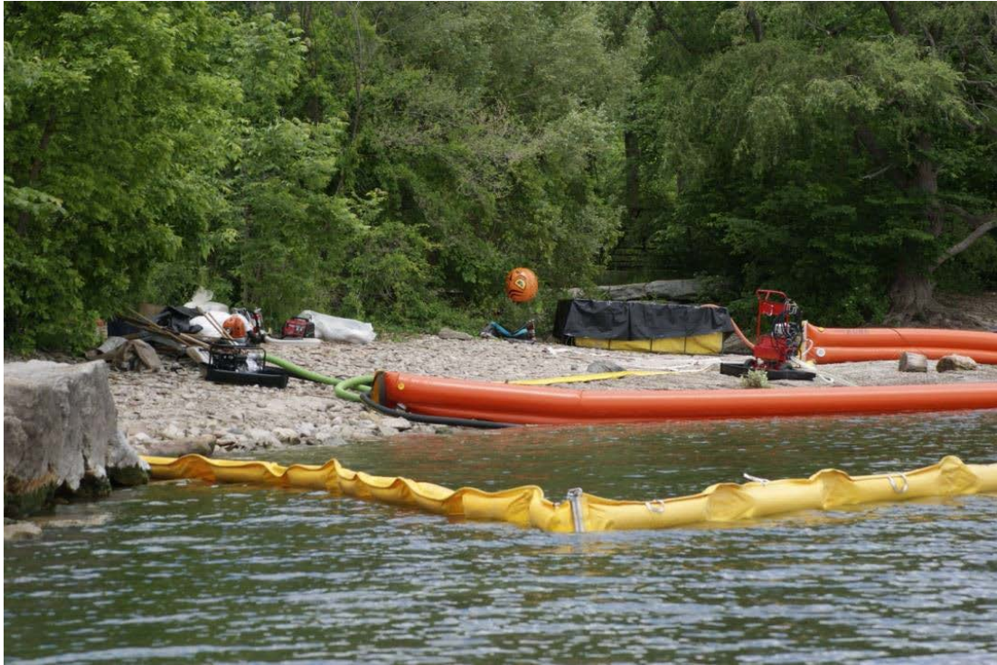
Photo 2: A shallow area near the shoreline that has been boomed off and is in the process of being dewatered using a general purpose pump.
