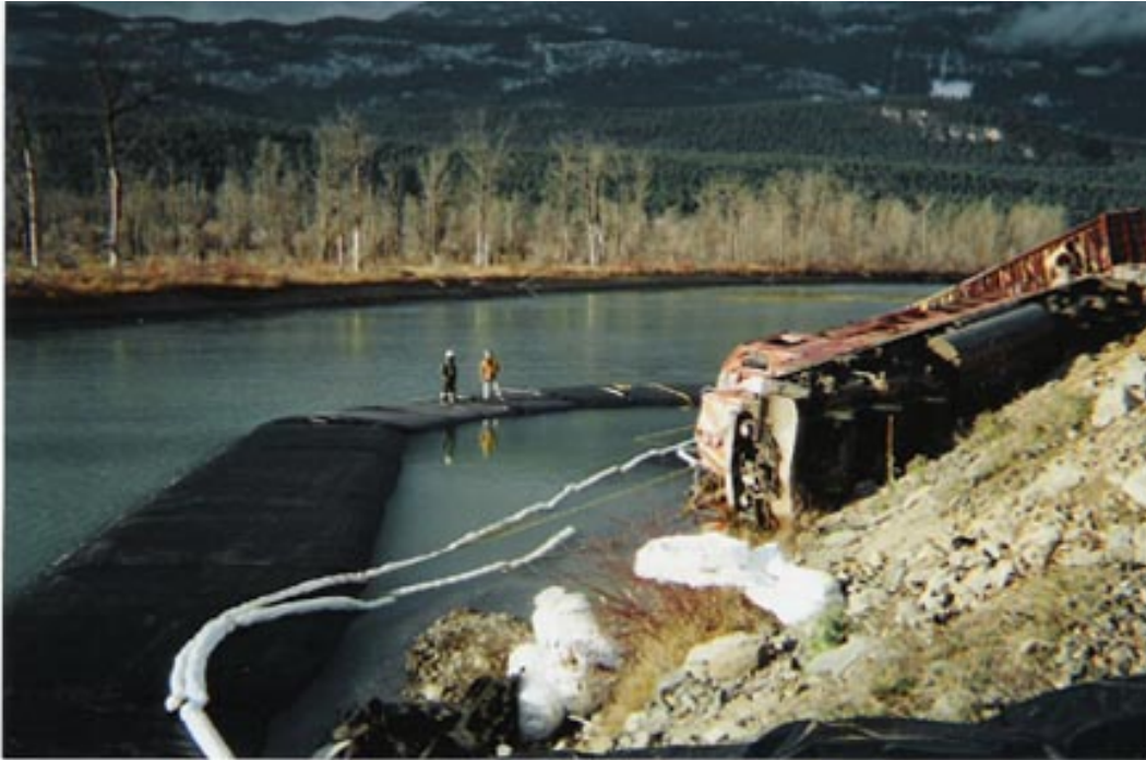
Photo 1: Water-filled dam (Aquadam ®) used at incident scene.
