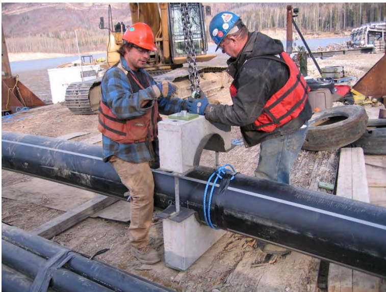
Figure 2 Typical Installation of Anchor Blocks on Pipeline
