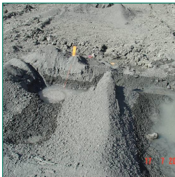
Photo 7.2: Emulsion loaded in a wet pit hole. A film residue is visible on the surface of the water.
