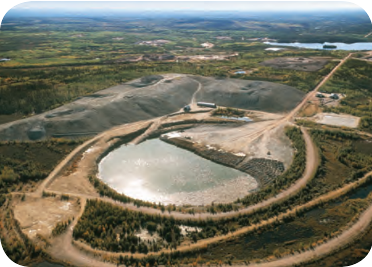
Ongoing decommissioning: Claude open pit mine had been partially backfilled during operations.
