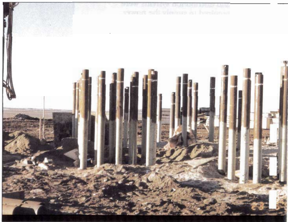
Steel piling for foundations.
