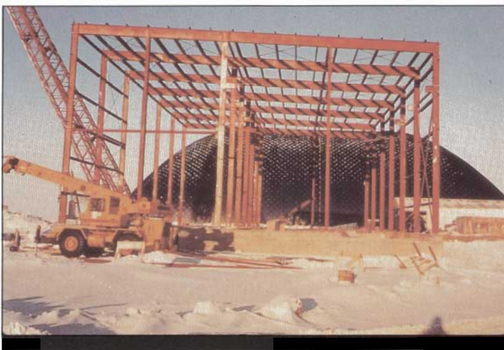
Erected structural steel framework in the foreground with temporary air supported structure in the background to provide a more temperate working environment.
