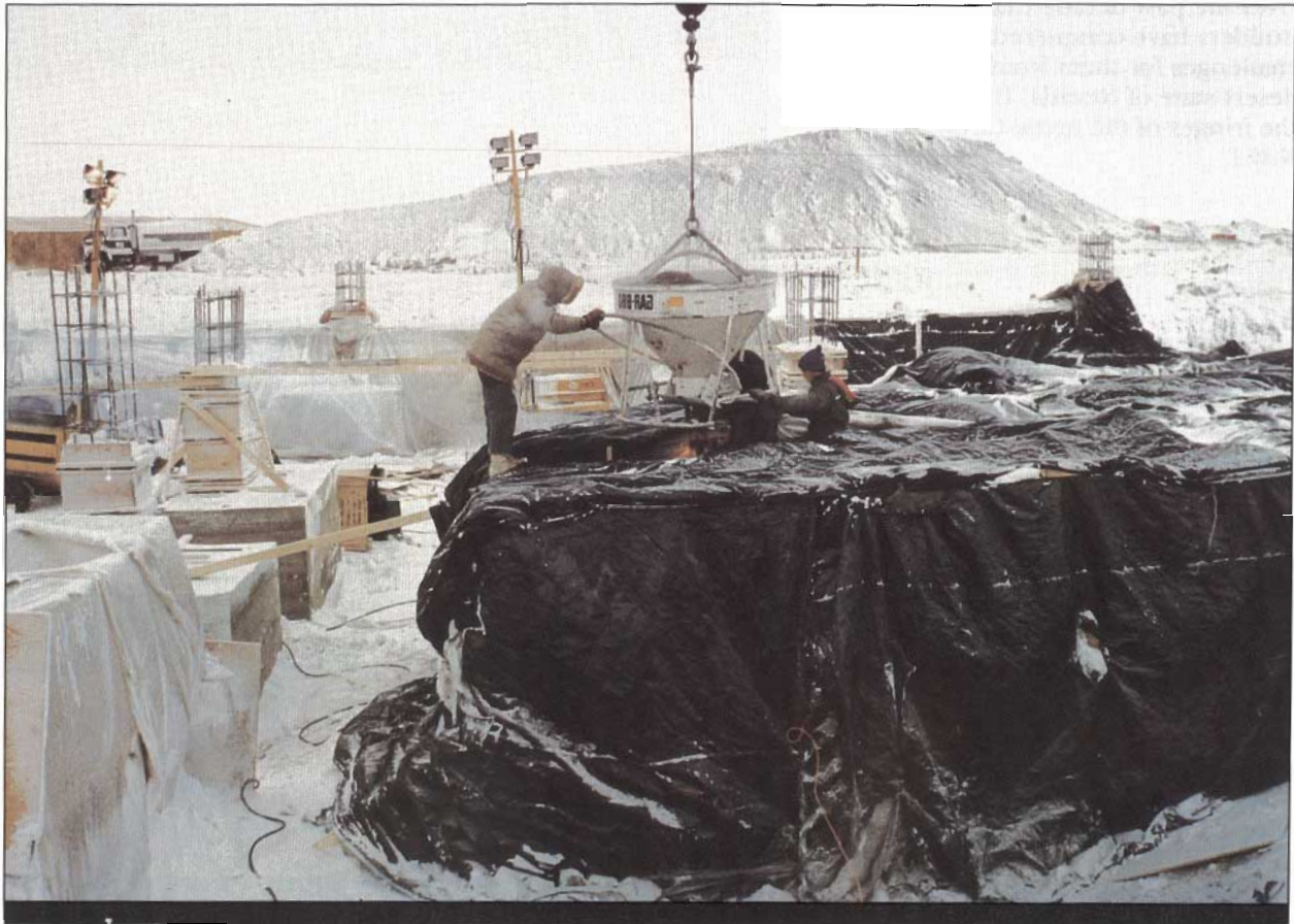
Pouring concrete at the Lupin Mine in -50°C temperatures.
