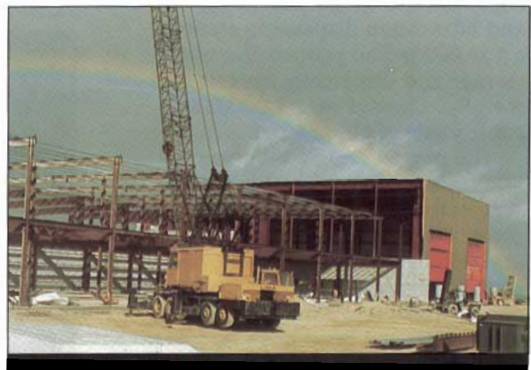
The tight schedule required extensive co-ordination of the numerous trade contractors. Simultaneously, slabs are prepared, steel is lifted, block is laid, and insulation/cladding is installed.
