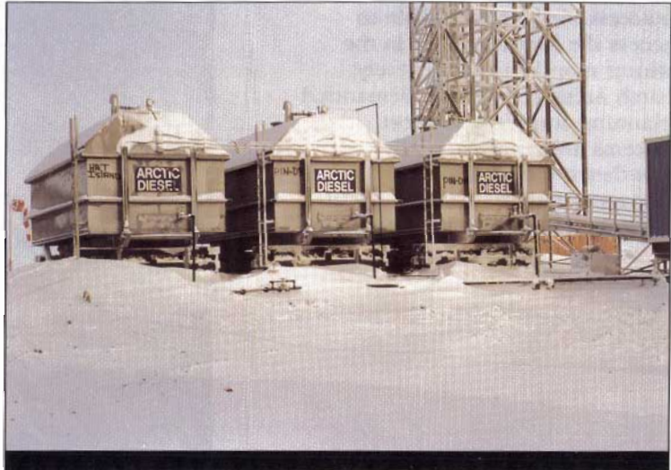
Fuel storage tanks at base of tower.
