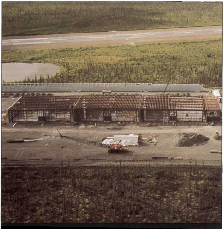
Aerial view of steel erection and construction of aircraft hangar bays.
