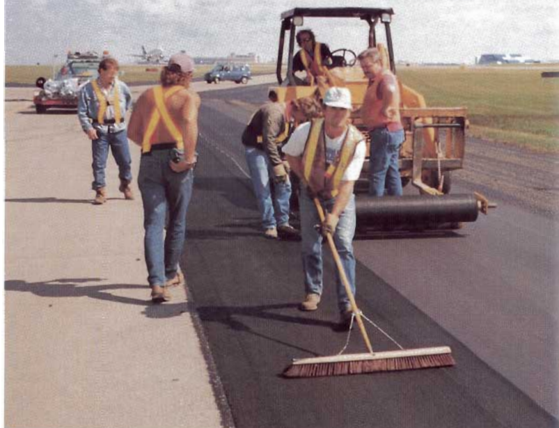
Asphalt overlay ▸
