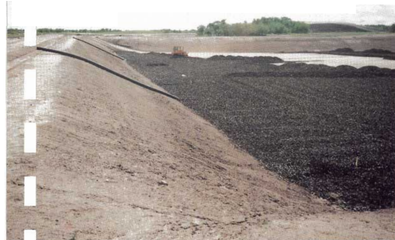
Innovative application of shredded tires for landfill drainage
