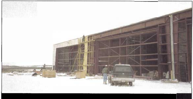
Cladding being installed on the hangar door steel framing.
