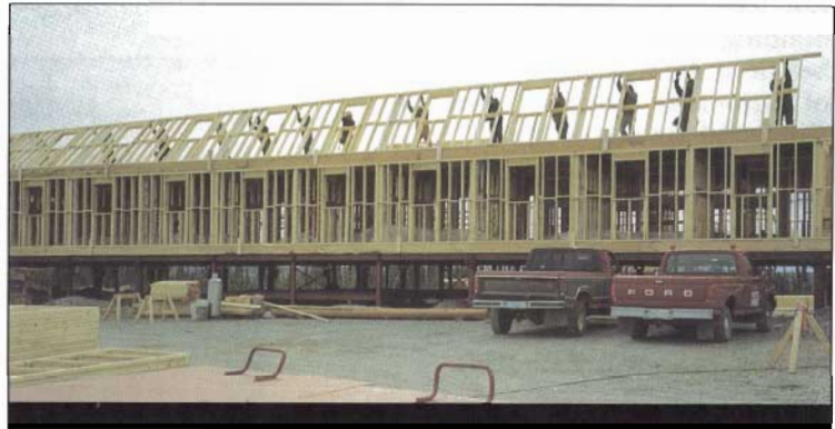
Raising a wall on the 102-room accommodation building.
