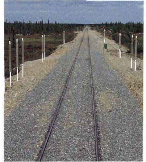
◇ Experimental railway sections using heat pipe installations to alleviate thaw settlement
