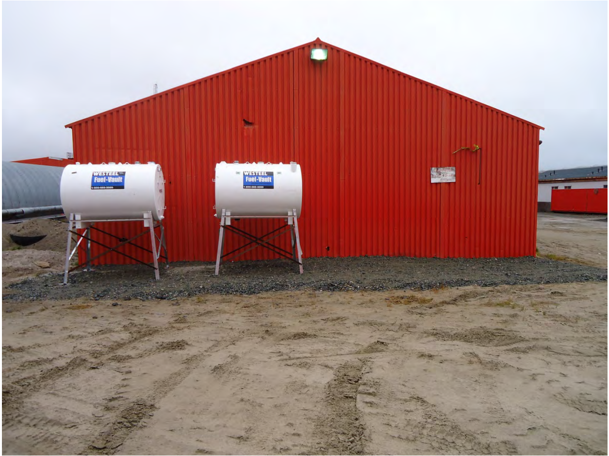
Photo 27: IND-6 new double wall tanks at Camp Generator 2012.
