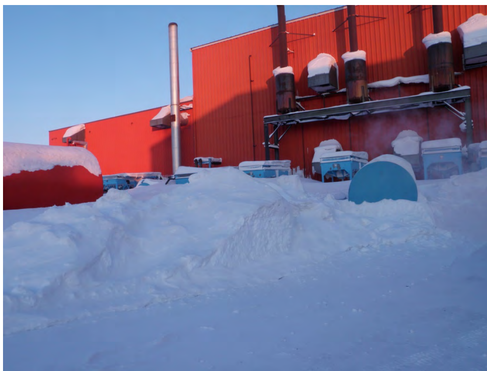
Photo 12: Blue Glycol Tank (GLY-2 in foreground, now in Boneyard) and Radiators, Feb 2012.
