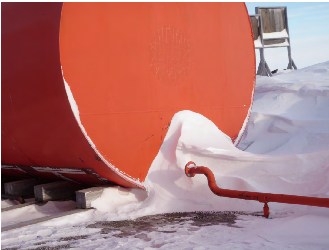
Photo 5: M-22 Disconnected From Piping, Feb 2012.
