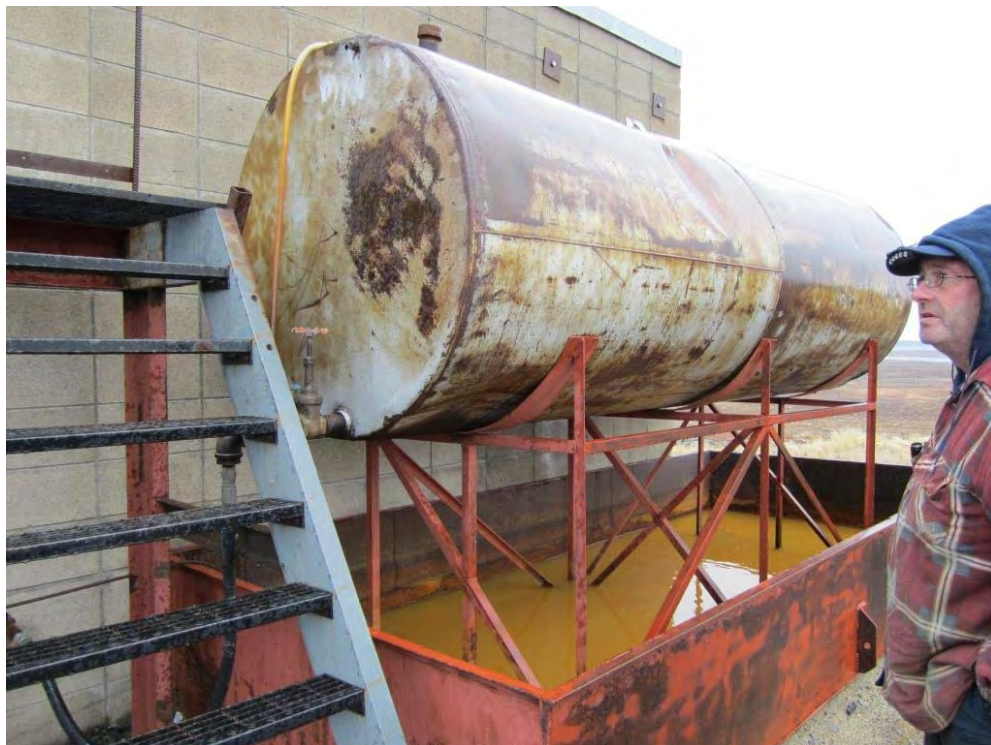
Photo 17: Incinerator Tank, IND-8. Replaced with a double wall tank 2012.
