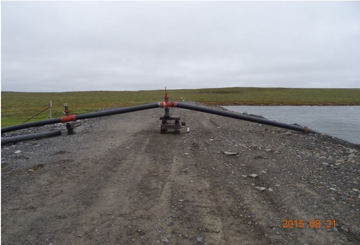
Figure 2 Berm wall - lower sewage lake with syphons installed
