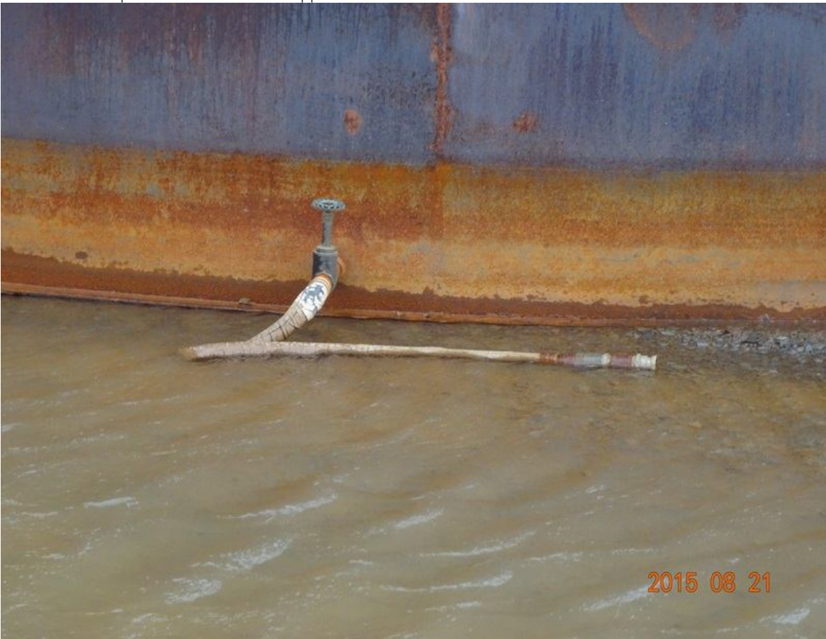
Figure 9 Hose attached to 5 million litre tank within the bulk fuel containment area
