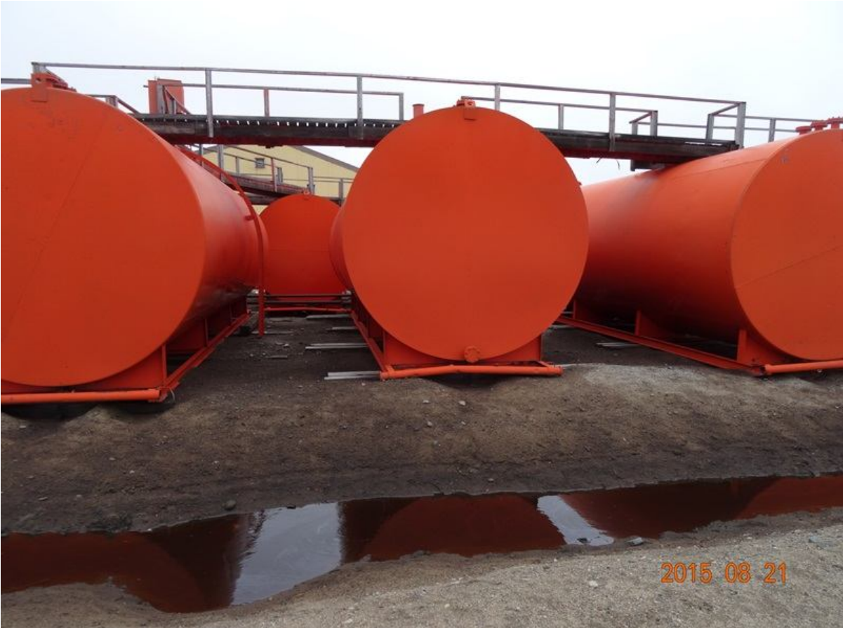
Figure 14 Satalitte tank farm - surface staining
