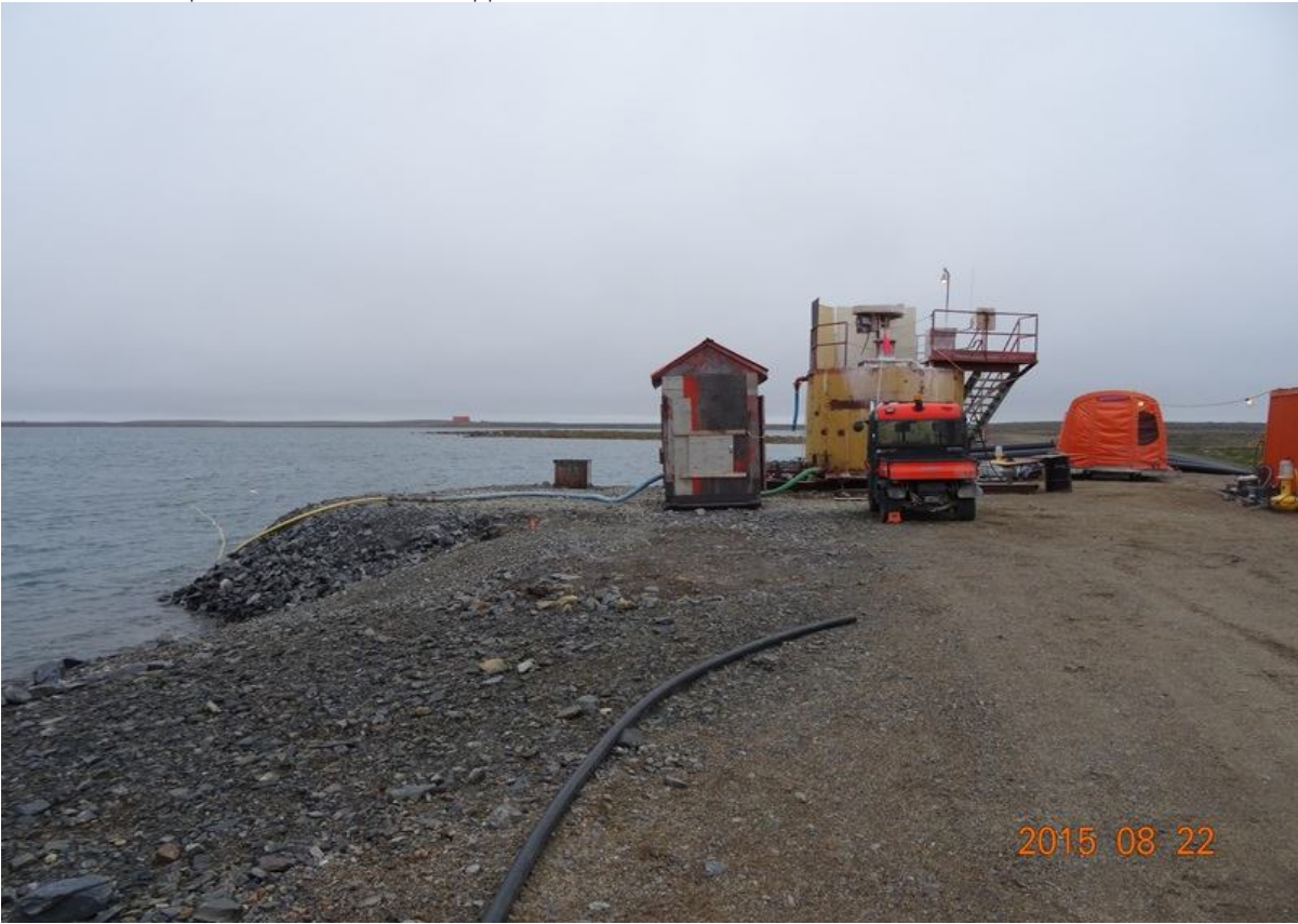
Figure 19 Contact water from within the tailings containment area - Lye mixing station on berm wall
