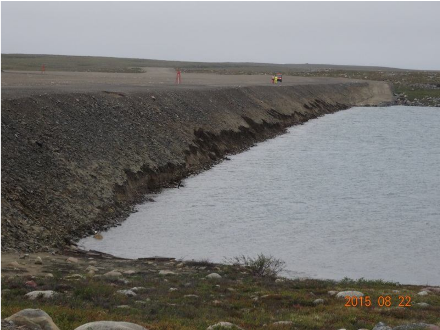
Figure 22 Water / surf scour and erosion of berm walls within the TCA.
