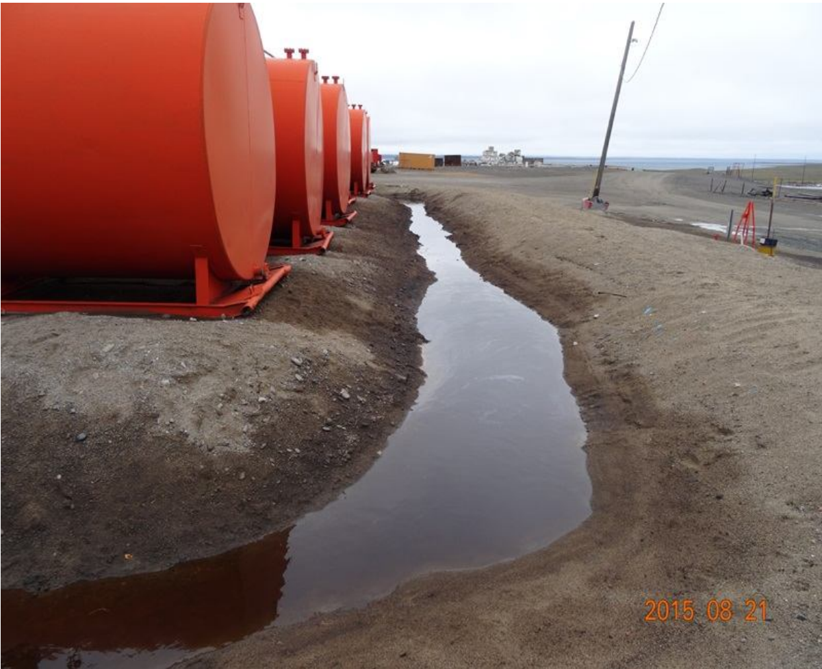
Figure 12 Satellite tank farm - free product and staining from previous spills
