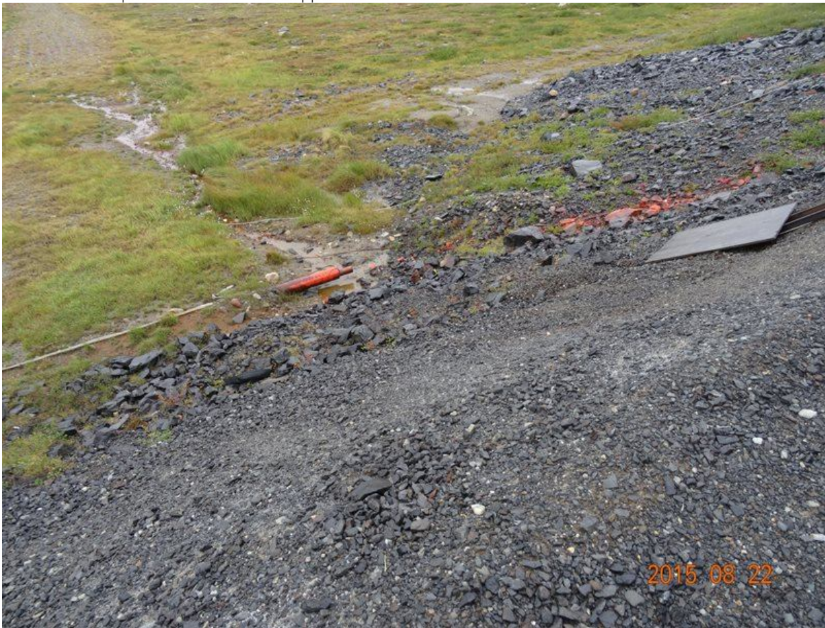
Figure 15 Drainage and flow from back side of Bulk Fuel storage tank farm berm
