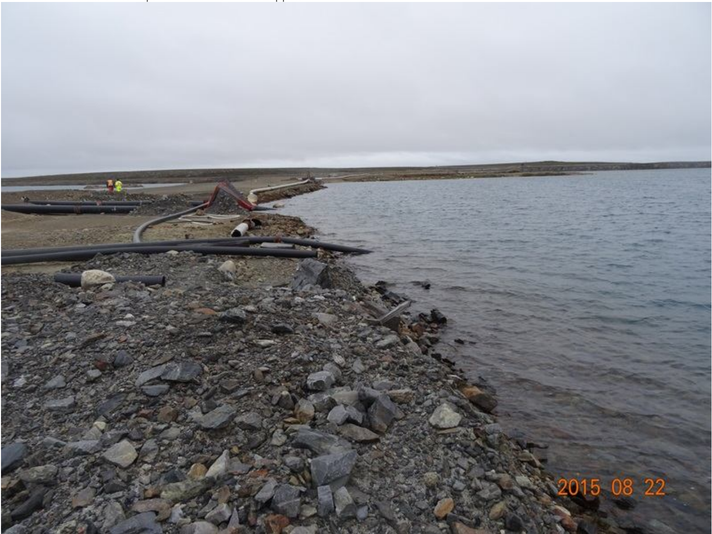
Figure 23 Berm wall less than 1 meter of free board as required by License
